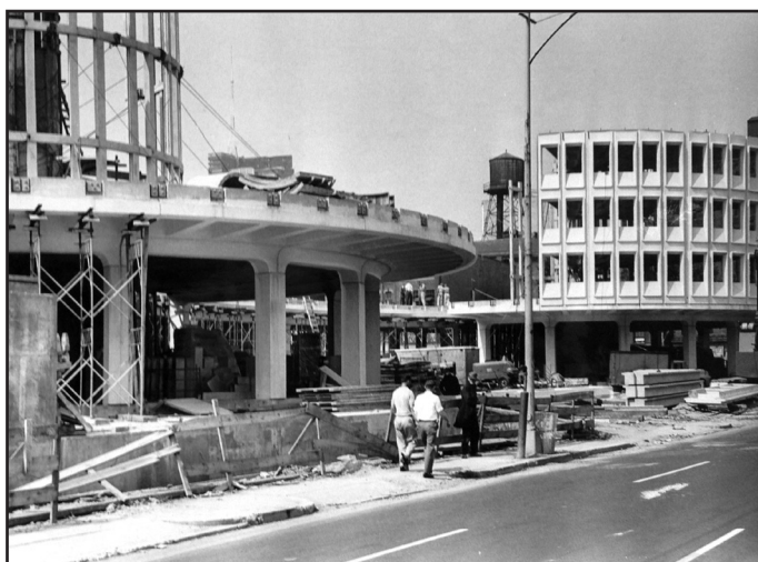
Figure 9: Circa 1960 photograph of the construction of the Philadelphia Police Headquarters. (Source: Urban Archives, Temple University)
