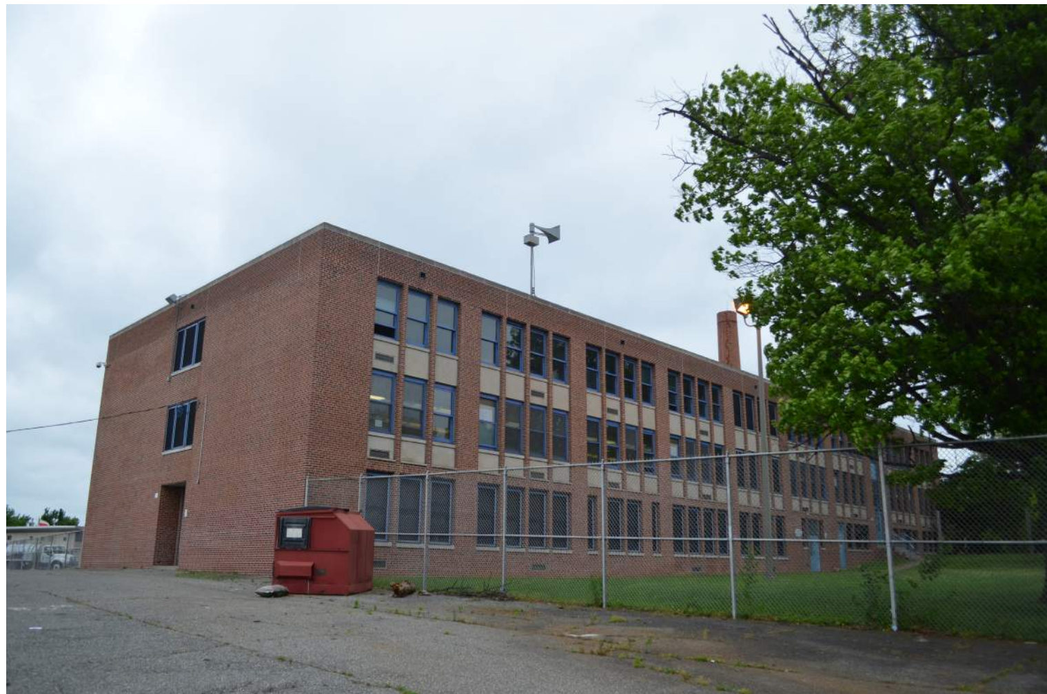
Site Photo A
