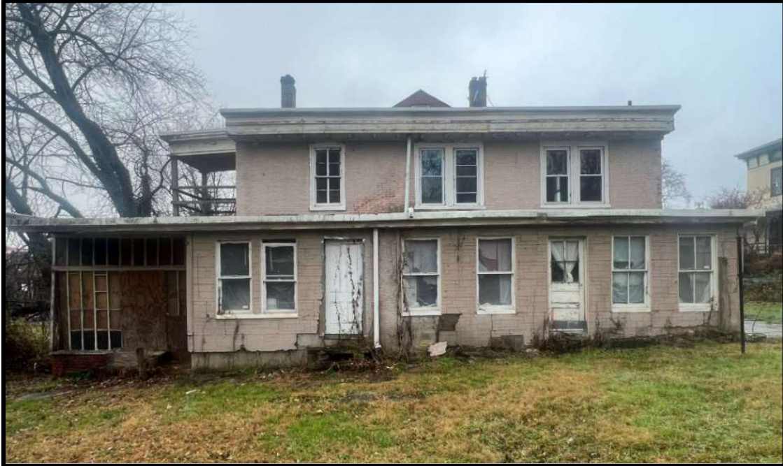
Figure 12. The Smith-Steel-Humphreys House, 424 E. Woodlawn Street, Rear (Southeast) Elevation of the Rear Brick and Rear Frame Additions. Source: Oscar Beisert, 2023.
