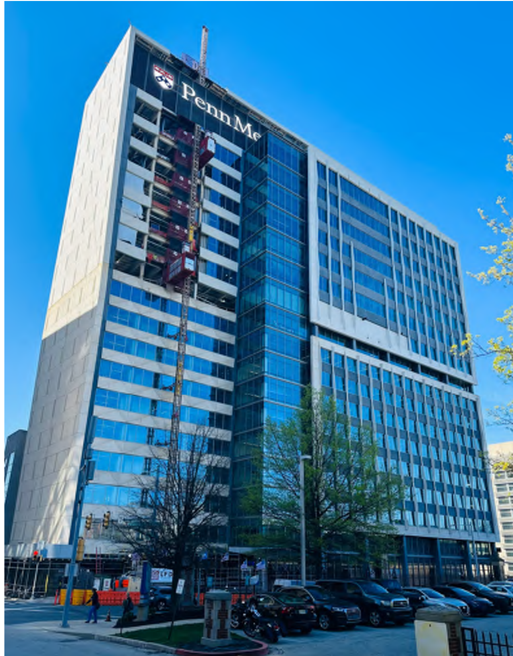
North Elevation View from Civic Center Boulevard, building NE
