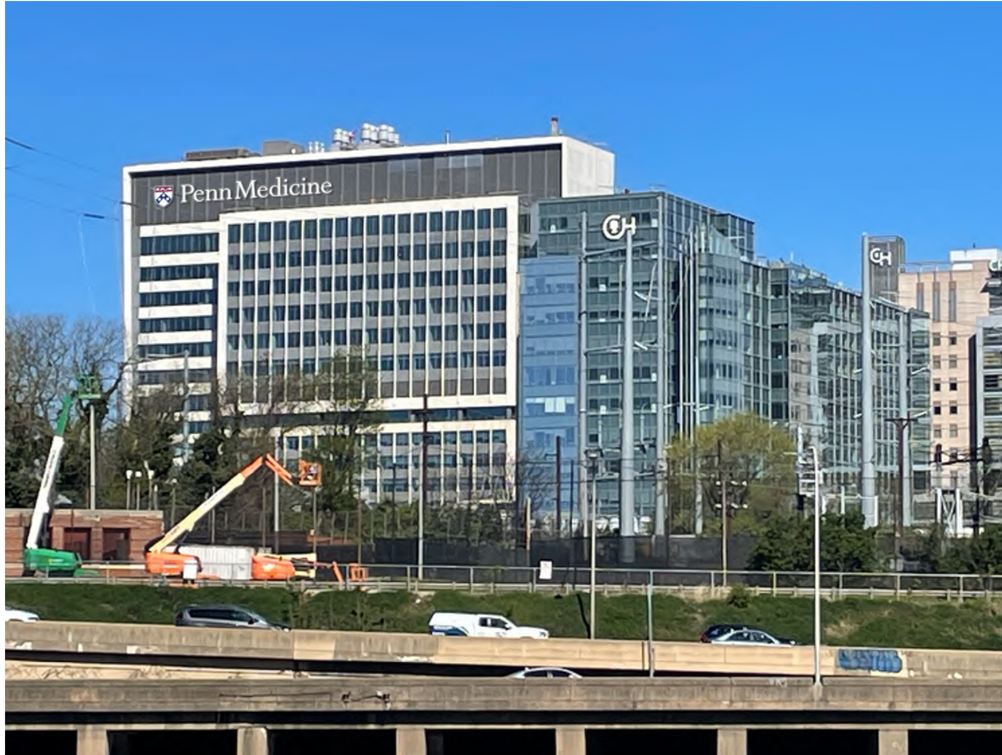
South Elevation View from south of Schuylkill River
