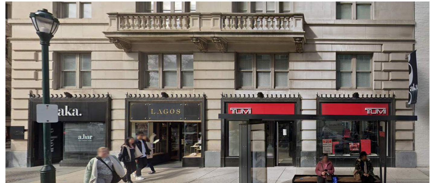
Composite Street View along Walnut Street
