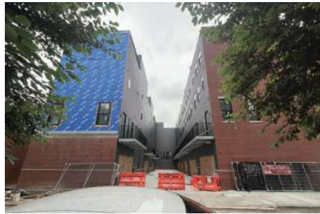
2 REAR VIEW OF 244-58 N. 2ND STREET
