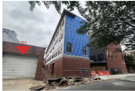
3 REAR VIEW OF 244-58 N. 2ND STREET
