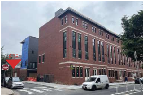
1 FRONT VIEW OF 244-58 N. 2ND STREET
