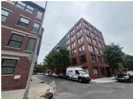
11 FRONT/SIDE VIEW OF 211 VINE STREET
