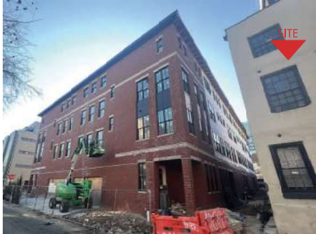
4 FRONT VIEW OF 244-58 N. 2ND STREET
