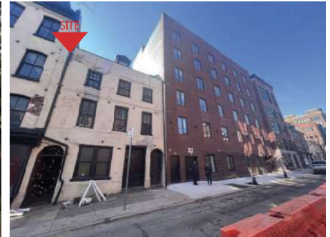
10 FRONT VIEW OF 214 VINE STREET
