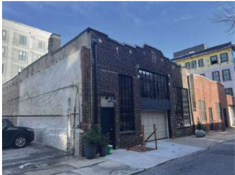
7 FRONT VIEW OF 213-15 NEW STREET
