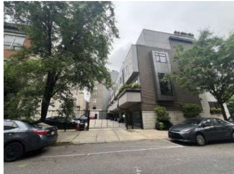
8 REAR VIEW OF 300-10 N. 2ND STREET
