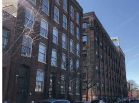
6 VIEW OF 214-18 NEW STREET
