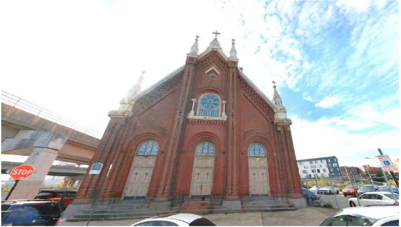
Figure 1: View the north elevation, October 2023
