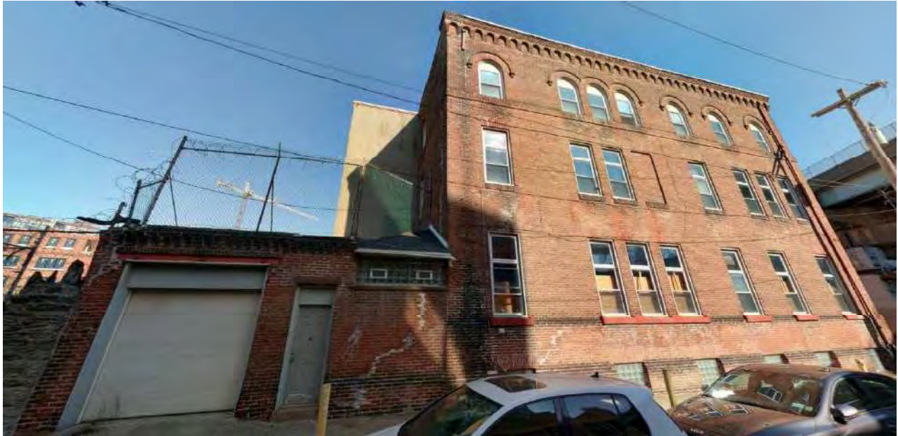
Figure 5: View of south elevation of Rectory, October 2023
