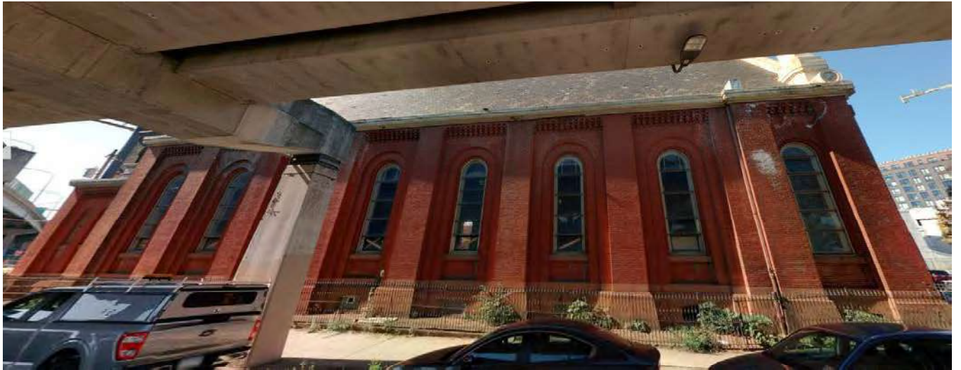
Figure 3: View the west elevation, October 2023
