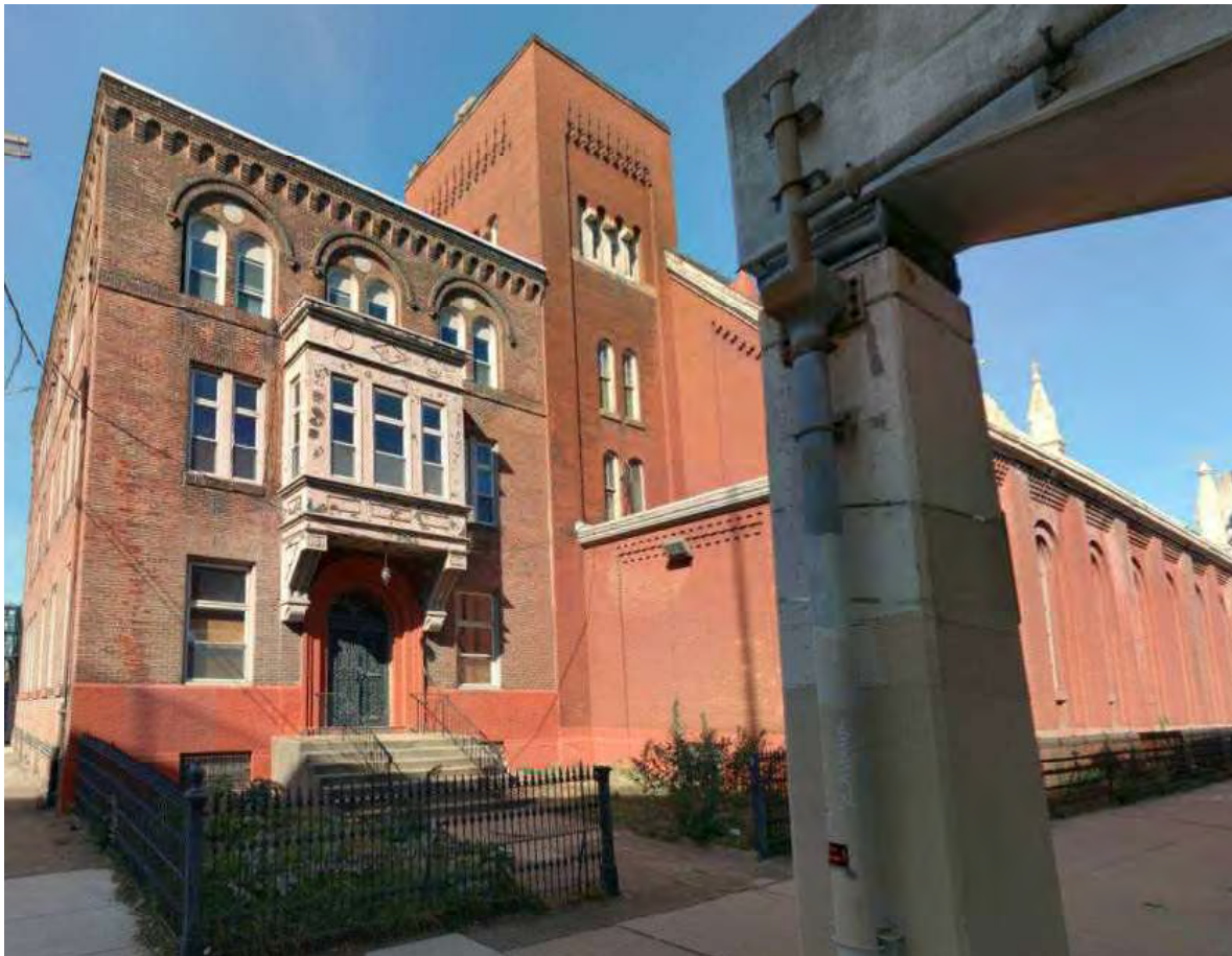
Figure 4: View east elevation of Rectory, October 2023
