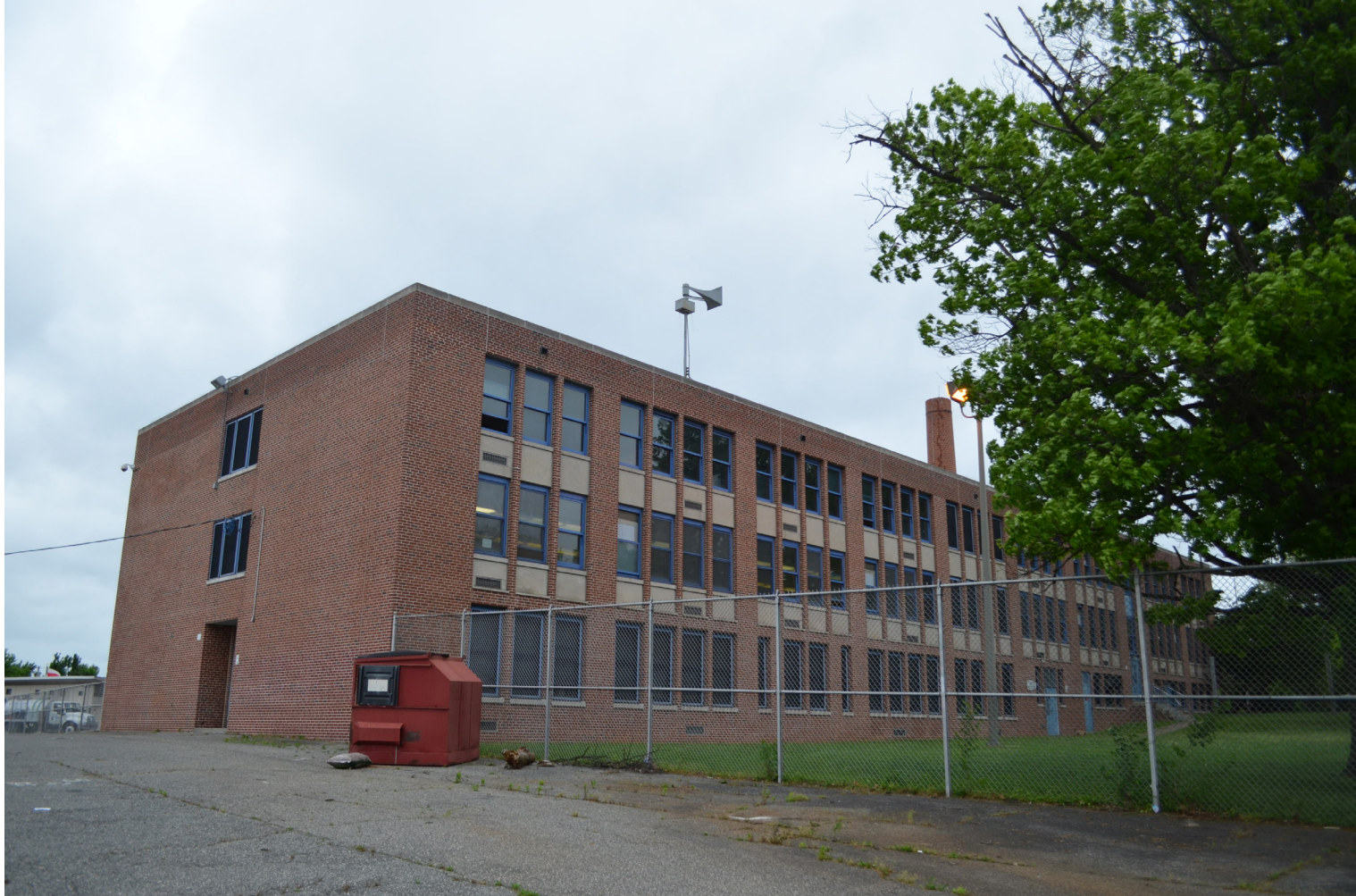
Site Photo A
