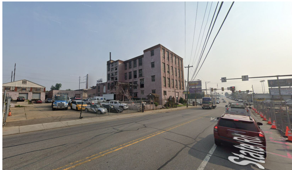
3_SITE VIEW FROM STATE RD.
