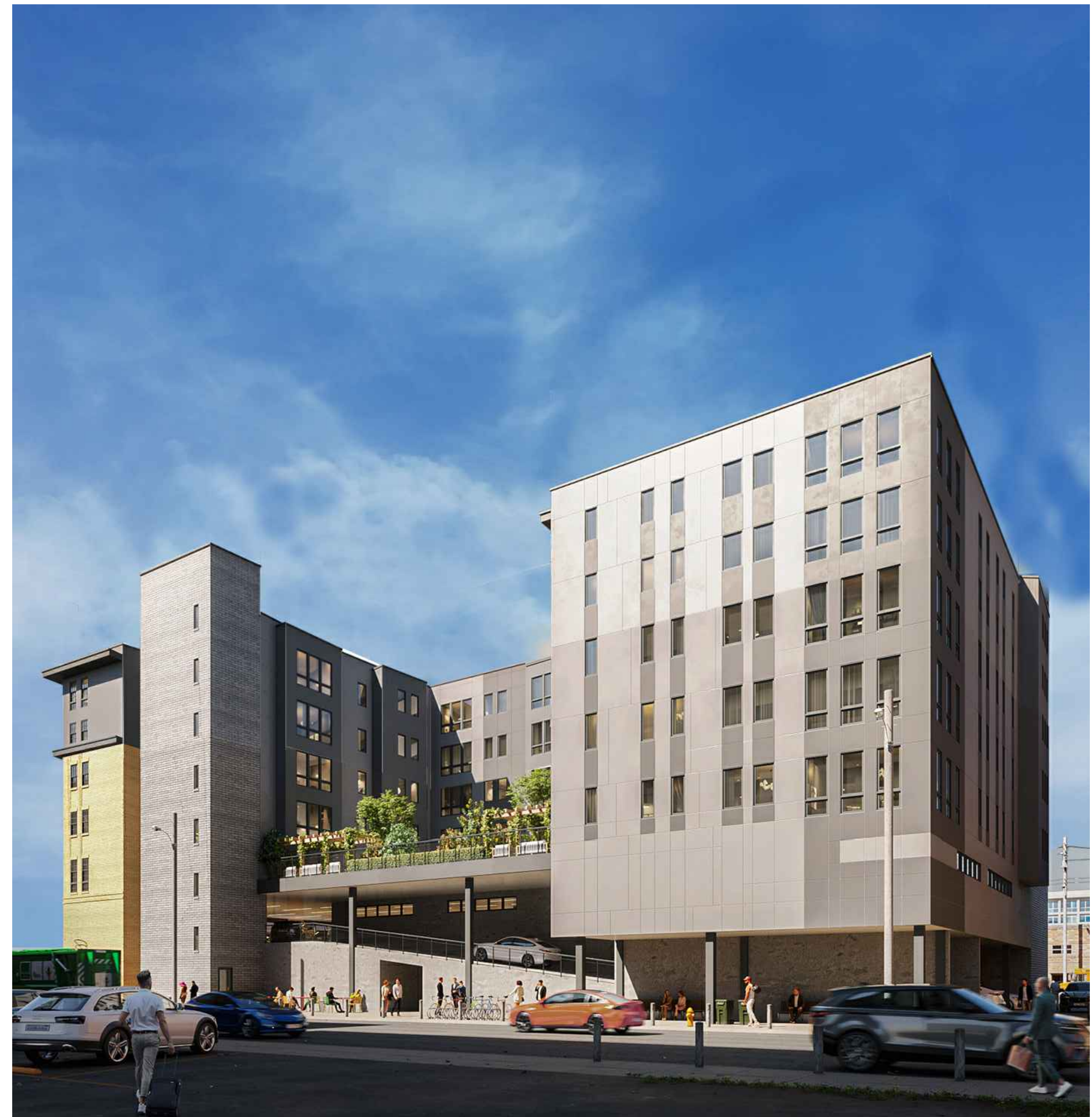
2 View Looking North
