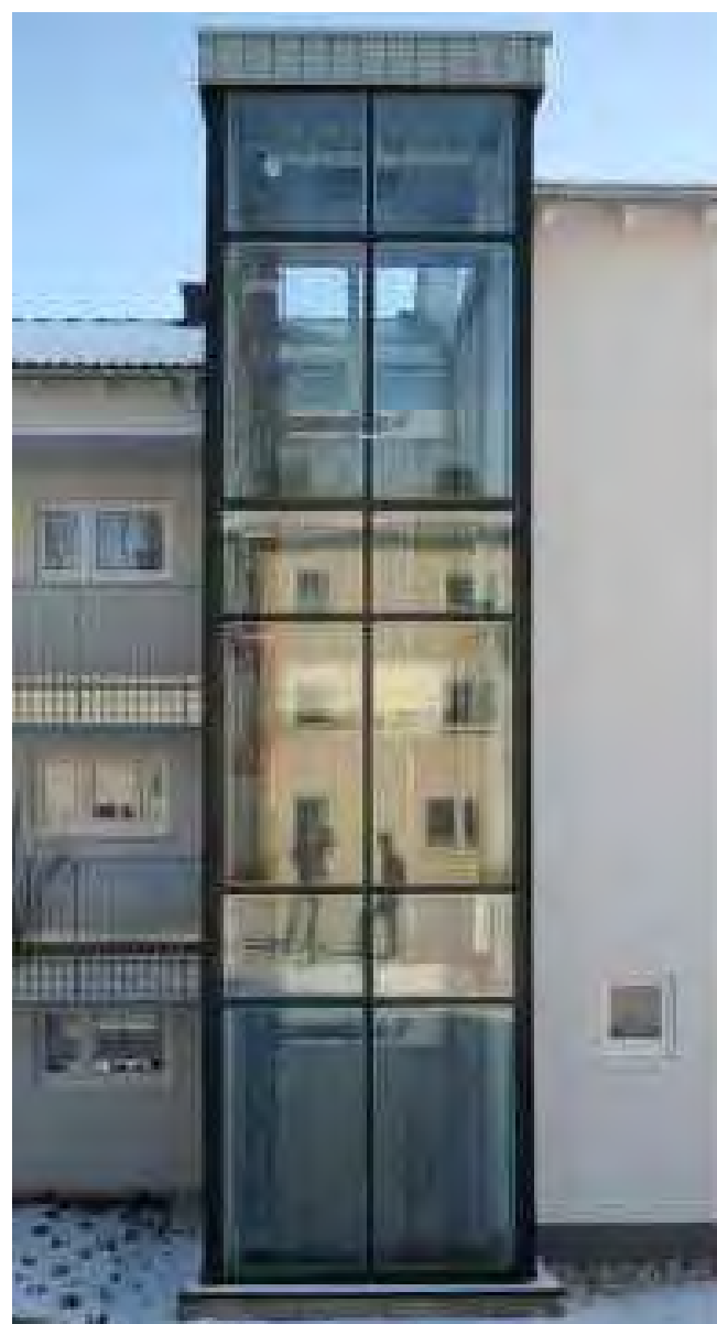
Glass Curtain Wall
