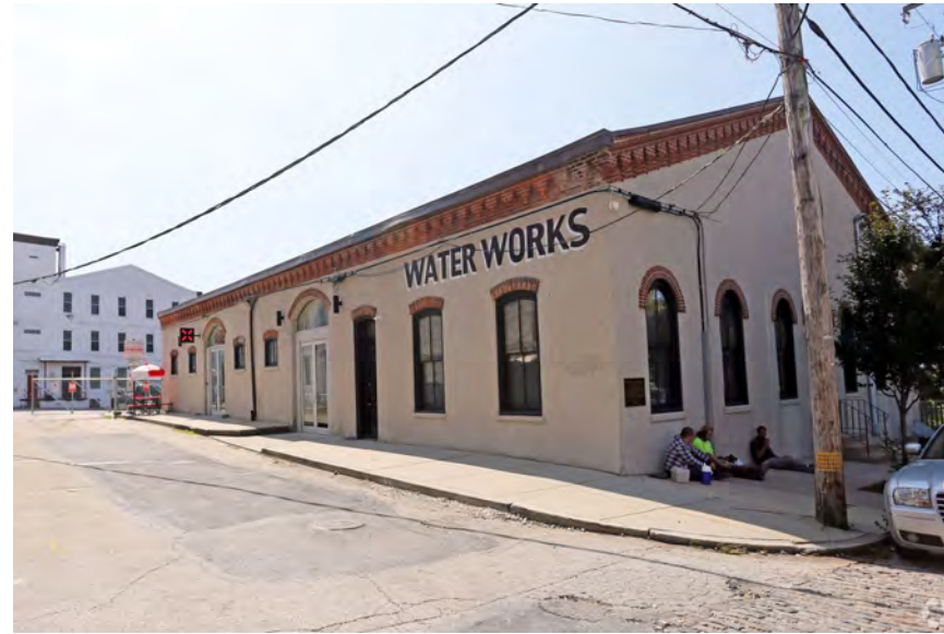
Water Works - Manayunk
