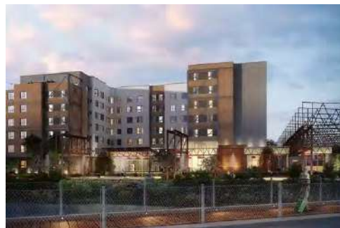
Residence Inn by Marriott 615 Righters Ferry Road, Bala Cynwyd 7 Stories - 124 Suites
