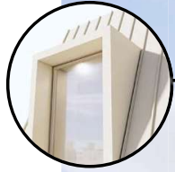
ALUMINUM WRAP DORMER MATCHED TO ROOF
