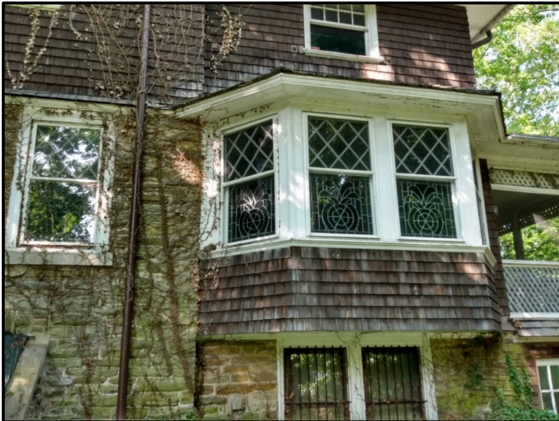
Figure 11: The large bay window on the east wall of the house, showing the leaded glass patterns.
