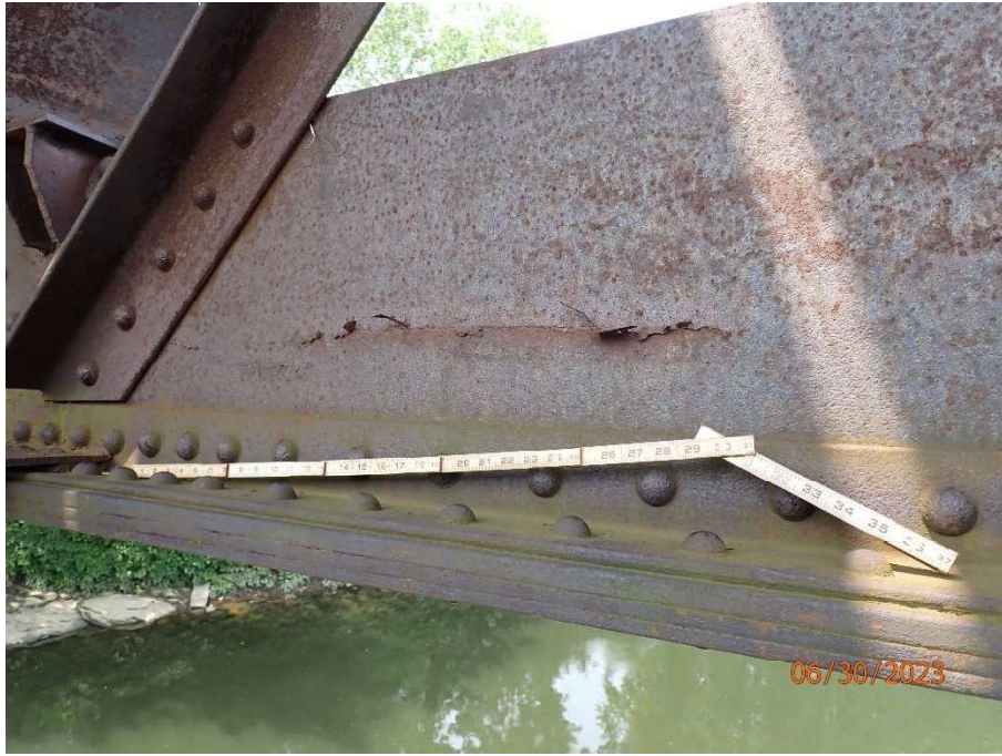
Girder 1, Span 5, looking southwest. 30" long steel defect in the bottom web plate.
