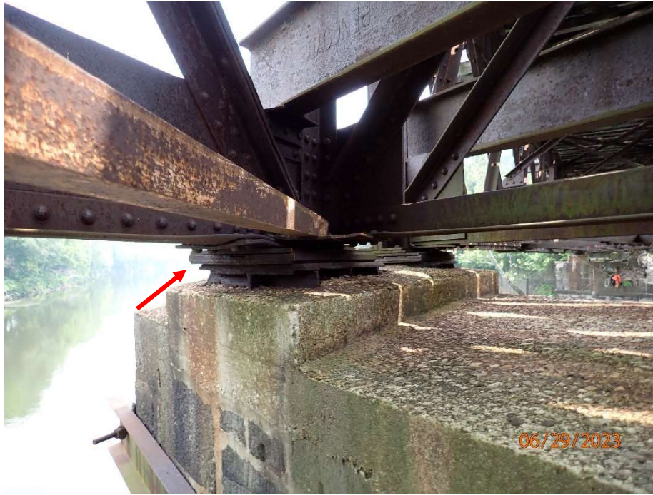
Girder 1 bearing at Pier 5, looking southeast. Bent top bearing plate.
