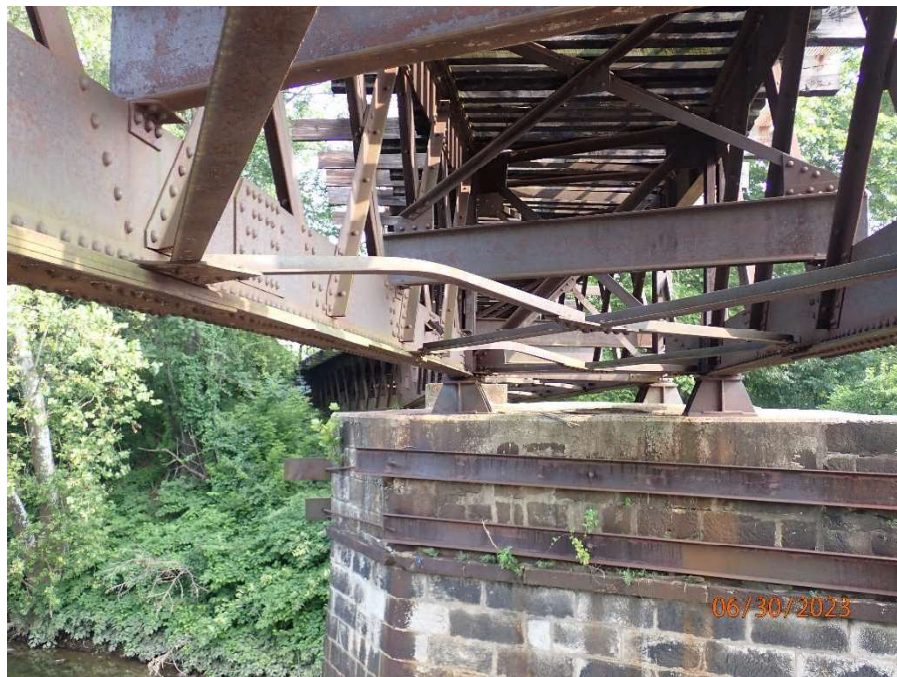
Girder 1, Span 6, looking north. Lower cross bracing is bent due to flood impact damage.
