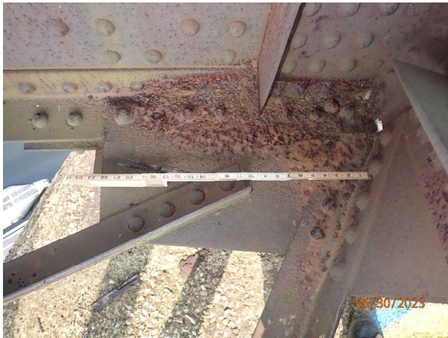
Span 5, Girder 1 bearing at Pier 6, looking west. Cracked connection to top bearing plate. Severe pitting to angles with up to 100% section loss to the rivet heads.
