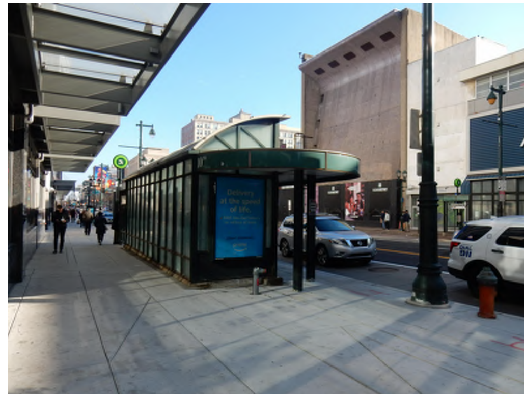
EXISTING NORTH HEADHOUSE - LOOKING EAST
