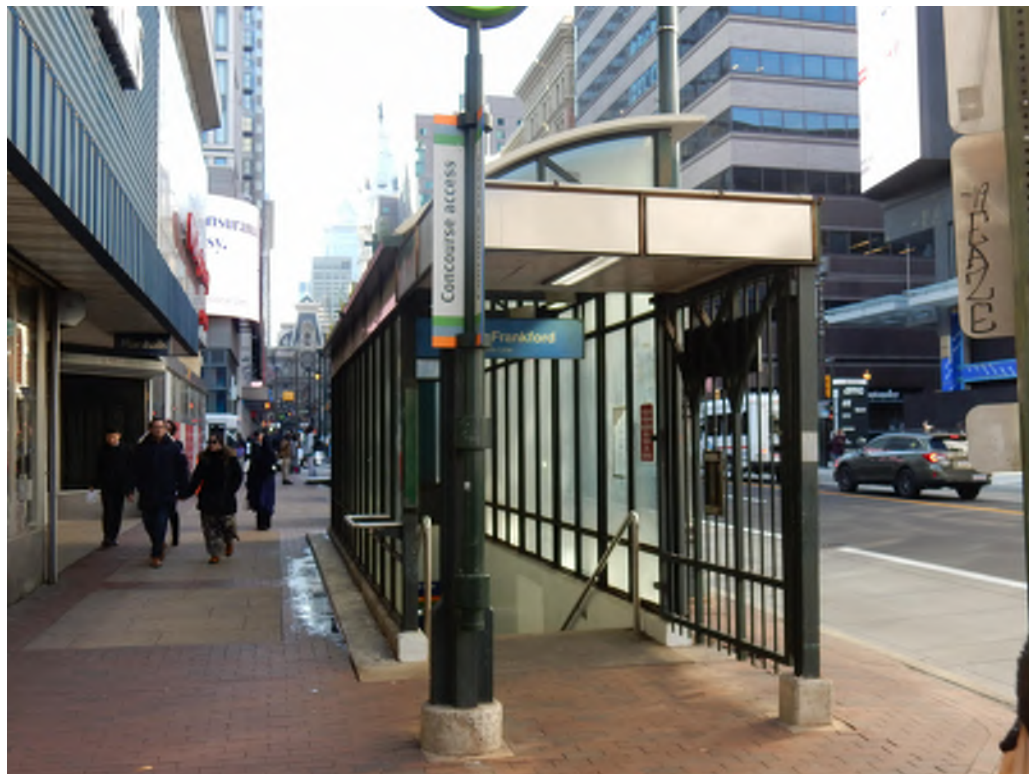
EXISTING SOUTH HEADHOUSE - LOOKING WEST
