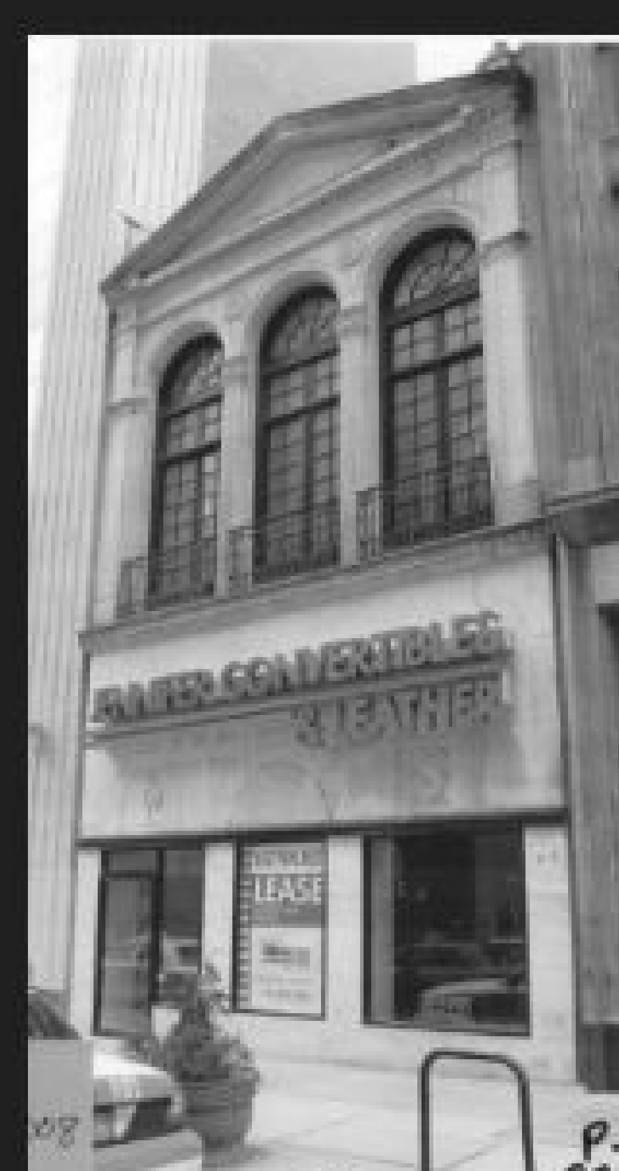
PREVIOUS TENANT FACADE RENOVATION
