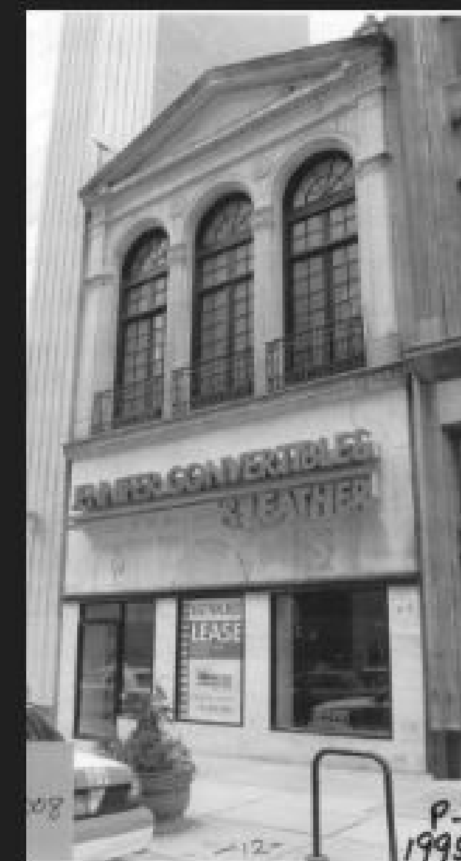
PREVIOUS TENANT FACADE RENOVATION
