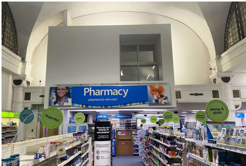
Figure 5a – South end of the Main Sales floor, looking south to the original mezzanine level, under which the pharmacy was located. The concrete frieze located behind the blue pharmacy sign is the lower edge of the mezzanine that was installed in 1913. The original inlaid Mercer tile details also remain, although the original iron mezzanine railing and the central stair leading up to the mezzanine were removed in recent decades.
