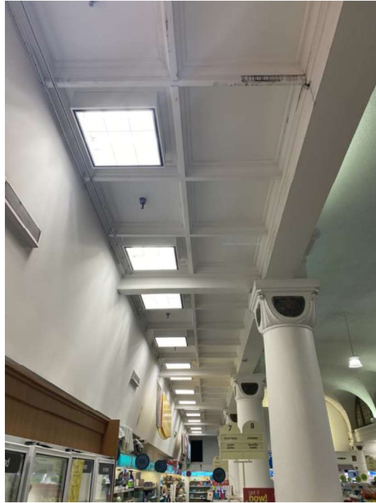
Figure 16 – Typical side aisle skylights (October 2021). At far left, a drywall bulkhead conceals a third row of skylight panels, a condition which is mirrored on the opposite side of the space.
