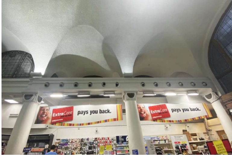
Figure 8 – View of west wall, columns 1-3 (right to left) showing the location of Murals 1 and 2.
