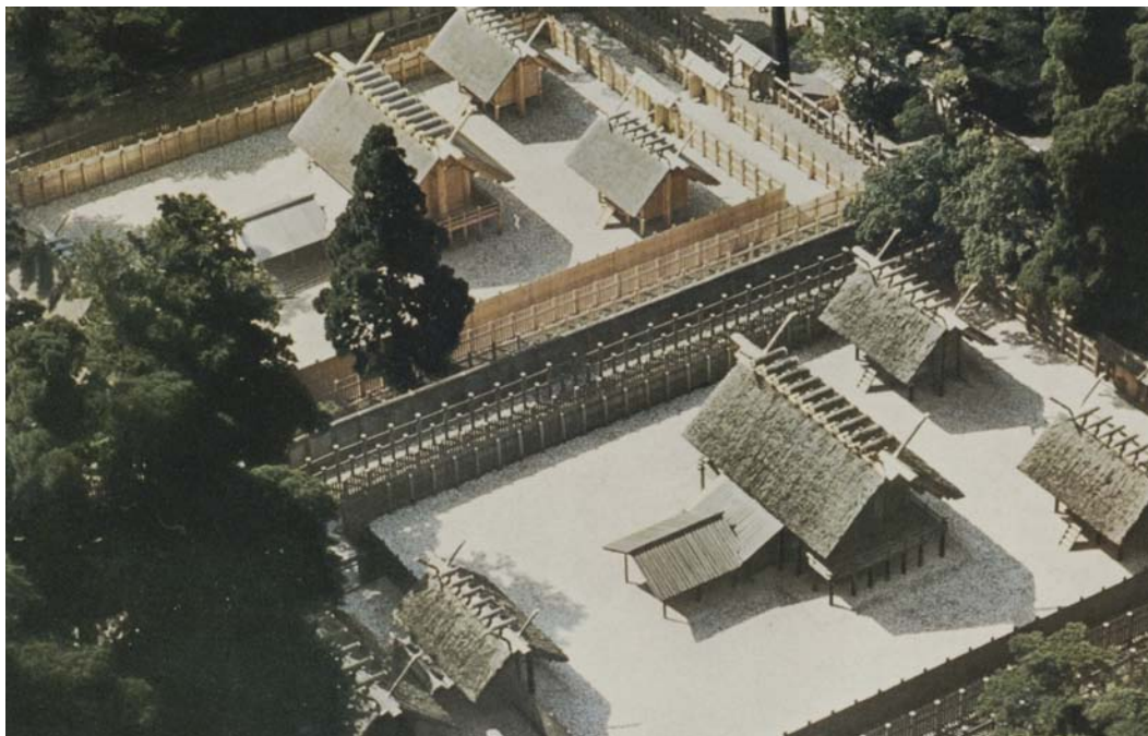
Ise Grand Shrine — Ise; Shinto Shrine, Aerial View showing layers of boundary fencing
