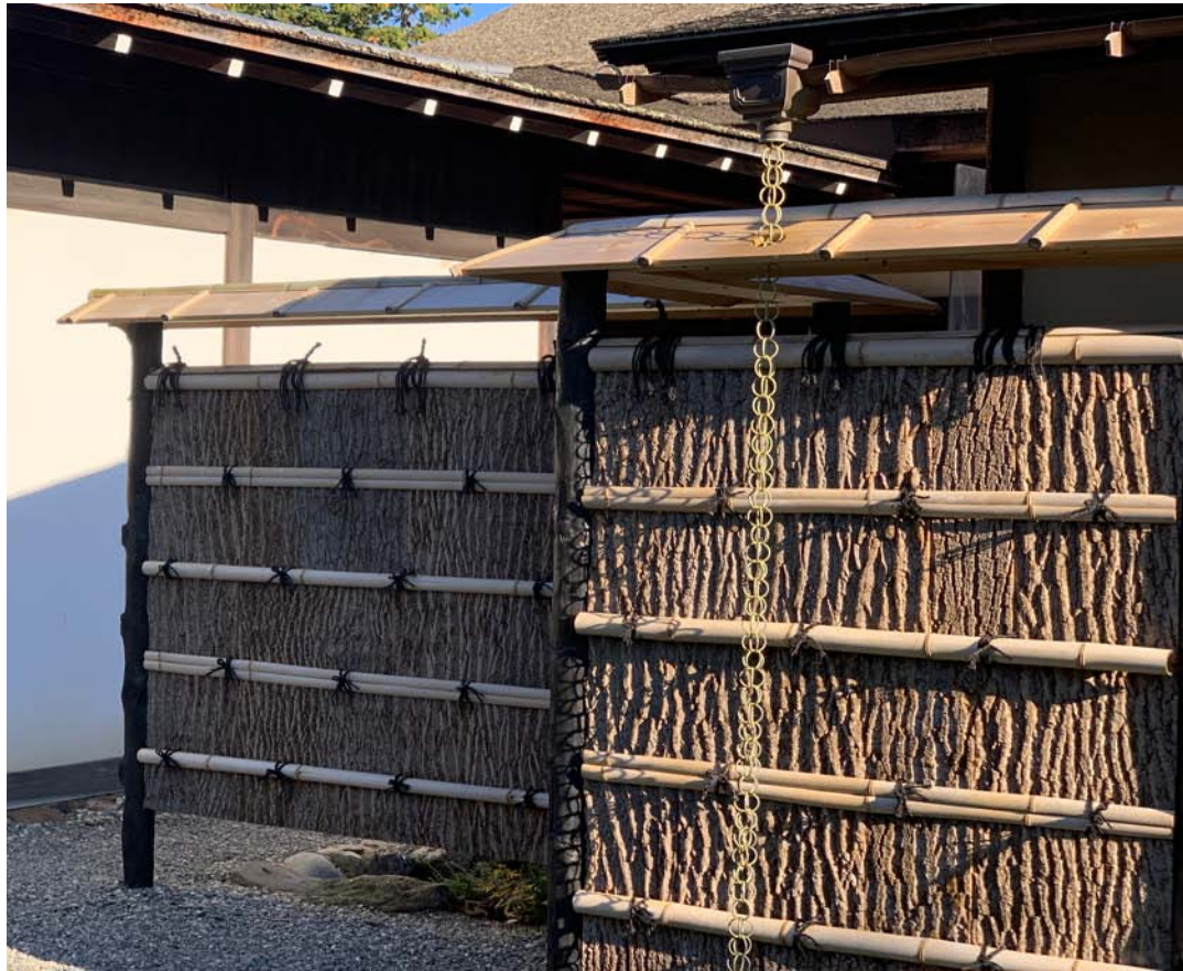
Shofuso Courtyard : Traditional Bark Fence using Local Tulip Poplar Bark & Cedar Wood
