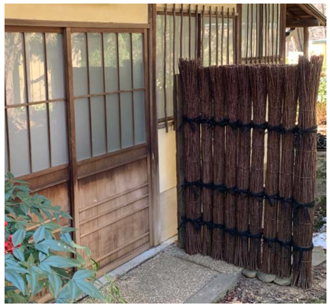
Embassy of Japan; Washington DC: Traditional Taimatsu-gaki Using Local Willow
