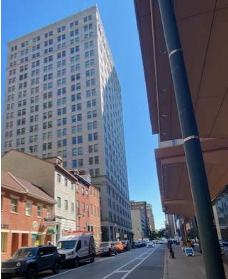
Figure 3. Spruce Street east of proposed building.
