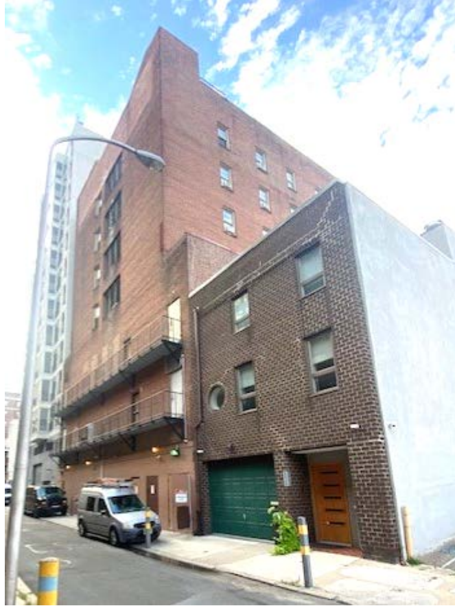
Figure 3. Ranstead Street immediately east of proposed building.
