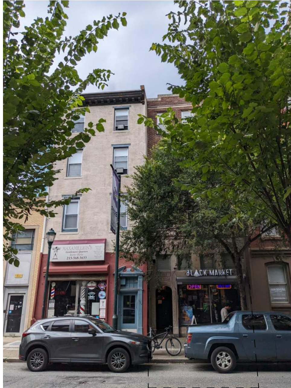
EXISTING BUILDING AT 2033 CHESTNUT STREET
