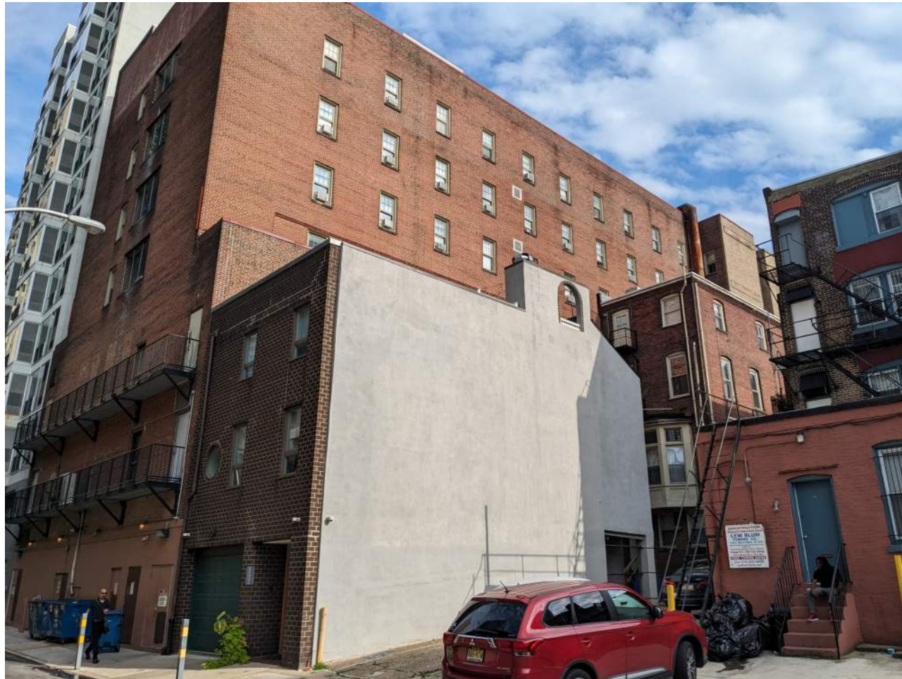
RANSTEAD STREET LOOKING SOUTHEAST THROUGH SITE
