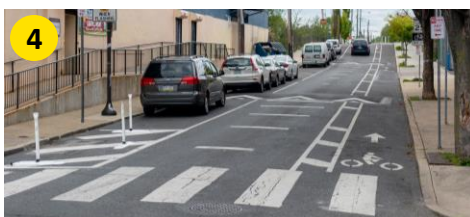
4. Speed cushions and corner clearance in Fairhill
