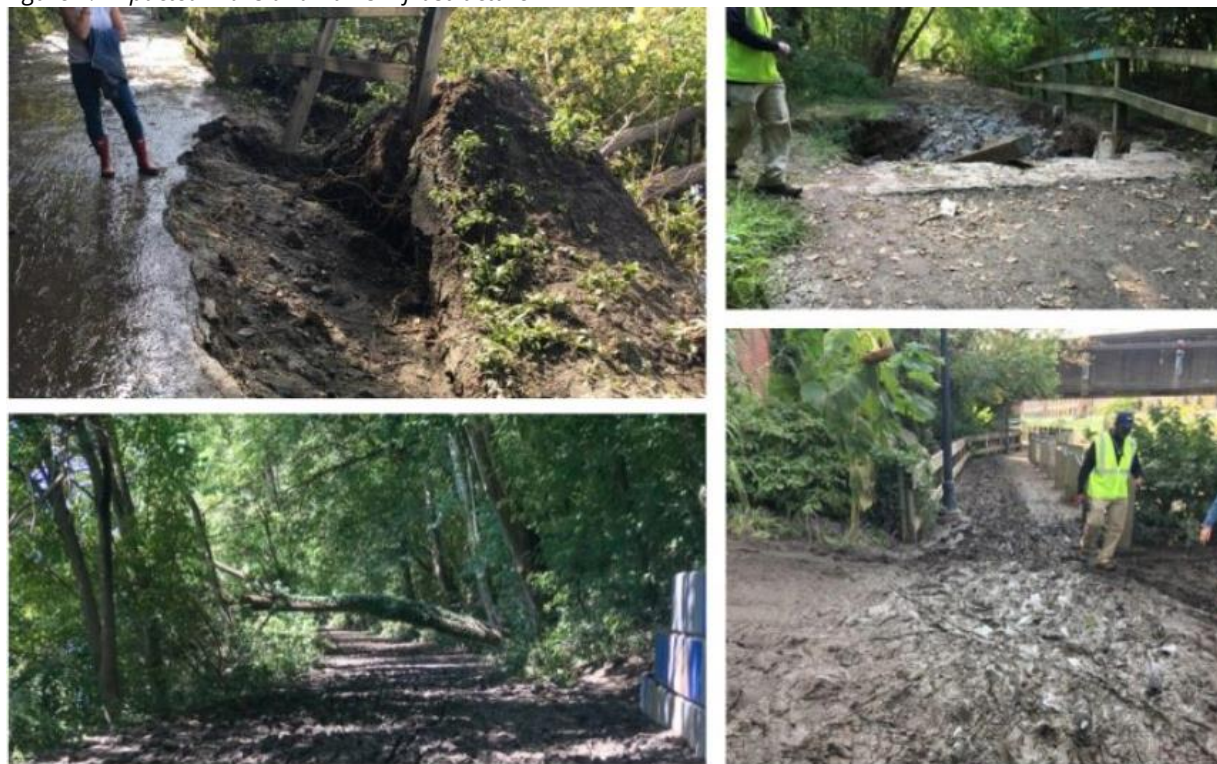
Figure 4: Impacted Trails and Parks Infrastructure
