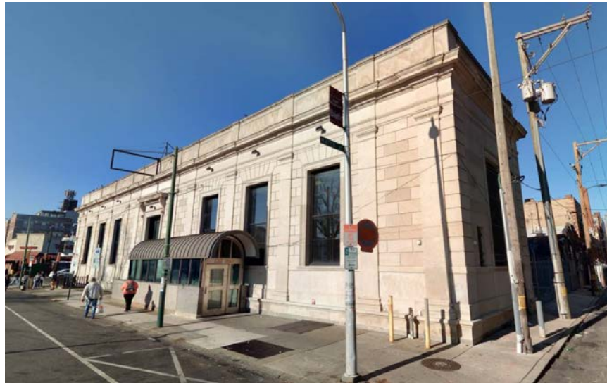
Figure 4: South elevation, looking northwest from Snyder Avenue.
