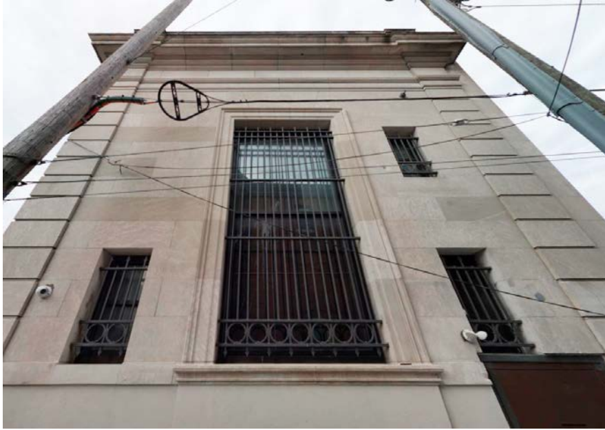
Figure 5: East elevation, looking west from Watts Street.
