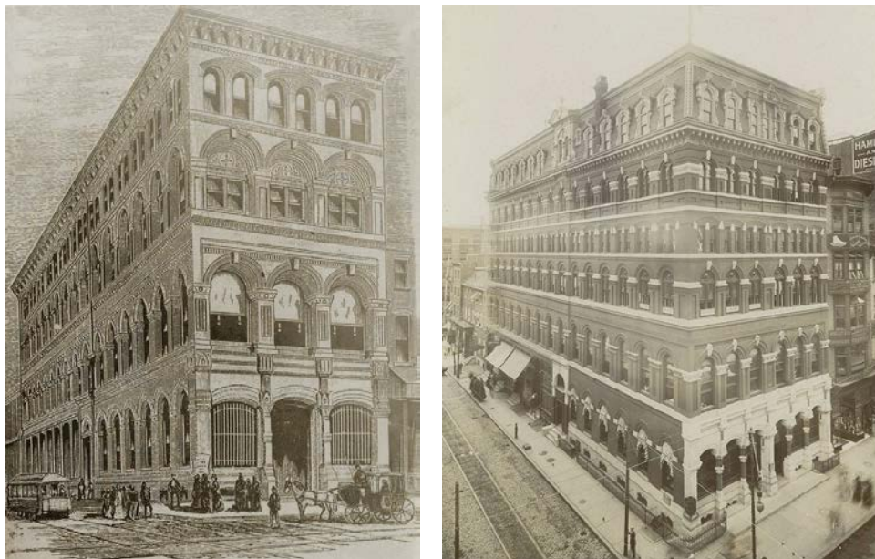
Figure 1 - The Beneficial Saving Fund Society building as it appeared in 1880, and after the 1887 additions and alterations (Free Library of Philadelphia).
