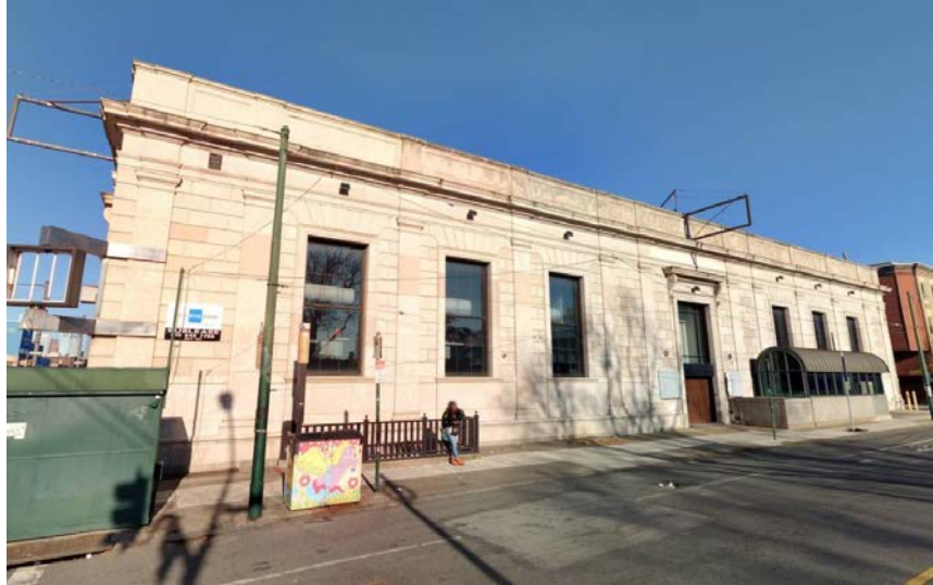
Figure 3: South elevation, looking northeast from Snyder Avenue.
