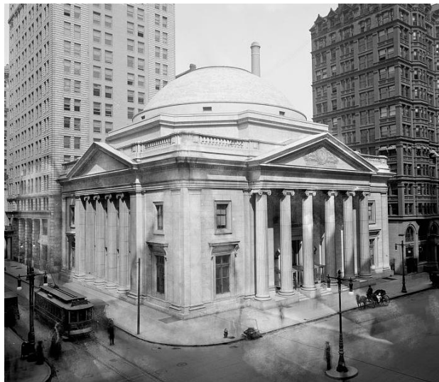
Figure 9 - The Girard Trust Company at Broad and Chestnut Streets, designed by Furness & Evans with McKim, Mead & White and built in 1907 (Library of Congress). Extant.
