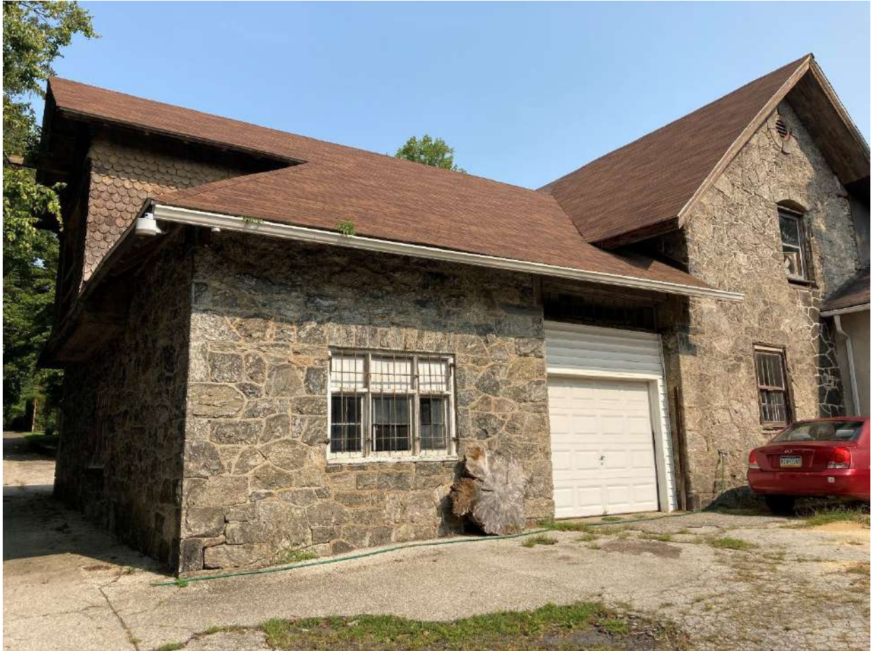
Figure 17: September 2022 photograph showing current conditions of the carriage house. View looking northeast.
