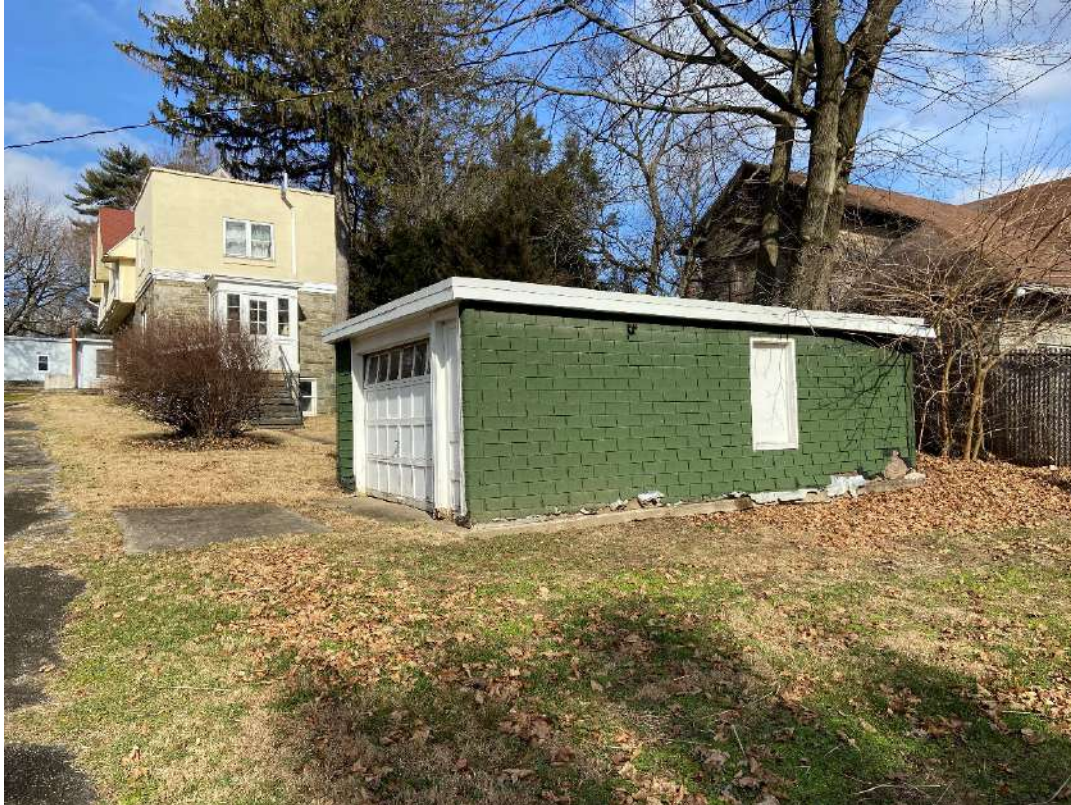
Site visit photograph, Ancillary Building
