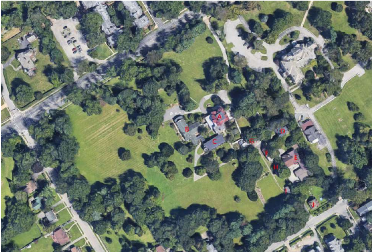
Figure 41: Aerial image illustrating individual buildings within the Property. Only buildings A, B, and J are visible from public rights-of-way.
