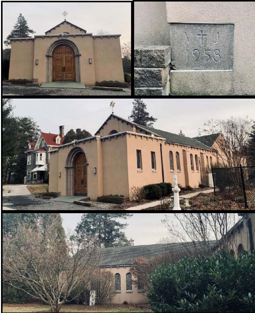
Figure 58. Left: The primary (northwest) elevation of 1e. Chapel Addition. Figure 59. Right: The “1958” cornerstone within primary (northwest) elevation of the 1e. Chapel Addition. Source: Oscar Beisert, 2019. Figure 60. Middle: The primary (northwest) and side (southwest) elevations of the 1e. Figure 61. Bottom: A side component of the primary (northwest) elevation of the 1e. Source: Oscar Beisert, 2019.
