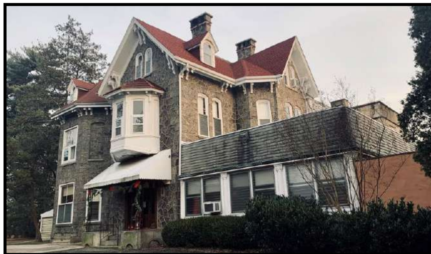
Figure 46. The primary (northwest) and side (southwest) elevations of the Main Block and the Porch Addition. Source: Oscar Beisert, 2019.
