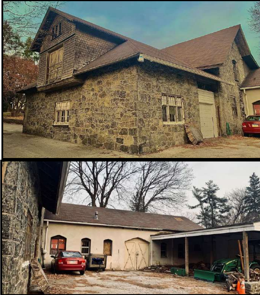
Figure 72. Top: The southwest and southeast elevations of the Carriage House & Stable. Figure 73. Bottom: The southwest elevation of the Stable component of the Carriage House & Stable. Source: Oscar Beisert, 2019.
