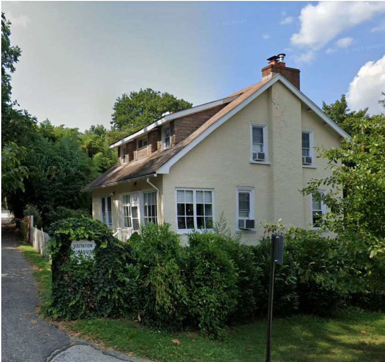
Figure 24: August 2021 image, showing the cottage at the south end of the subject property. View looking north from Overbrook Ave.
