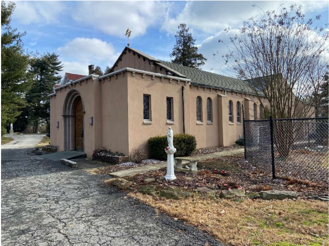
Site visit photograph, Chapel looking from the parking lot to the southeast
