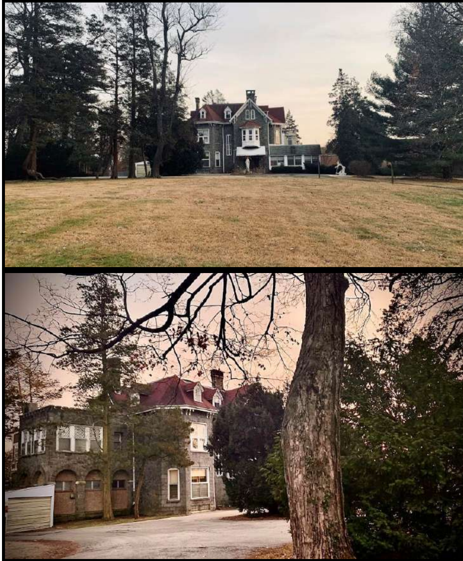
Figure 44. Top: The primary (northwest) elevation of the Main Block. Figure 45. Bottom: The northwest and northeast elevations of the Main Block from the driveway. Source: Oscar Beisert, 2019.
