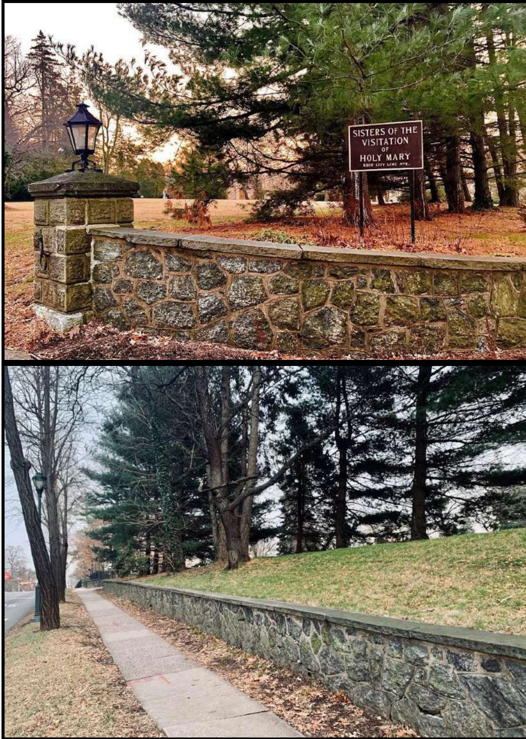
Figure 19. Top: Looking south at the stone curbing and wall at the North Driveway and along City Avenue at the northwest property line of the subject property. Figure 20. Bottom: Looking northeast at the stone wall and curbing along City Avenue at the northwest property line of the subject property. Source: Oscar Beisert, 2019.
