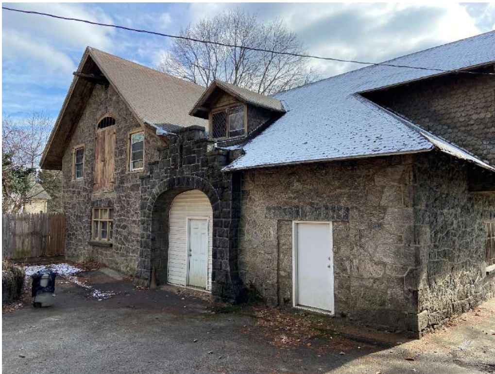
Site visit photograph, front of carriage house.
