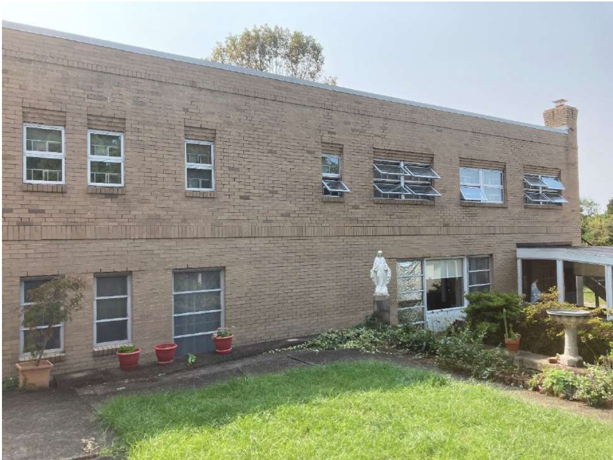
Figure 15: September 2022 photograph showing the dormitory addition to the mansion house. The dormitory addition is a visual intrusion when compared with the remainder of the main house. The addition eliminated the historic bucolic viewshed from the main house. View looking south.
