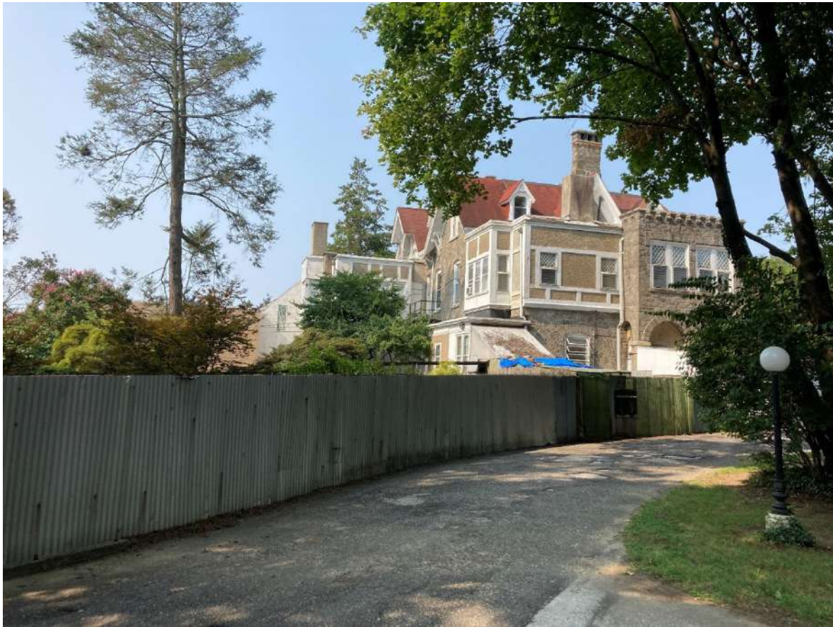
Figure 13: September 2022 photograph showing the south addition, which is located to the south of the arcade addition. View looking northwest.
