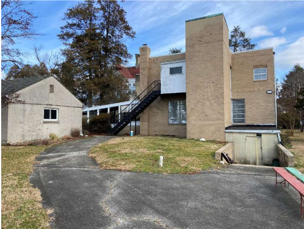
Site visit photograph, rears of the Chapel and Dormitory looking to the east
