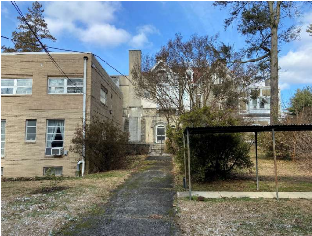
Site visit photograph, rear of main house with dormitory to the left and covered walkway to the right.
