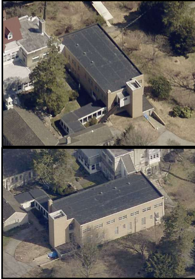
Figure 62. Top: The northwest and southwest elevations of the 1f. Dormitory. Figure 63. Bottom: The southwest and southeast elevations of the 1f. Dormitory. Source: Oscar Beisert, 2019.
