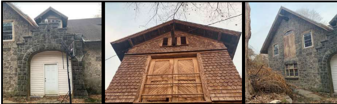
Figure 69. Left: A alteration to the central vehicle entrance of the primary (northwest) elevation of the Carriage House & Stable. Figure 70. Center: A projecting loading dormer on the second floor of the side (southwest) elevation, featuring much of its original details. Figure 71. Right: The northeastern most component of the primary (northwest) elevation of the Carriage House & Stable. Source: Oscar Beisert, 2019.
