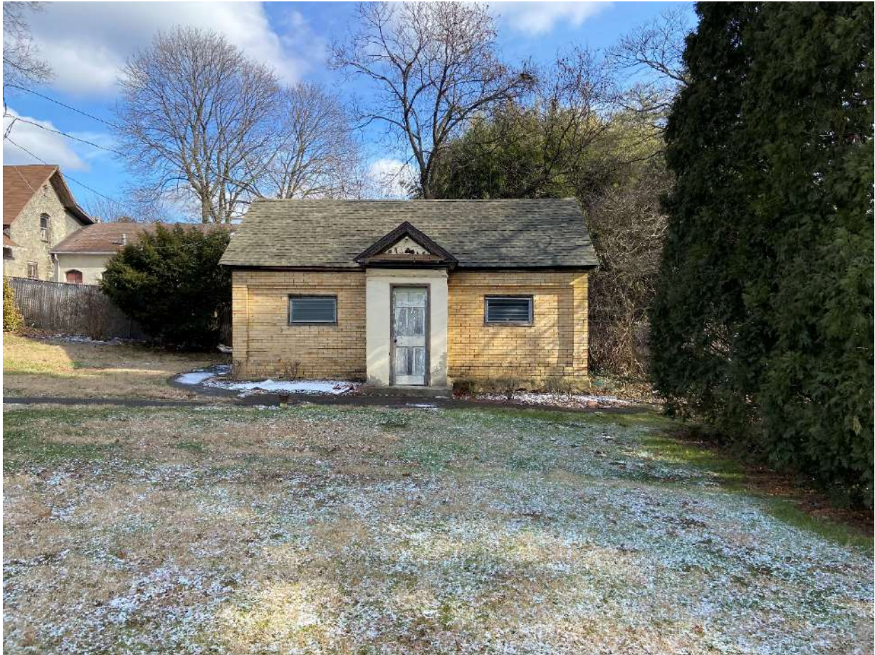
Site visit photograph, Garage/Storage Building (c1900-10)
