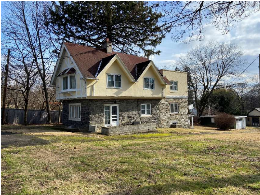
Site visit photograph, the building incorrectly referred to as the Cherry Cottage in the nomination.
