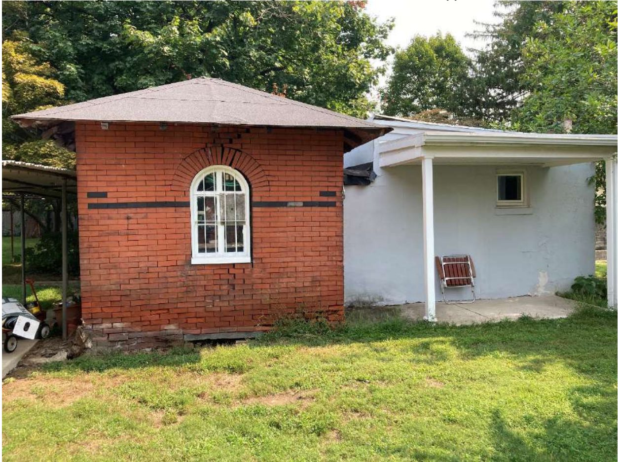
Figure 20: September 2022 photograph showing garden building A at left, with the modern garden building B at right.
