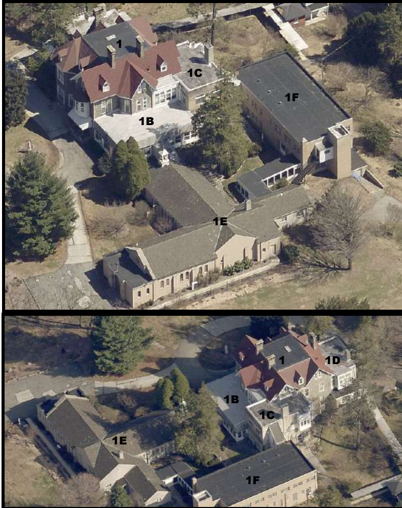
Figure 52. Top: Looking east at the Main Block and Additions 1B, 1C, 1E, and 1F of the subject property. Figure 53. Bottom: Looking north at the Main Block and the Additions of the subject property. Source: Pictometry, Atlas, City of Philadelphia, 2019.
