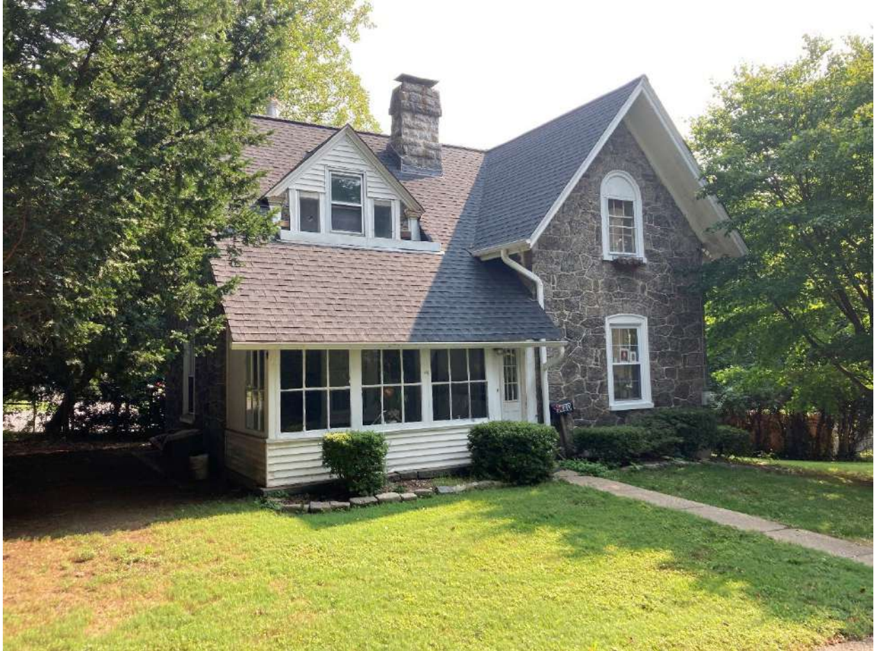
Figure 16: September 2022 image showing the gardener's cottage. View looking east.
