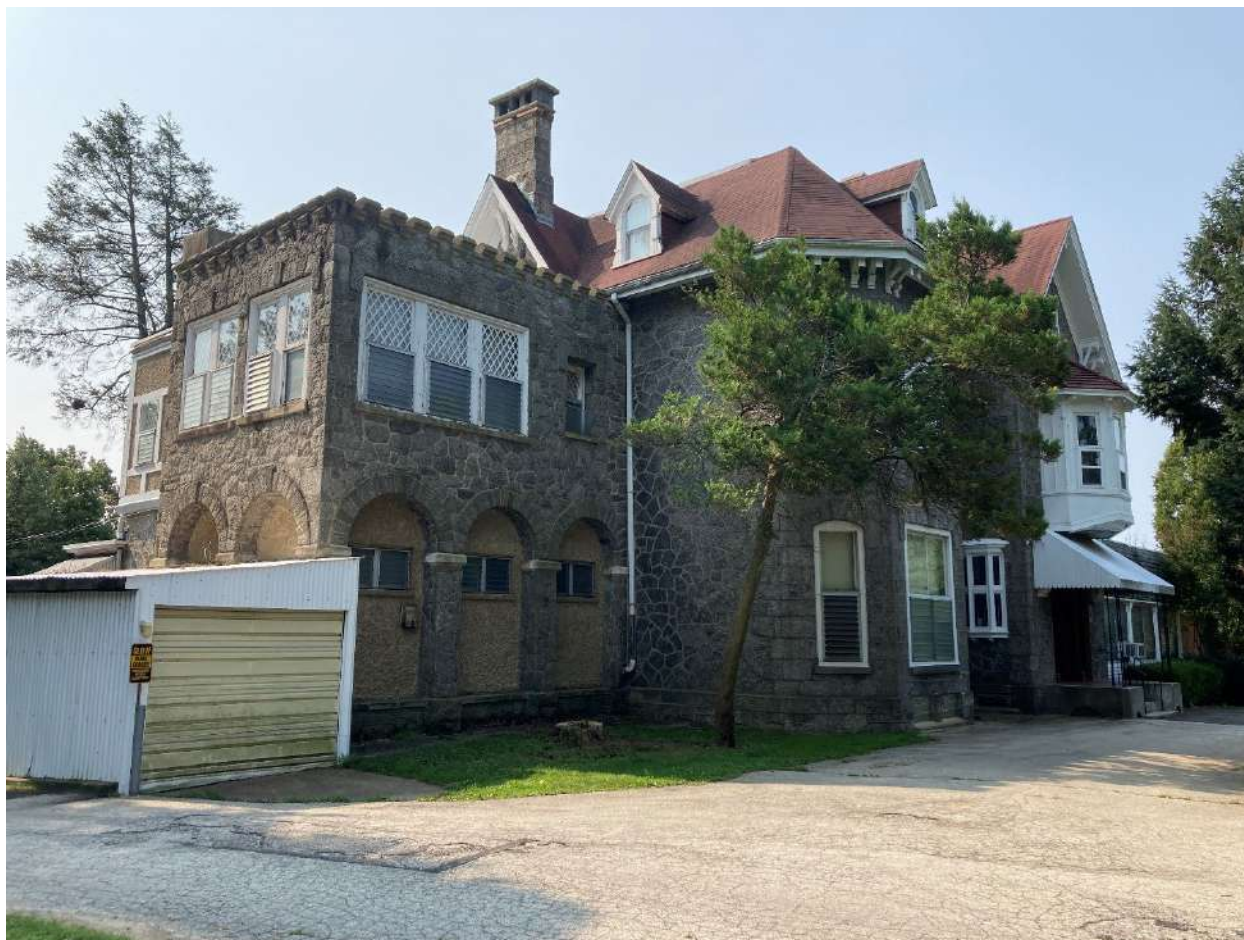
Figure 10: September 2022 photograph showing the arcade addition of the mansion house, located to the south of the main block. View looking south.
