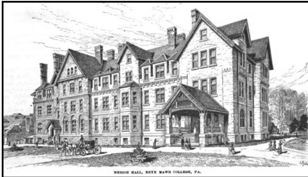
Figure 142. Merion Hall, Bryn Mawr College, Bryn Mawr, Pennsylvania, one of the buildings constructed under the leadership and philanthropy of David Scull, Jr. Source: Demorest's Family Magazine , October 1885.
