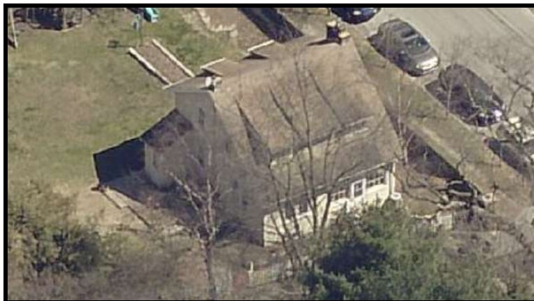
Figure 84. The northwest and primary (southwest) elevations of the Cottage 1921. Source: Pictometry, Atlas, City of Philadelphia, 2019.
