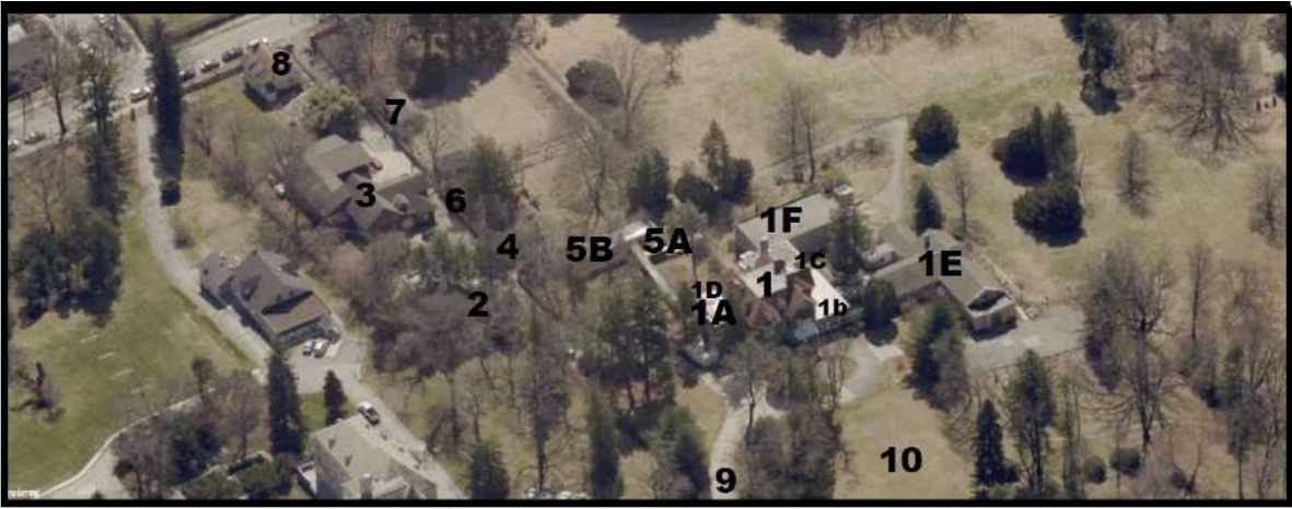
Figure 42. Top: Looking southeast at the subject property in context. Figure 43. Bottom: Looking southeast at the more specific context. Source: Pictometry, Atlas, City of Philadelphia, 2019.
