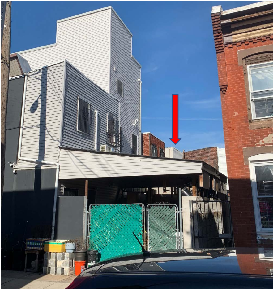
Figure 4. View of rear from Daly Street, December 2022. Only a very small section is visible, in white.
