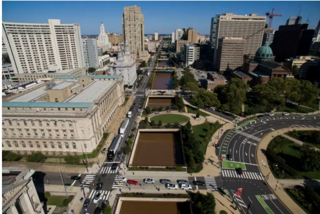
The flooded Vine Street Expressway after Ida in 2021. MONICA HERNDON / Staff Photographer
