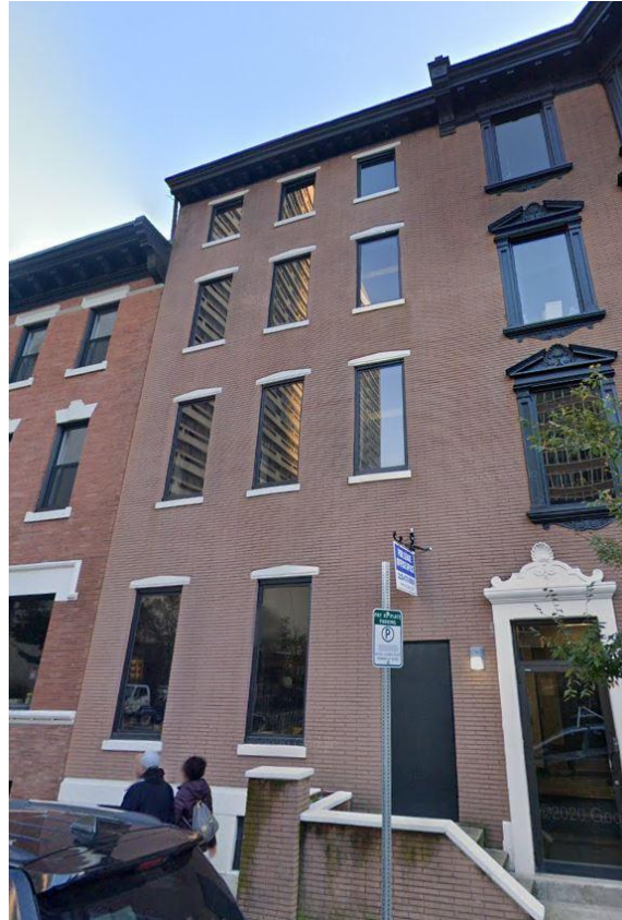
Figure 6 - 1704 Race Street, north elevation (facing Race Street).
