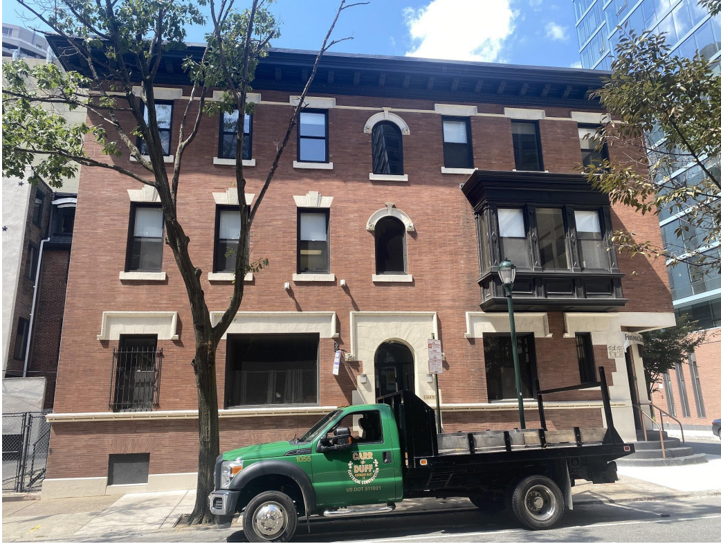
Figure 4 - 1700-02 Race Street, east elevation (facing 17th Street).
