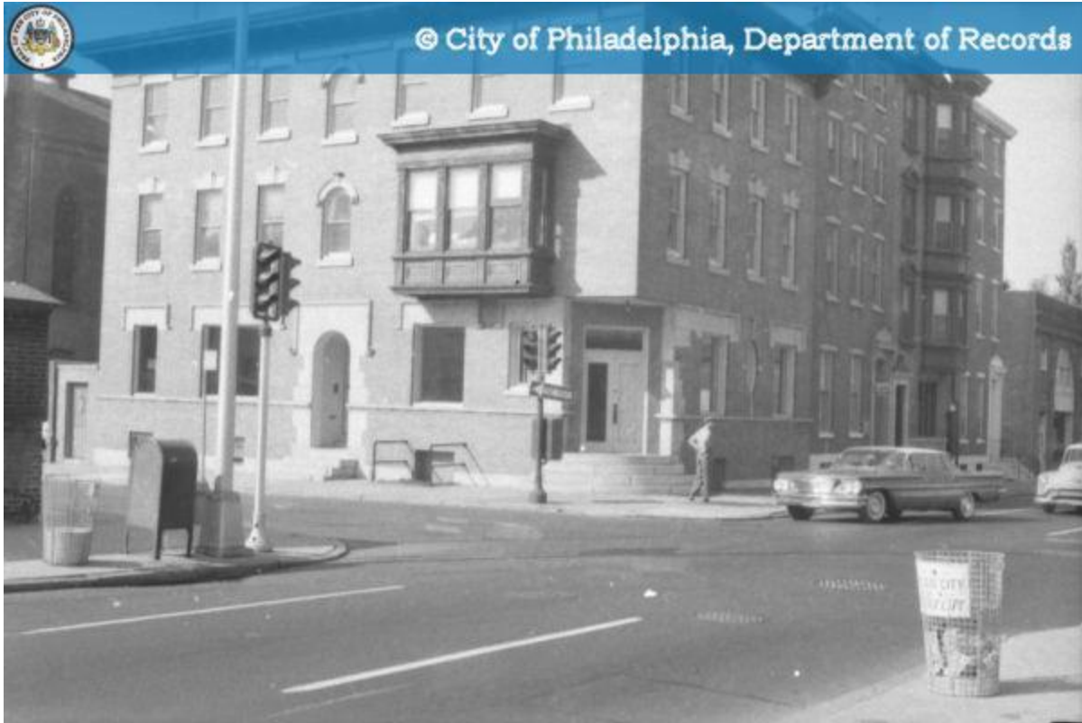
Figure 12: Looking southwest toward 1700-06 Race Street in 1960 (Phillyhistory.org).
