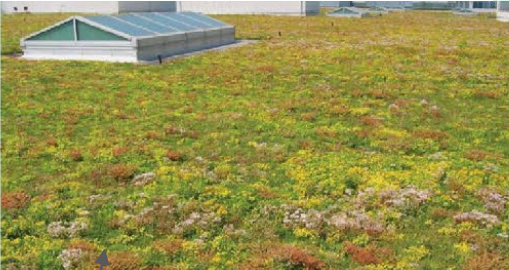
Green Roof- Sedum w/ Overseeding
