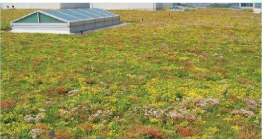
Green Roof- Sedum w/ Overseeding
