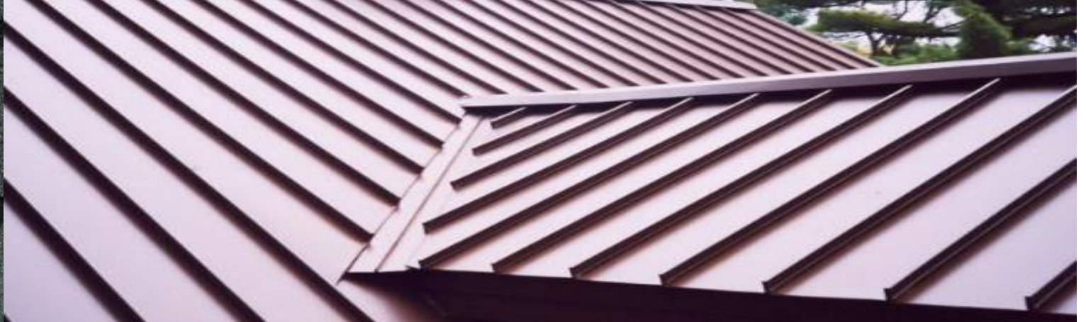
Standing Seam Metal Roof
