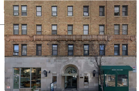
2218-2220 WALNUT MATERIALS: ORANGE BRICK WITH LIMESTONE BASE AND ALUMINUM STOREFRONT
