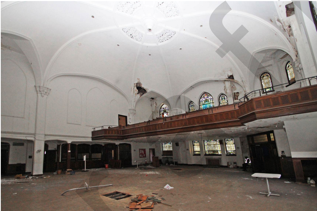
Photo 15: Sanctuary, looking southeast toward the balcony.
