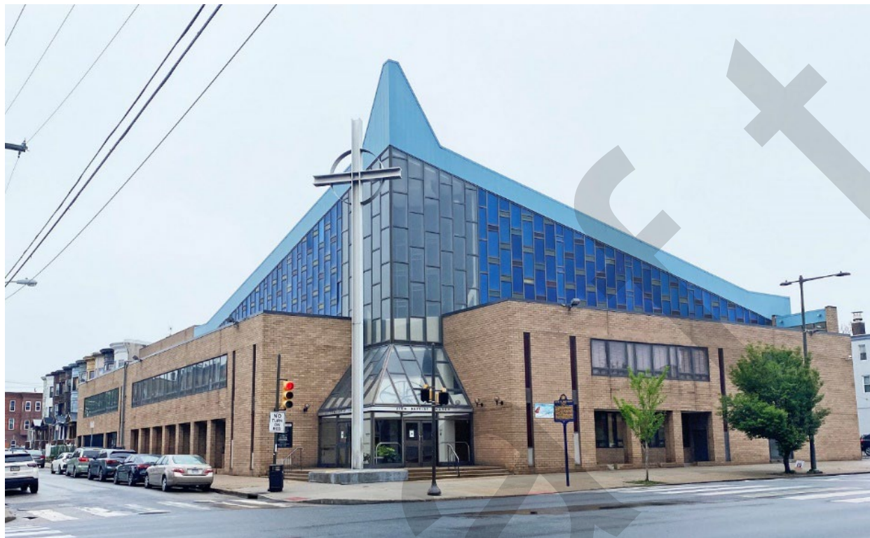
Photo 1 – South and east elevations, looking northwest from Broad Street.
