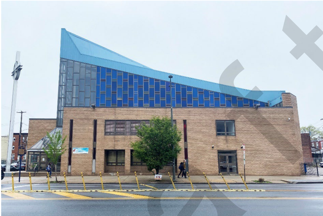
Photo 2 – East elevation, looking west from Broad Street.
