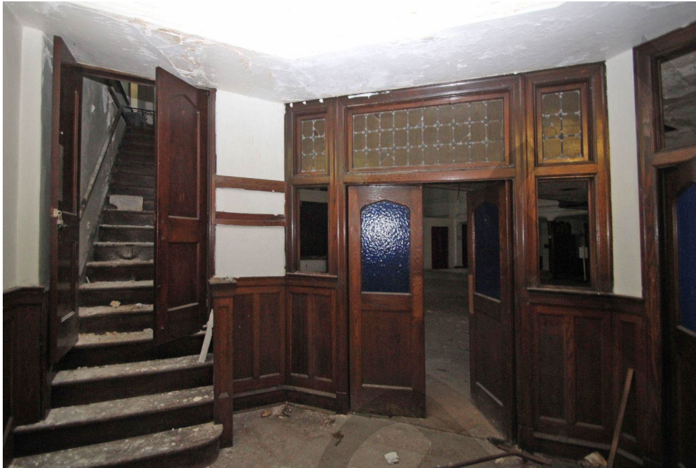
Photo 12: Vestibule, looking northeast.
