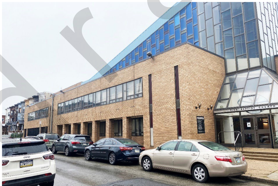
Photo 3 – South elevation, looking northwest from Venango Street.
