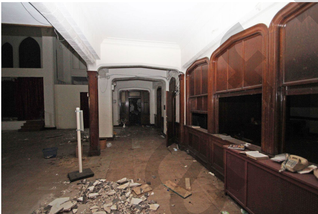
Photo 18: Passageway along east side of the sanctuary, looking north.
