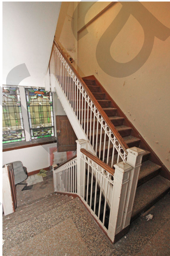
Photo 21 : Main stairway, looking southwest on the second floor.
