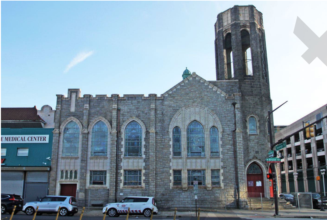
Photo 10: West elevation, looking east from Broad Street.
