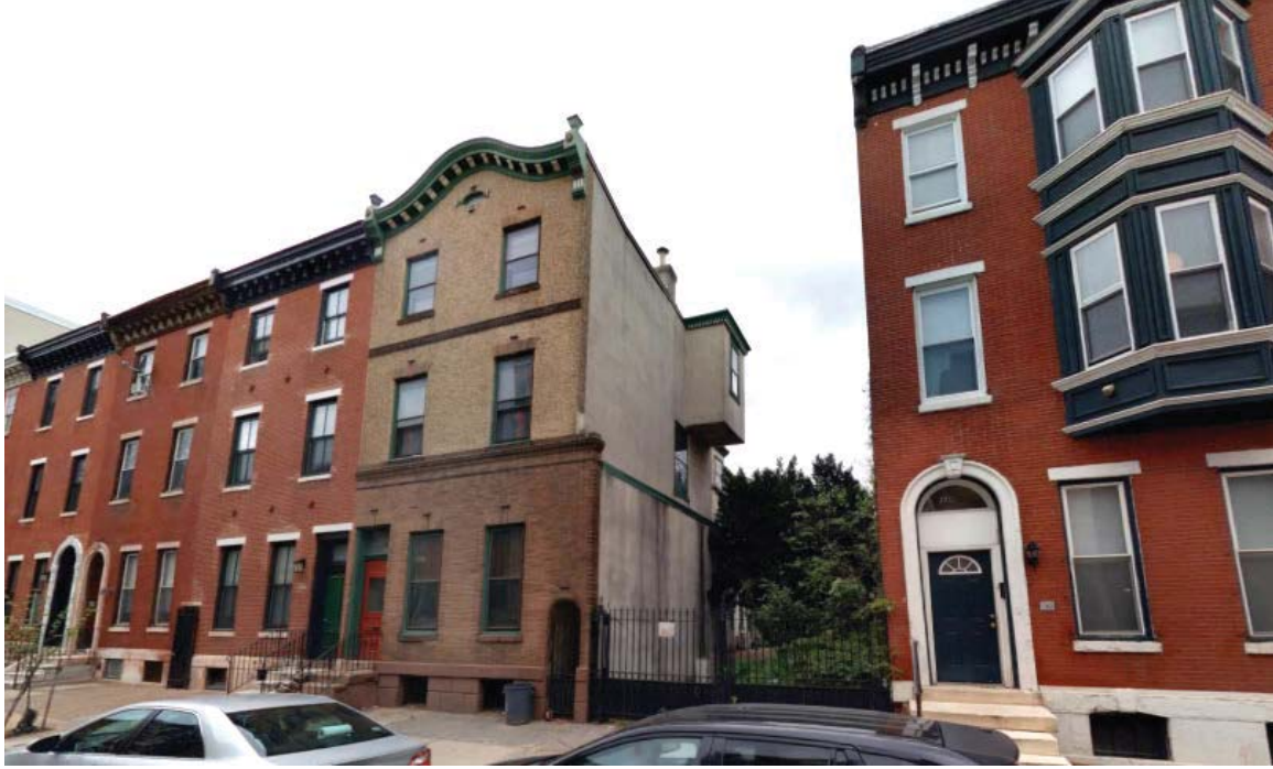
Figure 2: Streetview of 1717-19 Mount Vernon and adjacent parcels. Source: Cyclomedia.
