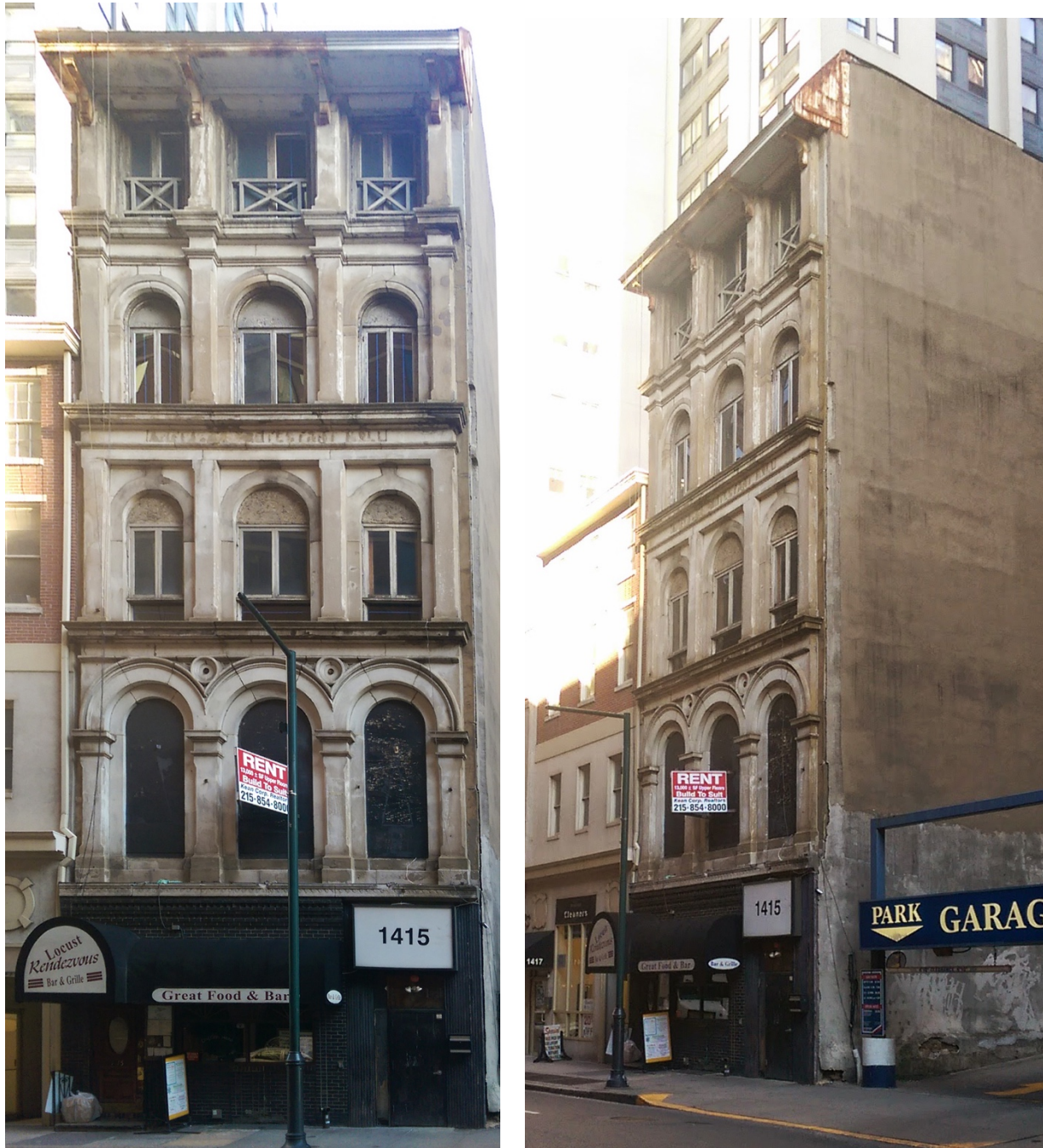
Figure 1 (left): Locust Street (south) elevation, perspective-corrected photo c.2015. Figure 2 (right): South and partial east elevations c.2015.
