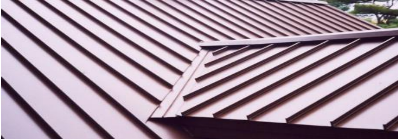
Metal Standing Seam Roofing
