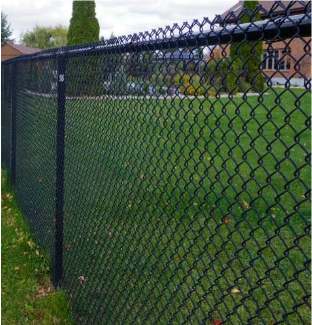
Black pvc-coated 8'-0" tall chainlink fence
