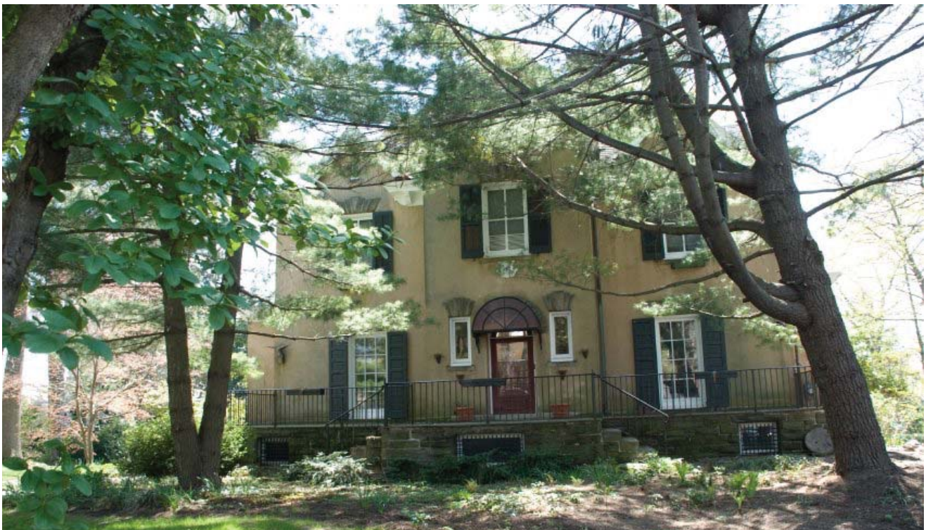
Figure 4. Main facade of The Yellowstone in 2008. Gabriella Gonzales Photograph Collection, Chestnut Hill Conservancy Archives.
