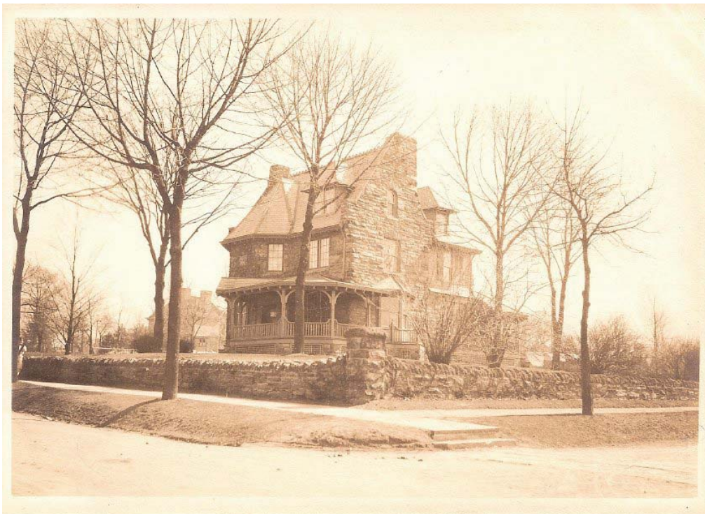
Figure 23. Chandler's Douglas house (1887) at 30 W. Chestnut Hill Ave. Photograph from the archives of the Chestnut Hill Conservancy.
