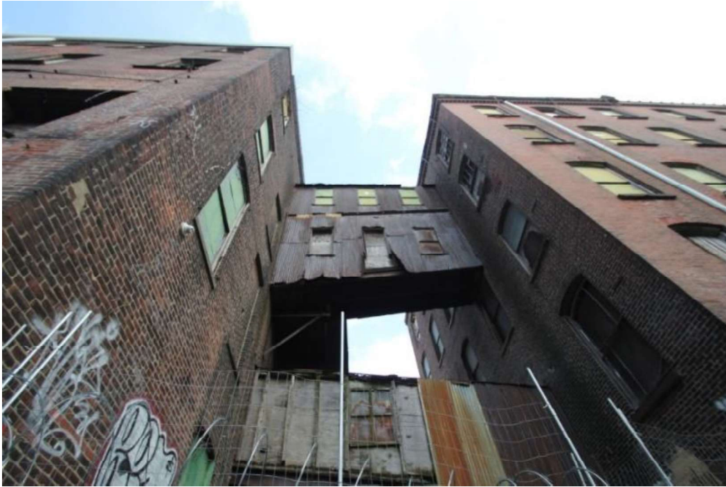
Figure 10: Bridges between Mill #1 (right) and Mill #2 (left), view west.
