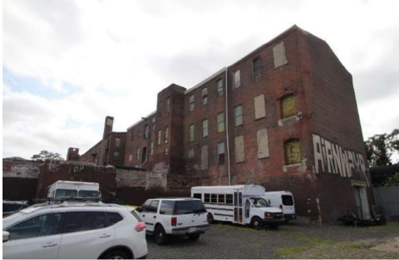
Figure 13: West and south elevations of Mill #2, view northeast.
