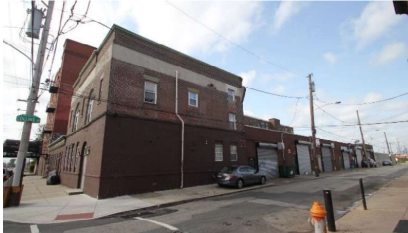
Figure 21: West elevation of the Warehouse, view southeast.
