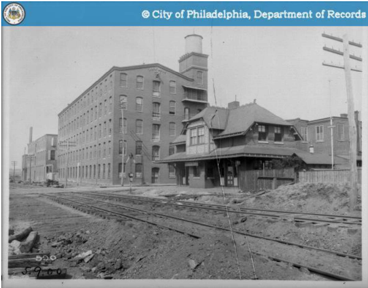
Figure 21: Looking south to Mill #1 in 1900 (Philadelphia Dept. of Records). This image shows the adjacent railroad at grade, prior to its elevation around 1909. Mill #2 also has yet to be expanded to four stories. The building in the foreground is a former Pennsylvania Railroad Depot, which was demolished when the railroad was elevated.
