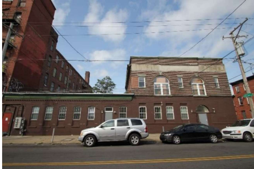
Figure 19: North elevation of the Warehouse, view south. As seen in this view and in Figures 20 and 21, below, the stucco band above the second floor windows was historically the location of a cornice as seen in Figure 4.
