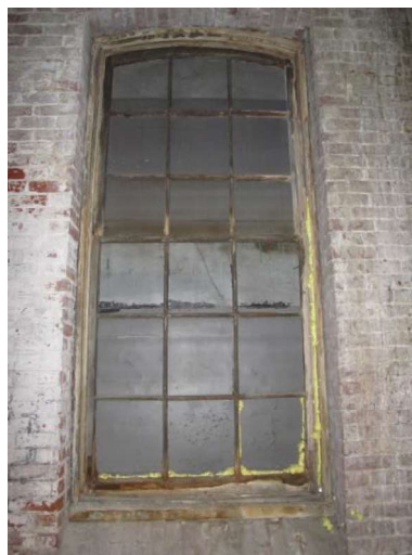
Figure 15: Typical 9-over-9 window in Mill #2.
