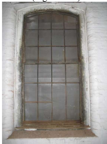
Figure 9: Typical 12-over-12 window in Mill #1.
