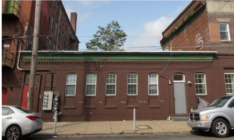
Figure 16: North elevation of the Office building, view south. The two westernmost bays (far right) were not part of the original building and were likely added shortly after 1920.
