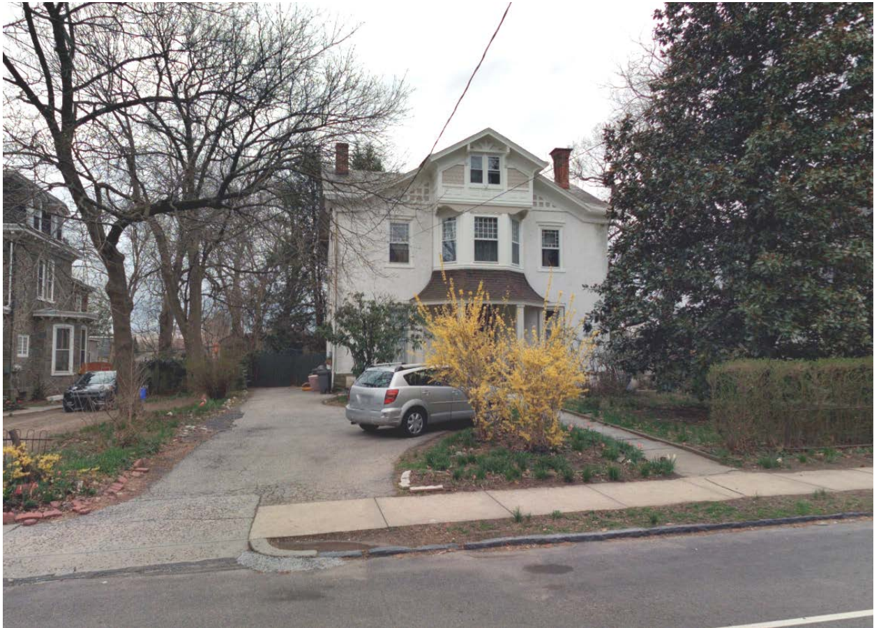
Figure 2. 138 W. Walnut Lane. View southeast from W. Walnut Lane, 17 April 2018. Source: Cyclomedia.
