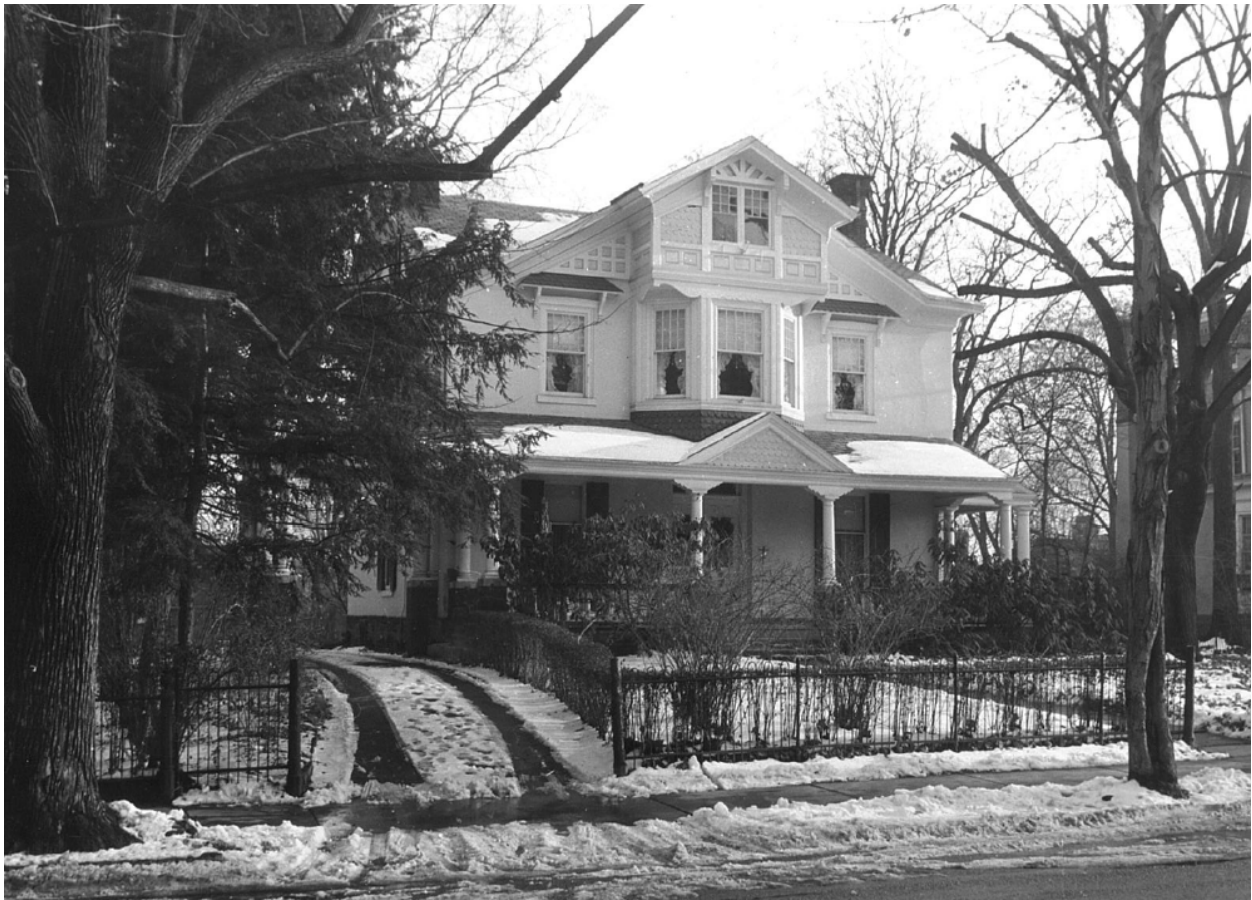
Figure 20. Photograph of the property in 1963. Source: Philadelphia Historical Commission.
