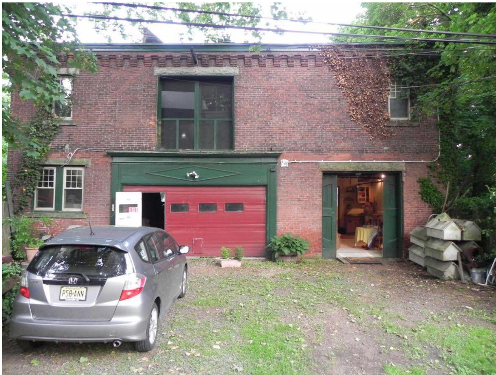
Figure 12. Front facade of the carriage house.
