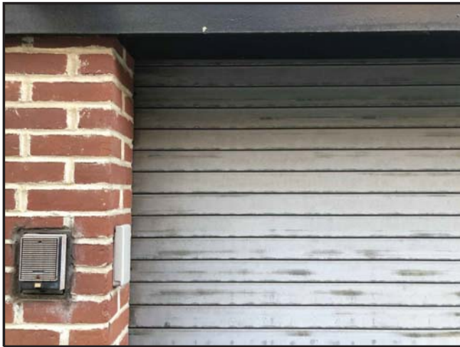
(FROM SIDEWALK ON SOUTH SIDE OF CYPRESS STREET-1) 11-28-2020
