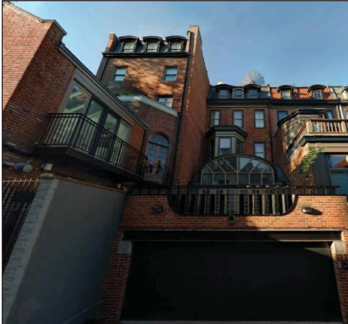
2019/2021 DELANCEY PLACE @ CYPRESS STREET
