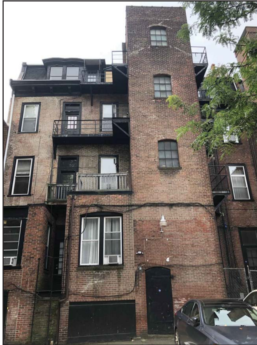
2011 DELANCEY PLACE @ CYPRESS STREET
