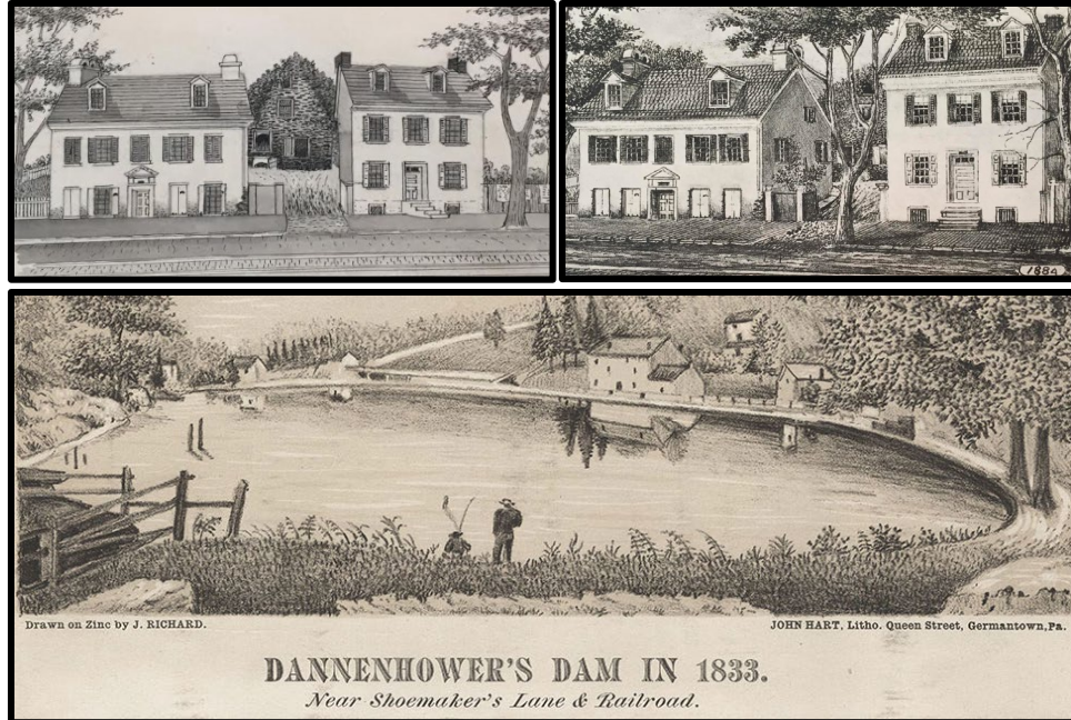
Figures 42. and 43. Top: Two views drawn by John Richards in 1884, depicting, left to right, the Jacob Muller House, an old bake house at the rear, and the George Dannenhower House (ca.1745), all of which stood near the present site of E. Clapier Street. Source: Germantown Historical Society. Figure 44. Bottom: “Dannenhower’s Dam in 1833” looking towards E. Penn Street, on the property Johann Eckstein purchased in 1736, drawn on Zinc by John Richard in 1868. Source: Free Library of Philadelphia.
