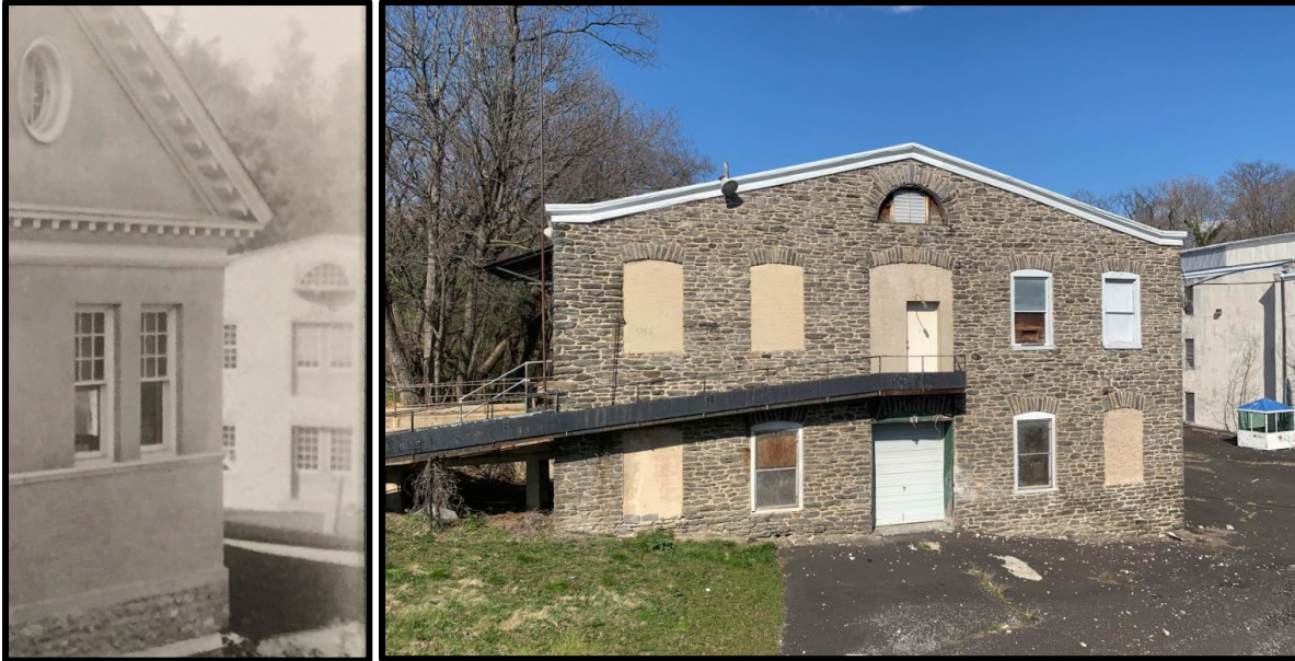
Figure 20. Left: Looking north from the Philadelphia Gas Works' at Germantown across Belfield Avenue at the newly completed Building 3 in 1903. Source: The Philadelphia Gas Works Photograph Collection, City Archives of Philadelphia. Figure 21. Right: The primary (south) elevation of Building 3. Source: Oscar Beisert, 2020.
