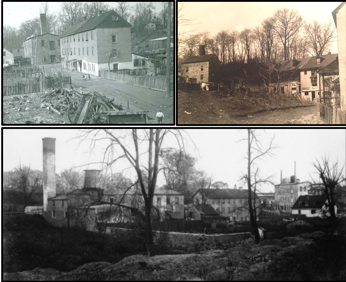
Figure 51. Top left: The Wakefield Mills at Fisher's Hollow, near Lindley and Belfield Avenues, built by William Logan Fisher, photographed by John G. Bullock ca. 1913. All but one building of this complex has been demolished. Source: The John C. Bullock Lantern Slide Collection, The Library Company of Philadelphia. Figure 52. Top right: Harper's Hollow, a mill complex, at Thorpe's Lane and Old York Road near Germantown, taken by Edwin Costley Jellet. Source: The Germantown Historical Society. Figure 53. Bottom: The Wakefield Mills at Fisher's Hollow near Lindley and Belfield Avenues in 1900. Source: Irvin Miller and Judith Callard. Remembering Germantown, 60 Years of the Germantown Crier . (Arcadia Publishing, 2008).
