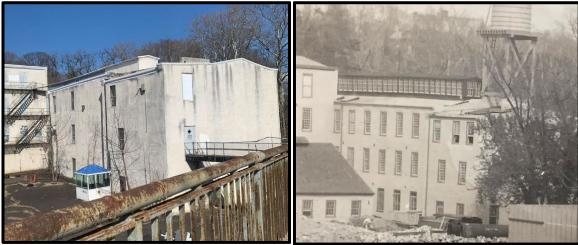
Figure 9. Left: Looking northeast at Buildings 1 and 6. Source: Oscar Beisert, 2020. Figure 10. Right Looking northeast at Buildings 1 and 6 in 1902. Source: The Philadelphia Gas Works Photograph Collection, City Archives of Philadelphia.
