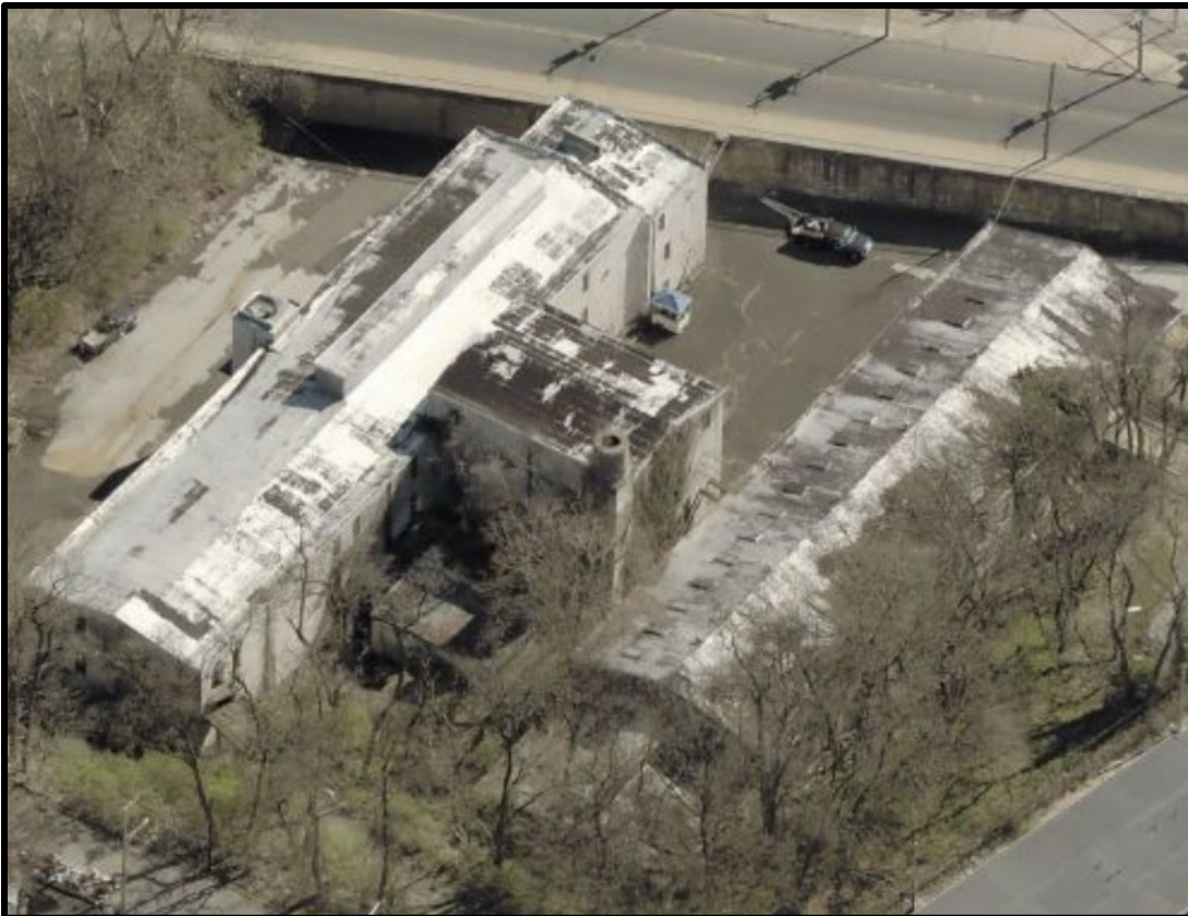
Figure 18. Top: The primary (south) elevation of Building 2. Source: Oscar Beisert, 2020. Figure 19. Bottom: A bird's eye view of the subject property with the rear (north) and side (west) elevations circled. Source: Pictometry, Atlas, City of Philadelphia.
