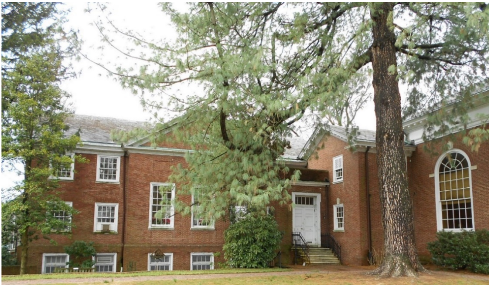
Figure 14: Parish Hall on southeast end of church. Nancy Pontone, March 2019.
