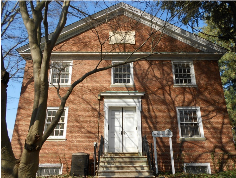
Figure 16: Gable end of Parish Hall looking northwest. Nancy Pontone, January 2019.
