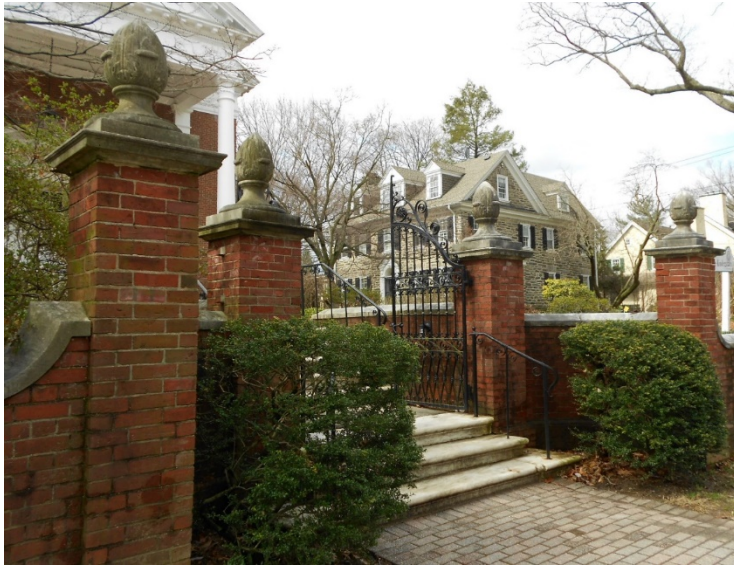
Figure 8: Church gate posts and front steps looking west. Nancy Pontone, January 2019.
