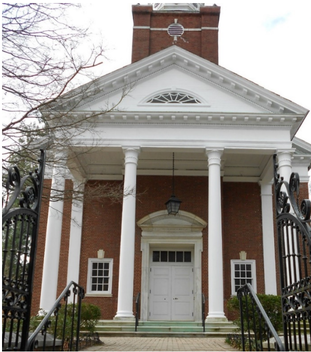
Figure 11: Front elevation of church looking southwest. Nancy Pontone, March 2019.
