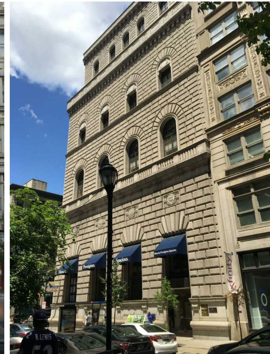
5 LOOKING NORTHWEST AT WALNUT STREET FACADE
