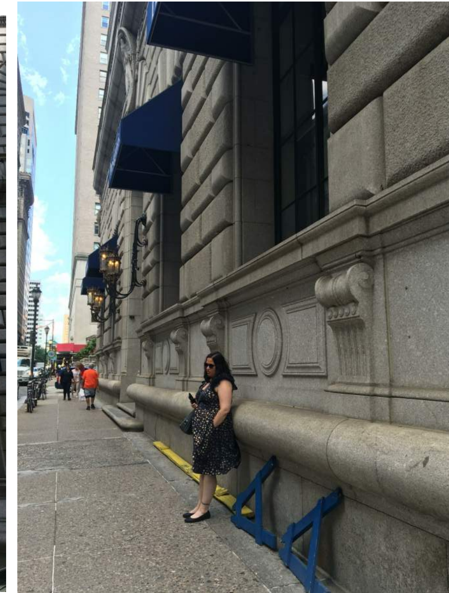
8 ALONG 15TH ST FACADE
