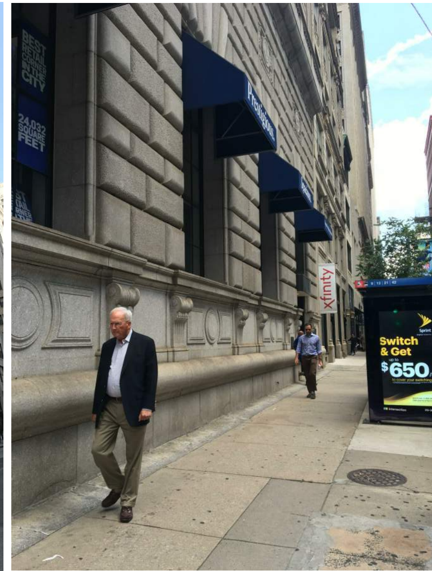
2 LOOKING ALONG WALNUT ST FACADE
