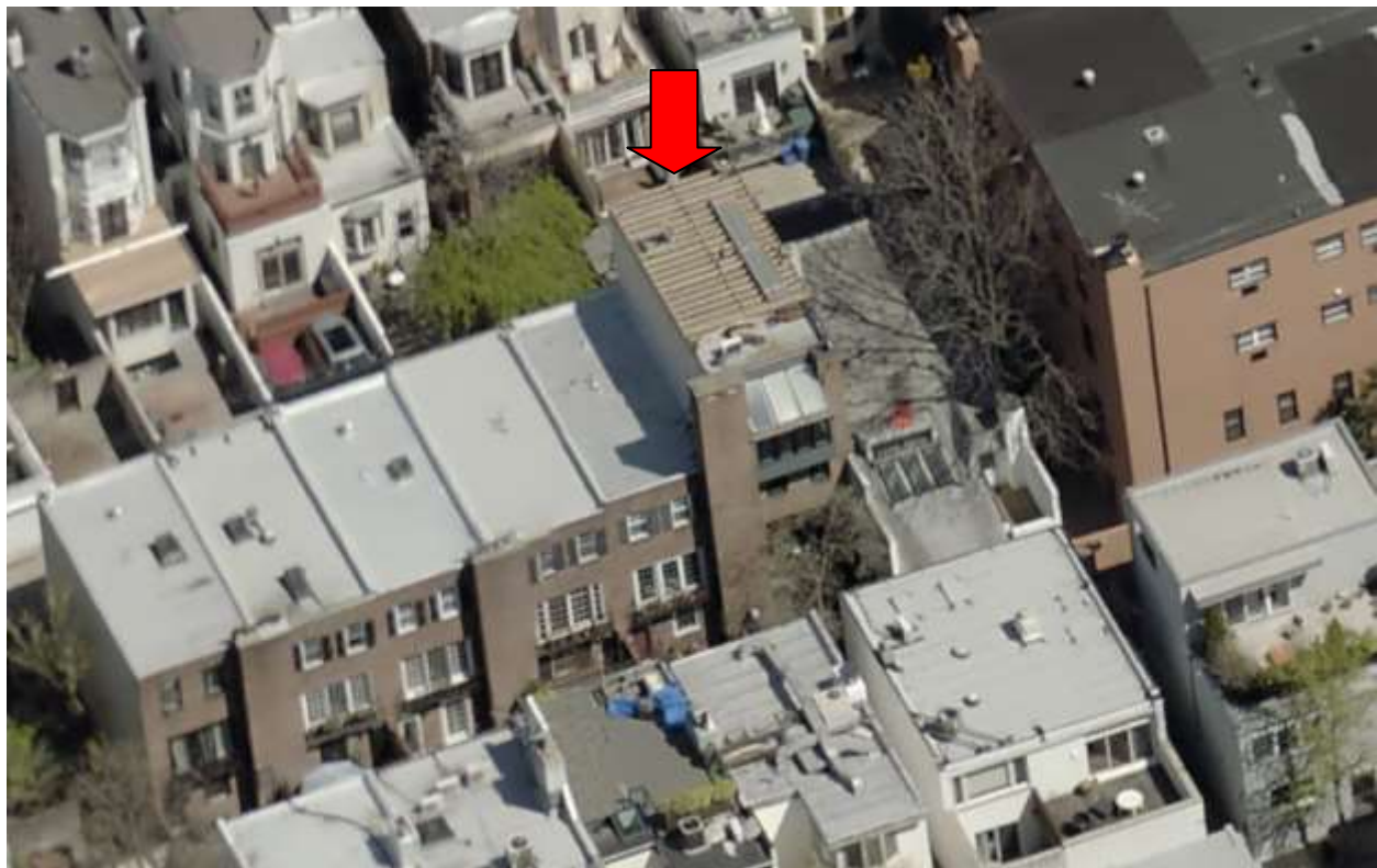
Figure 2: The courtyard façade of 2411 Delancey Place, Unit A, prior to demolition, 2020. Source: Pictometry.
