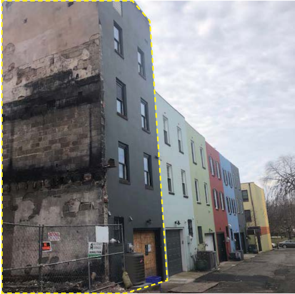
(5) VIEW WEST ON CYPRESS ST
