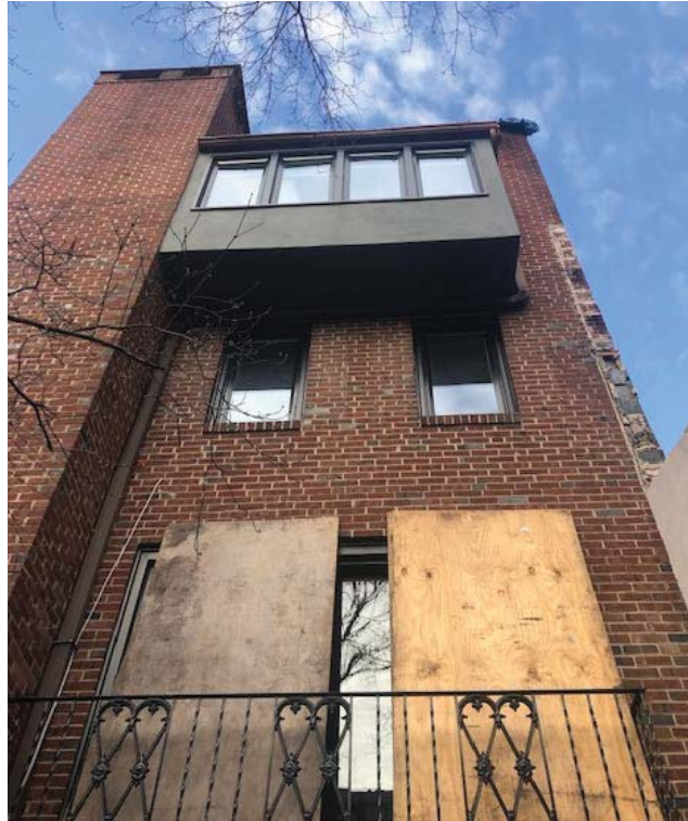
(2) VIEW FROM INTERIOR OF COURTYARD OF RECENTLY DEMOLISHED STRUCTURE
