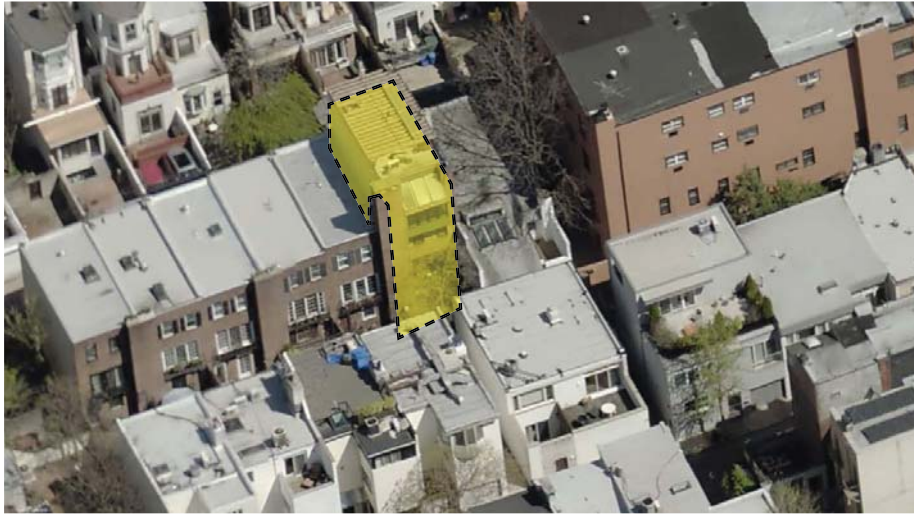
AERIAL VIEW - SOUTH (RECENTLY DEMOLISHED 4 STORY STRUCTURE SHOWN)
