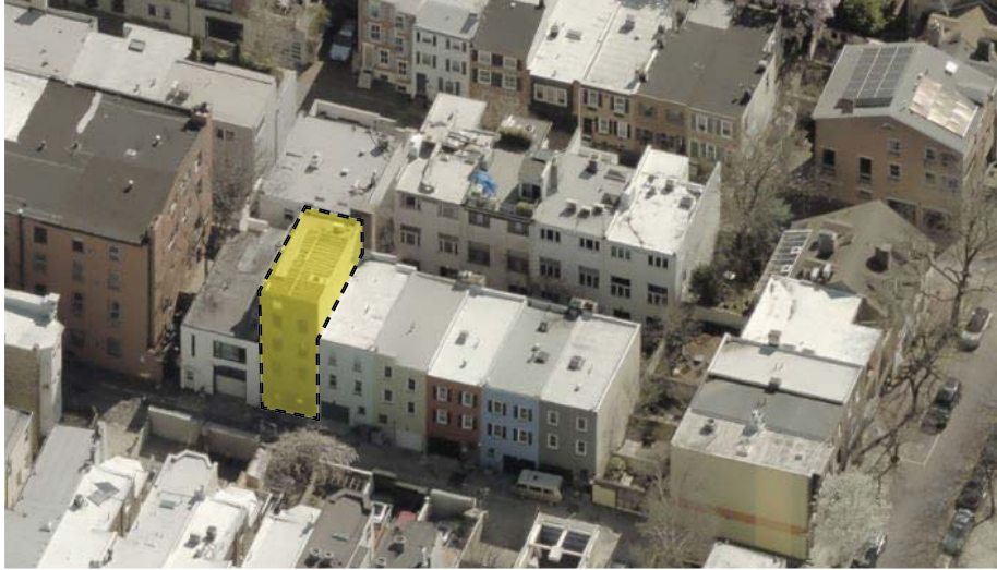
AERIAL VIEW - NORTH (RECENTLY DEMOLISHED 4 STORY STRUCTURE SHOWN)
