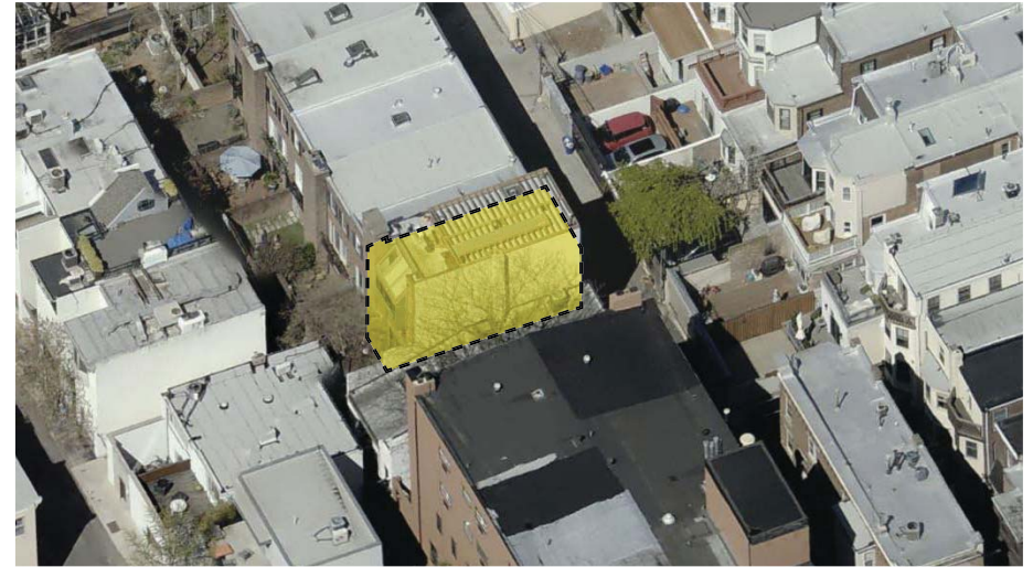
AERIAL VIEW - WEST (RECENTLY DEMOLISHED 4 STORY STRUCTURE SHOWN)
