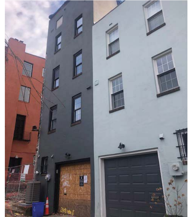
(3) VIEW OF REAR ELEVATION FROM CYPRESS ST OF RECENTLY DEMOLISHED STRUCTURE
