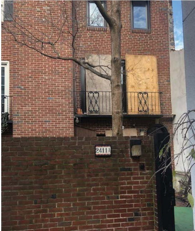
(1) VIEW FROM INTERIOR ENTRY COURT OF RECENTLY DEMOLISHED STRUCTURE
