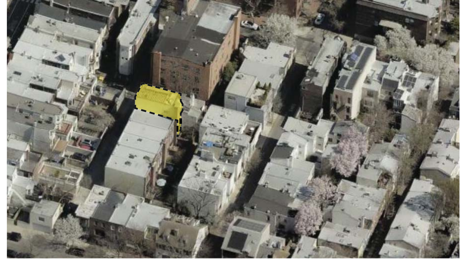
AERIAL VIEW - EAST (RECENTLY DEMOLISHED 4 STORY STRUCTURE SHOWN)
