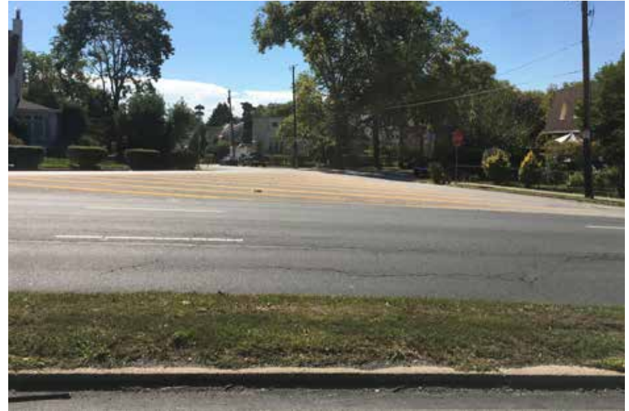
Figure 6-2. Ramona Avenue/Foulkrod Street and Roosevelt Boulevard (see Figure 6-17)
