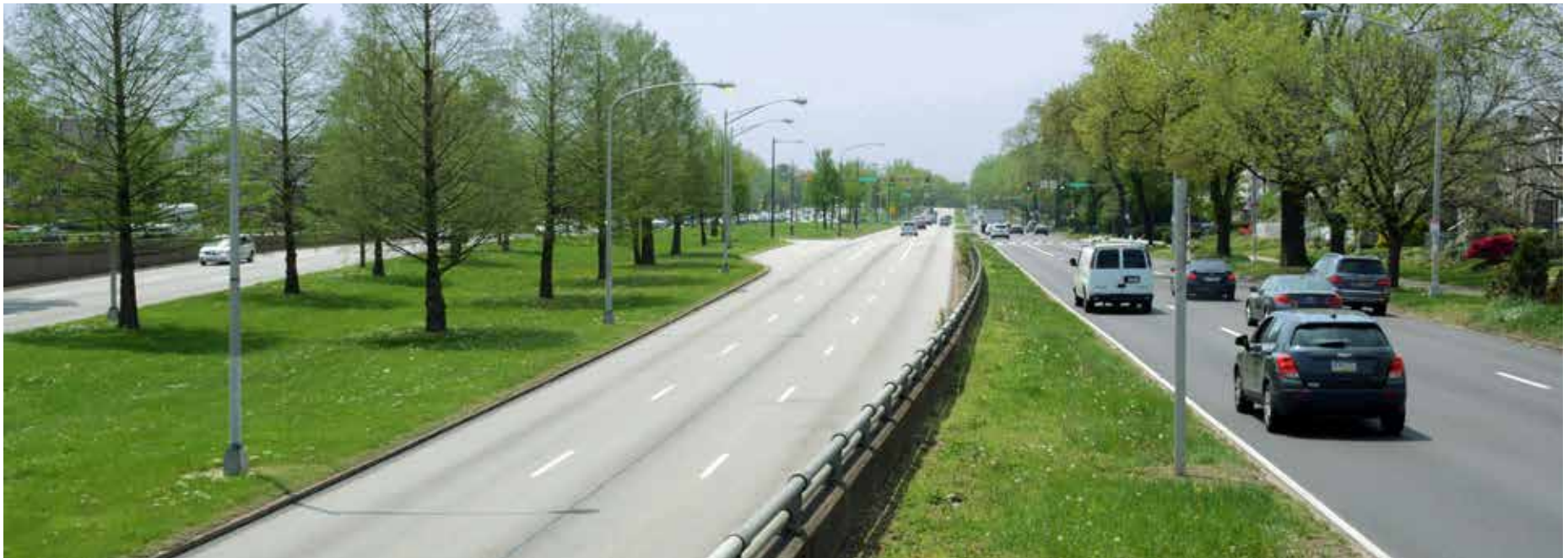
Figure 2-21. Segment 3 between Sanger Street and Bridge Street
