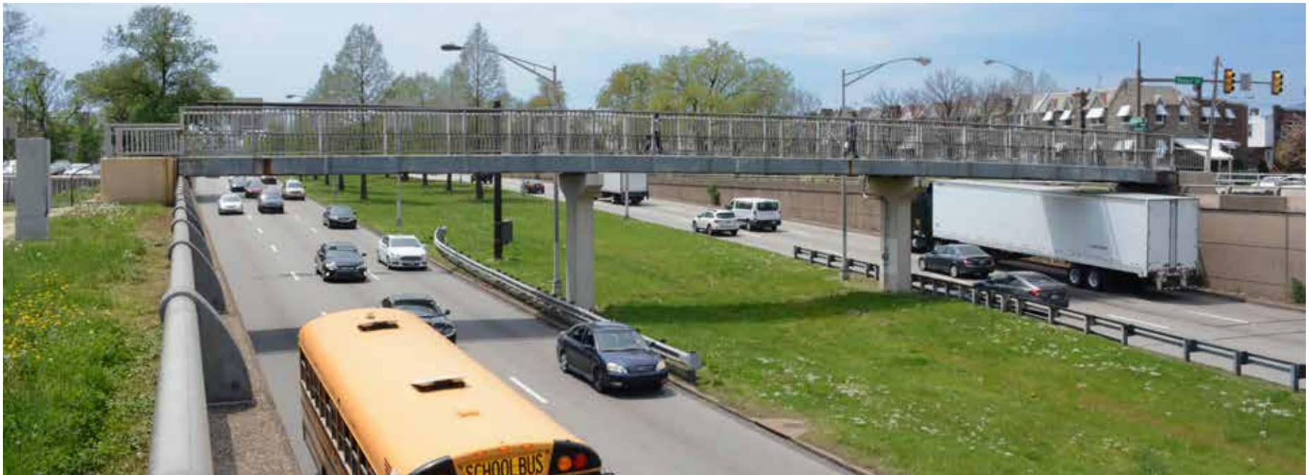
Figure 2-8. Grade-Separated Pedestrian Bridge Crossing at Sanger Street
