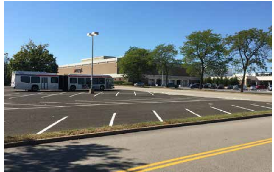
Figure 2-25. Segment 6 at Neshaminy Mall
