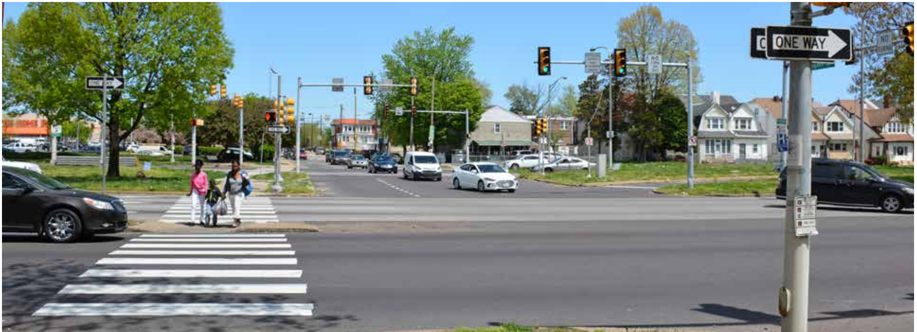
Figure 2-9. Long Crossing Distances and narrow medians at Landgon Street make crossing a challenge.
