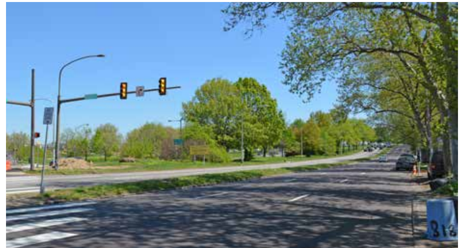
Figure 2-16. Example of On-Street Parking
