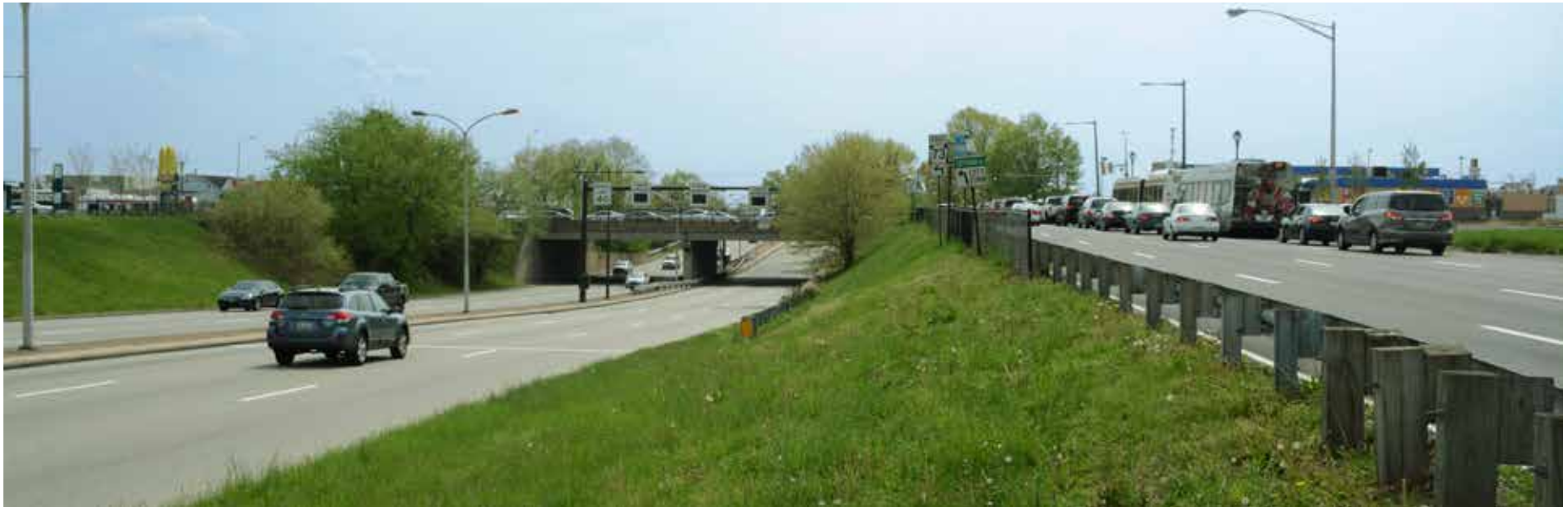
Figure 2-23. Segment 4 at Cottman Avenue
