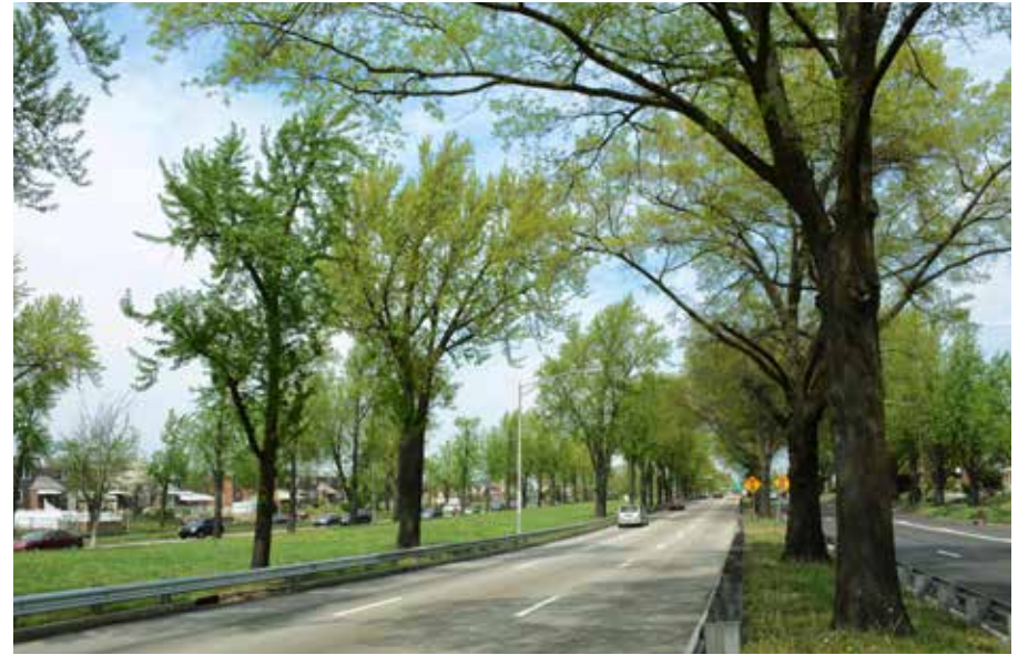
Figure 5-19. Narrow Side Median with Mature Trees
