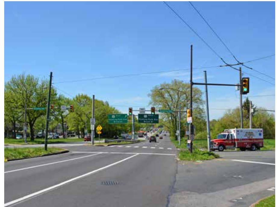
Figure 5-2. Traffic Signals at Wyoming Avenue and Roosevelt Boulevard
