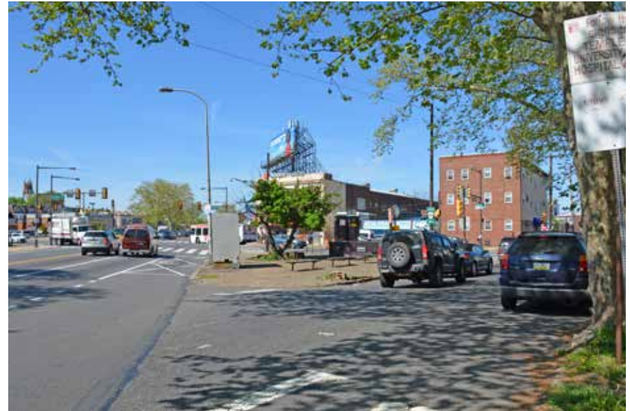
Figure 6-3. W. Bristol Street and Roosevelt Boulevard (see Figure 6-4)
