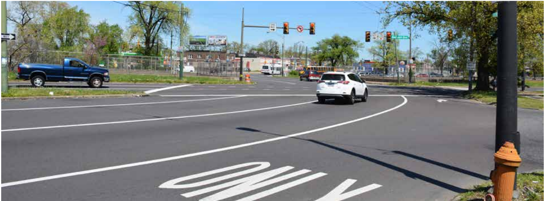
Figure 4-14. Oxford Circle at Roosevelt Boulevard
