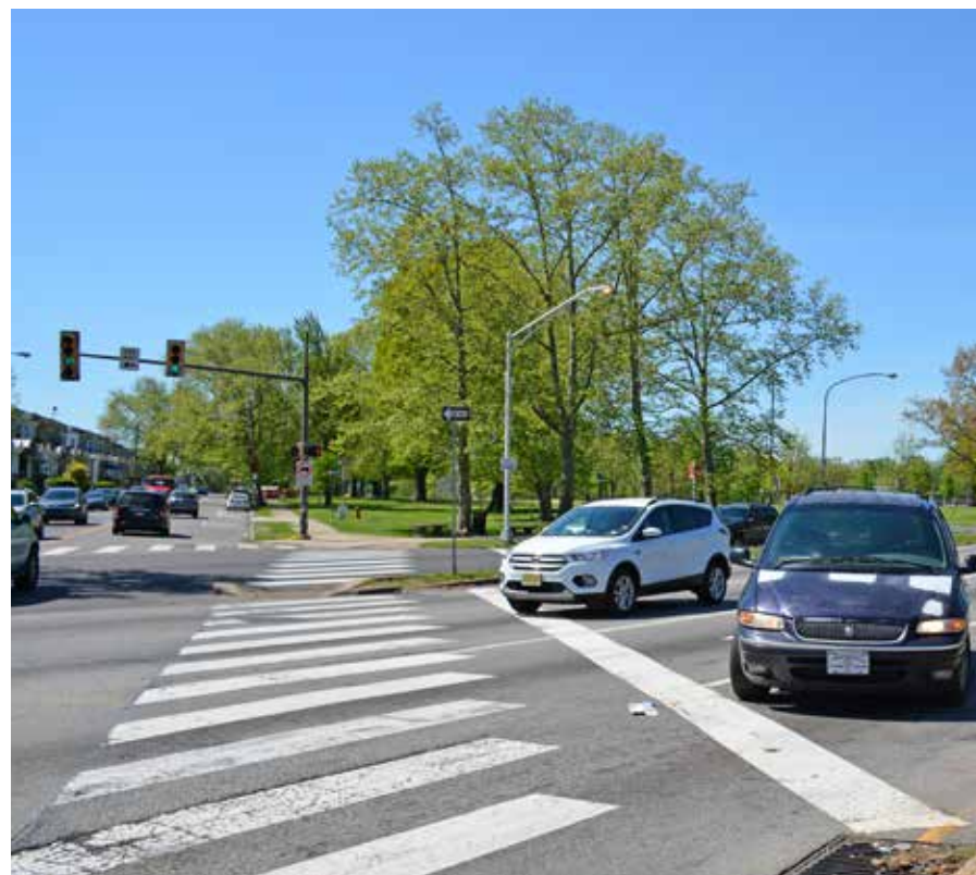
Figure 5-3. Skewed Crosswalk at Ninth Street and Roosevelt Boulevard
