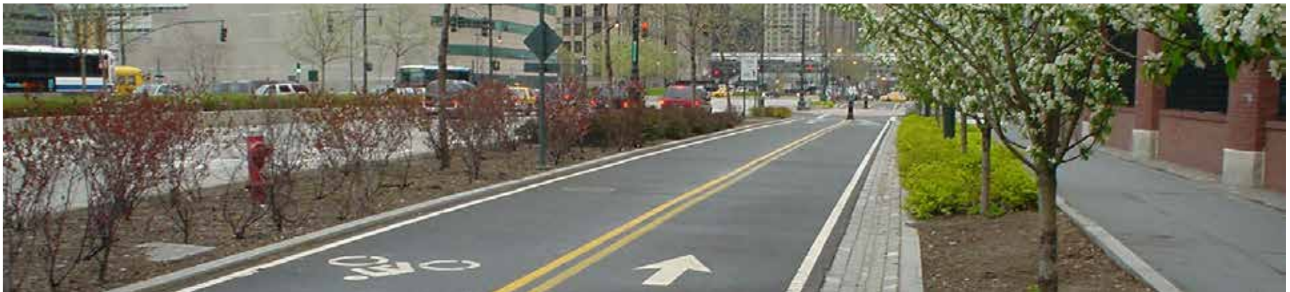
Figure 8-5. Example of Two Way Cycle Track
