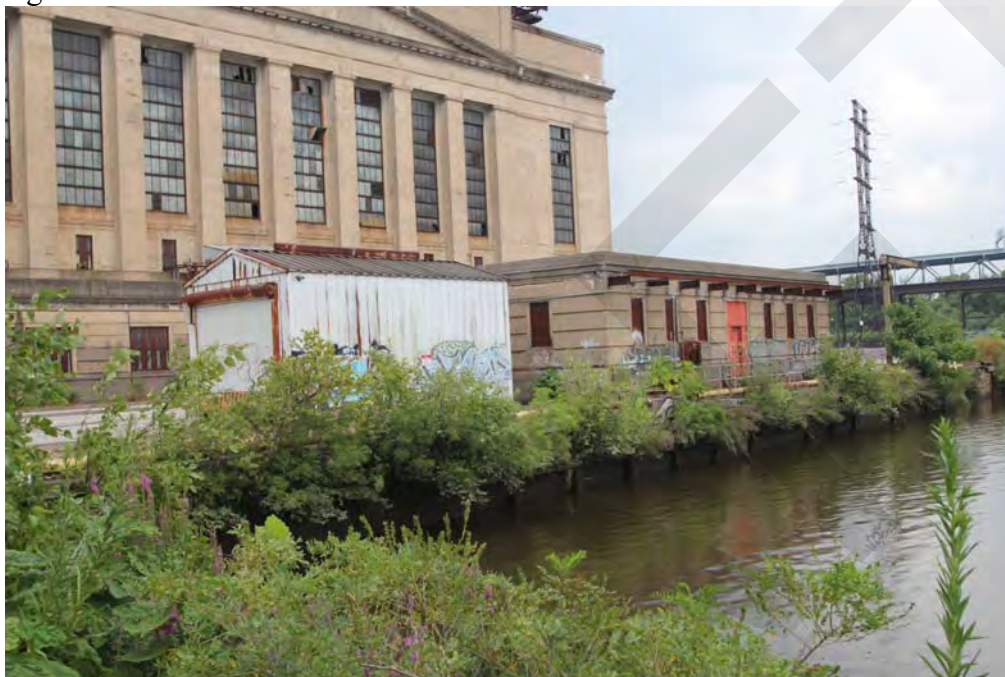
Photo 37 - Storage Shed, looking northwest from Pier 225.
