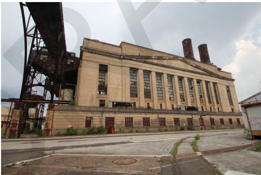
Photo 1 - Boiler House, east elevation, looking northwest. The coal conveyer is seen at far left.
