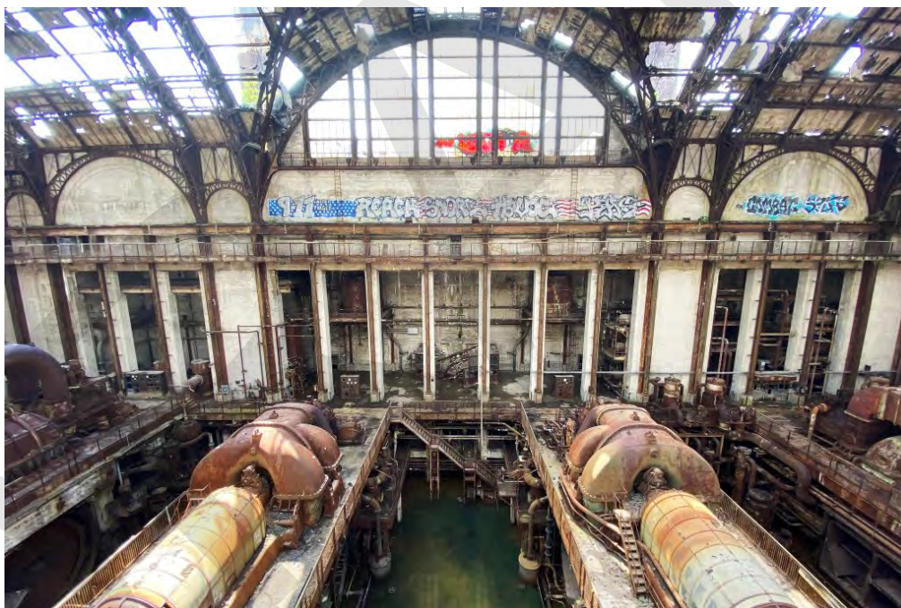
Photo 14 - Turbine Hall, looking east from the fourth floor control room.
