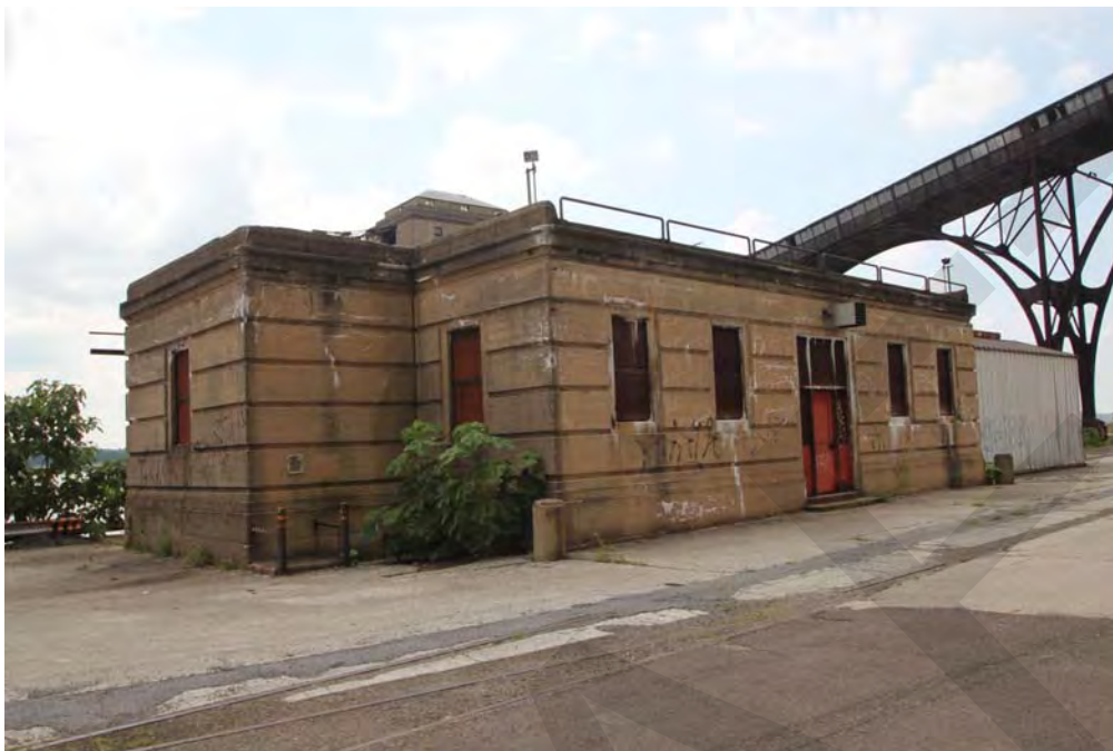
Photo 28 - Screenhouse, north and west elevations, looking southeast.
