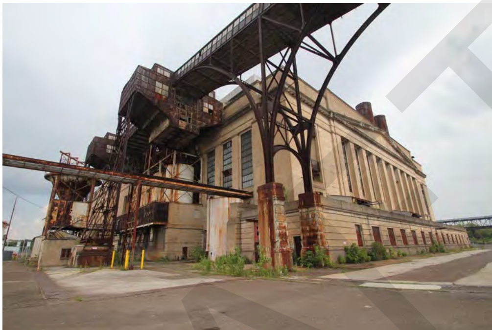
Photo 4 - Boiler House, south and east elevations, looking northwest.
