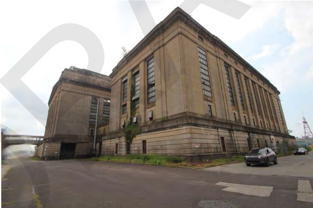
Photo 8- Switch House, north and west elevations, looking southeast.
