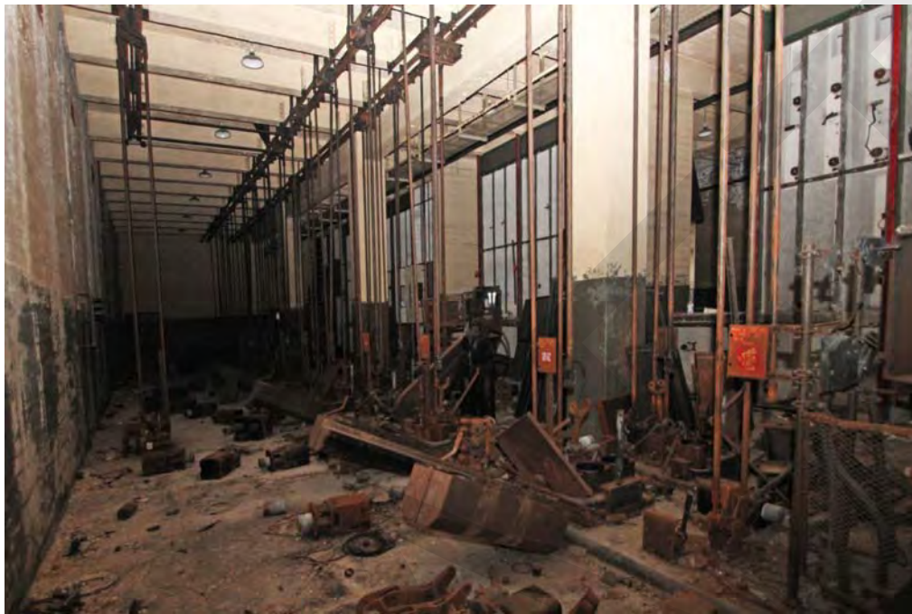
Photo 23 - Switch House, second floor, looking north.
