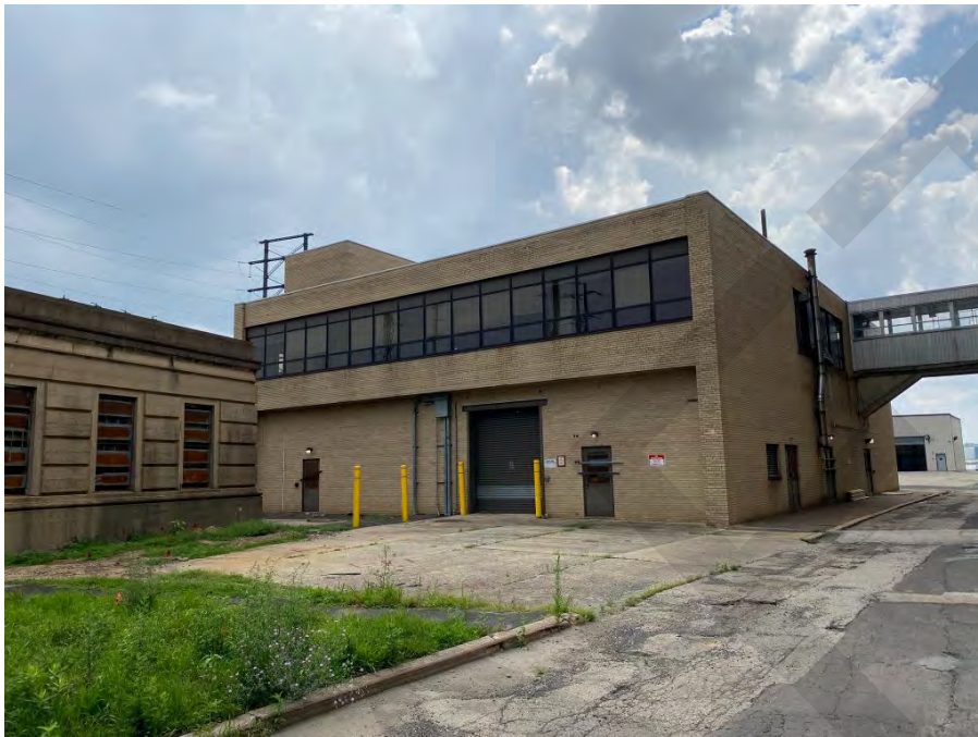
Photo 35 - Utility Building, west and south elevations, looking northeast.
