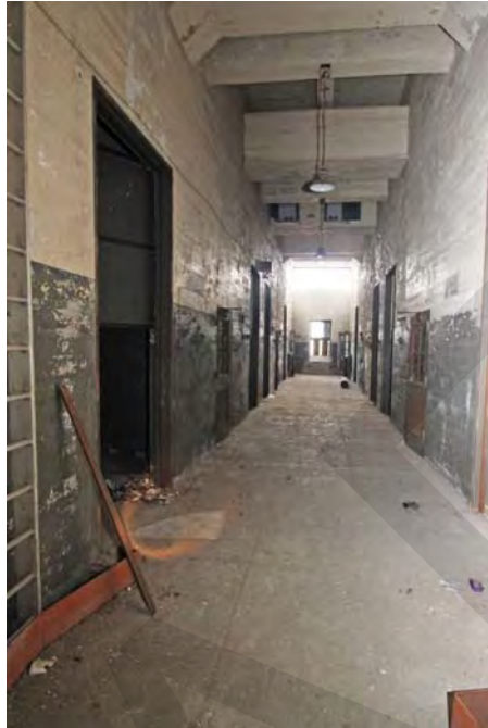
Photo 21 - Switch House, second floor corridor, looking west.
