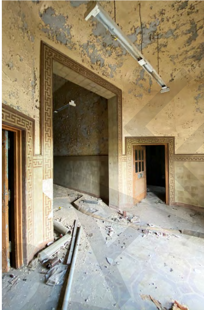
Photo 20 - Switch House, first floor vestibule, looking southeast.
