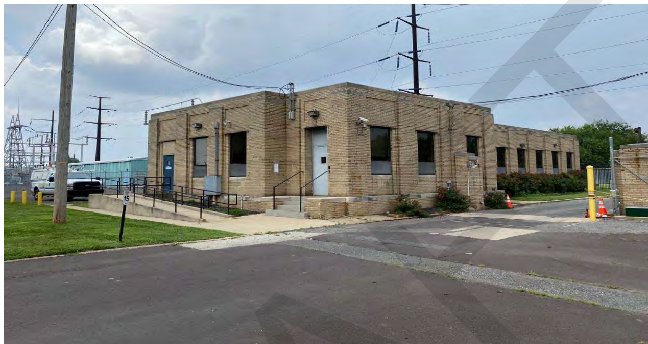
Photo 32 - Administration Building, east and north elevations, looking southwest.
