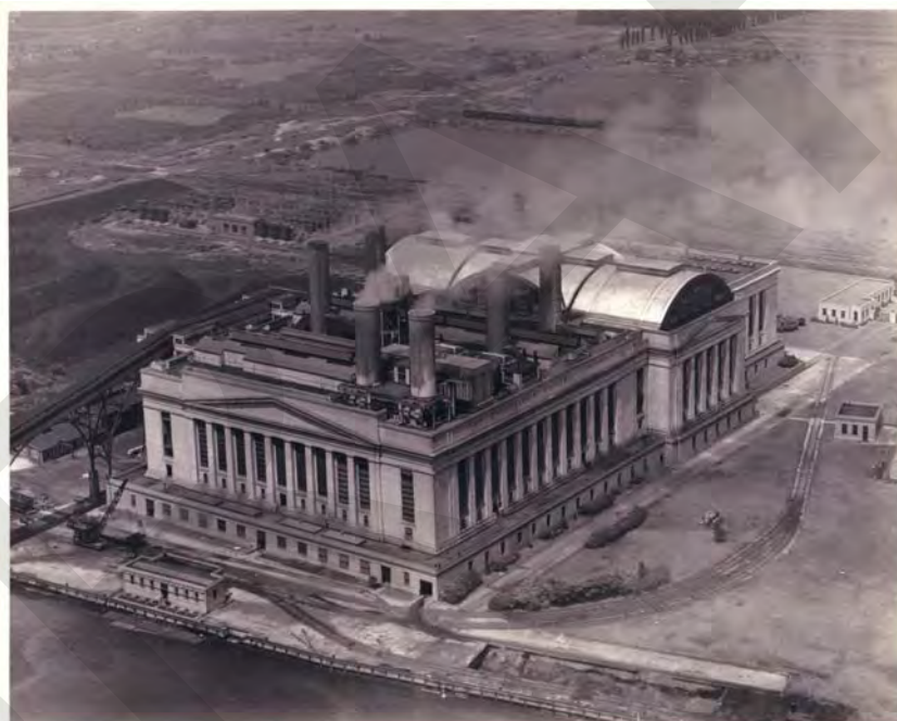
Figure I - This 1941 photo shows the two exhaust stacks that were added to the northeast corner of the Boiler House in 1932 with the installation of the new Westinghouse turbogenerator. The photo was taken by the Dallin Aerial Survey (Hagley).
