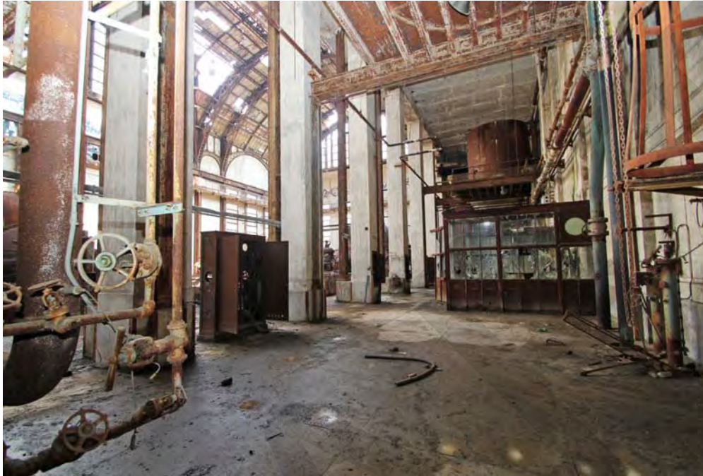
Photo 15 - Turbine Hall, heater gallery, looking north.
