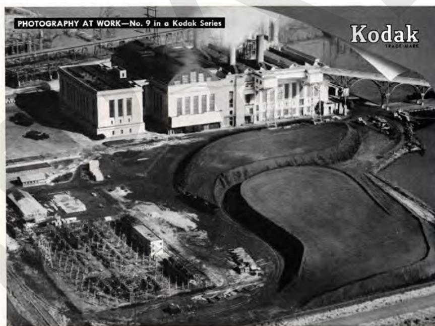
Figure J - In this 1955 Kodak advertisement, which appeared in several national magazines, including Fortune and Newsweek, the use of the site south of the Power Station for coal storage is depicted. The outdoor substation is seen at far left. The photo was taken by the Aero Service Corporation of Philadelphia.
