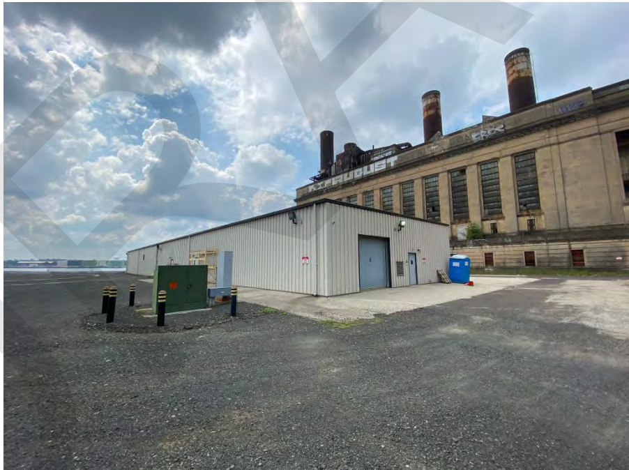
Photo 39 - Storage Building, north and west elevations, looking southeast.
