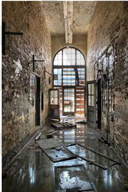
Photo 22 - Switch House, second floor corridor, looking east to Turbine Hall.
