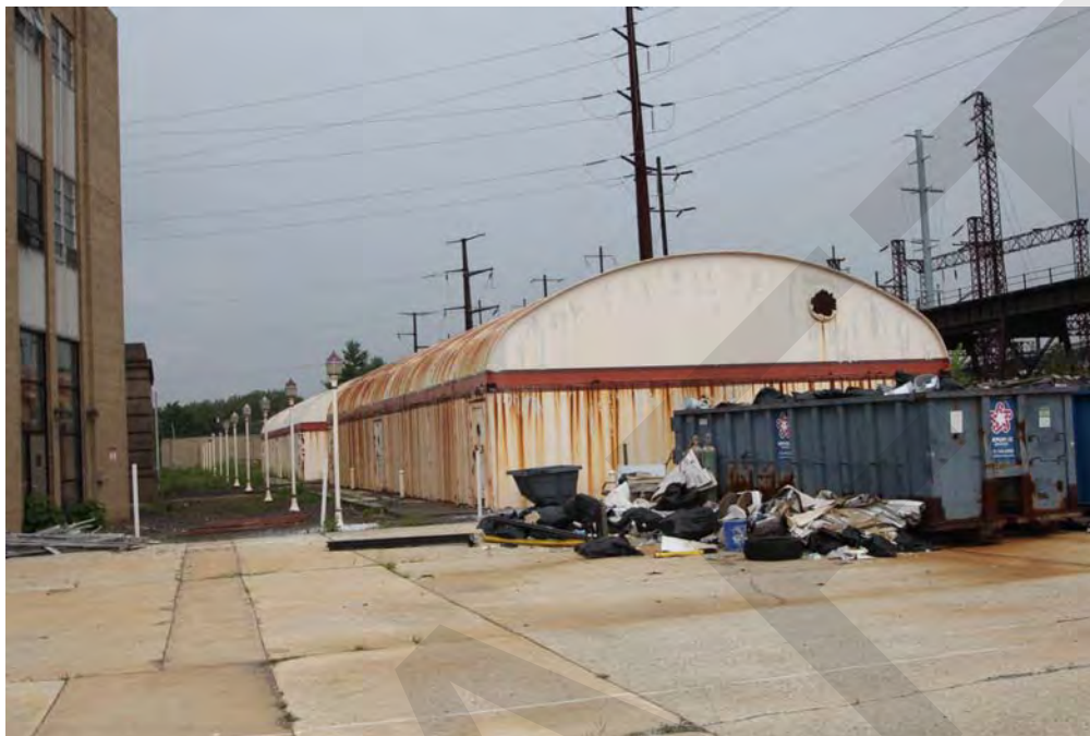
Photo 31 - Converter Unit #4, looking northwest.
