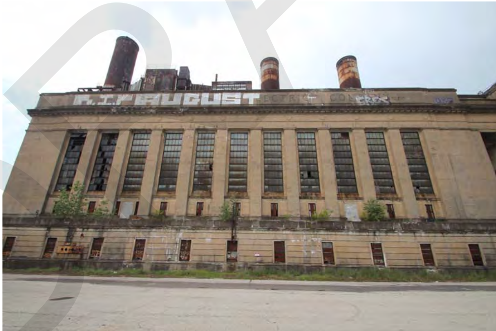
Photo 3 - Boiler House, north elevation, looking south.
