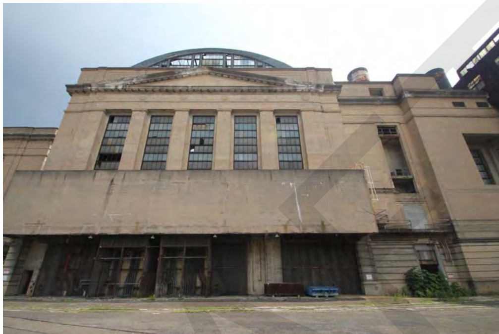
Photo 6 - Turbine Hall, south elevation, looking north.
