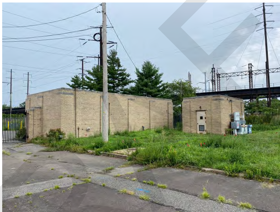
Photo 34 – Garage and Sewage Pumphouse, south and east elevations, looking northwest.
