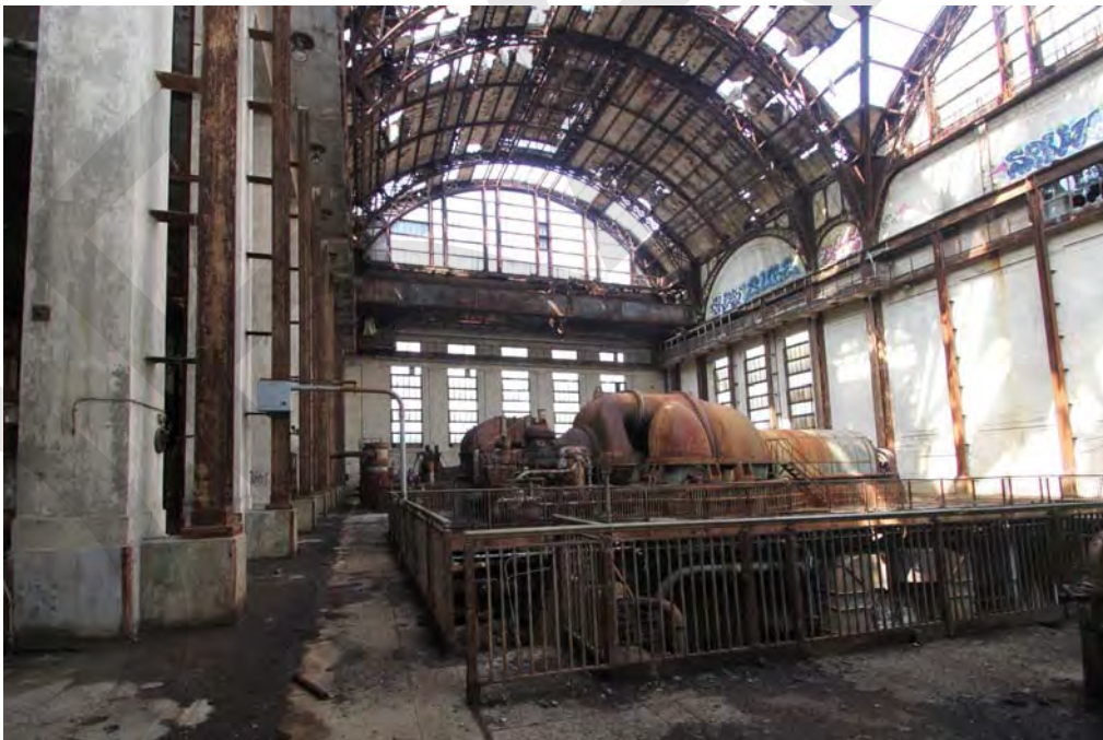
Photo 17 - Turbine Hall, main floor, looking northeast.
