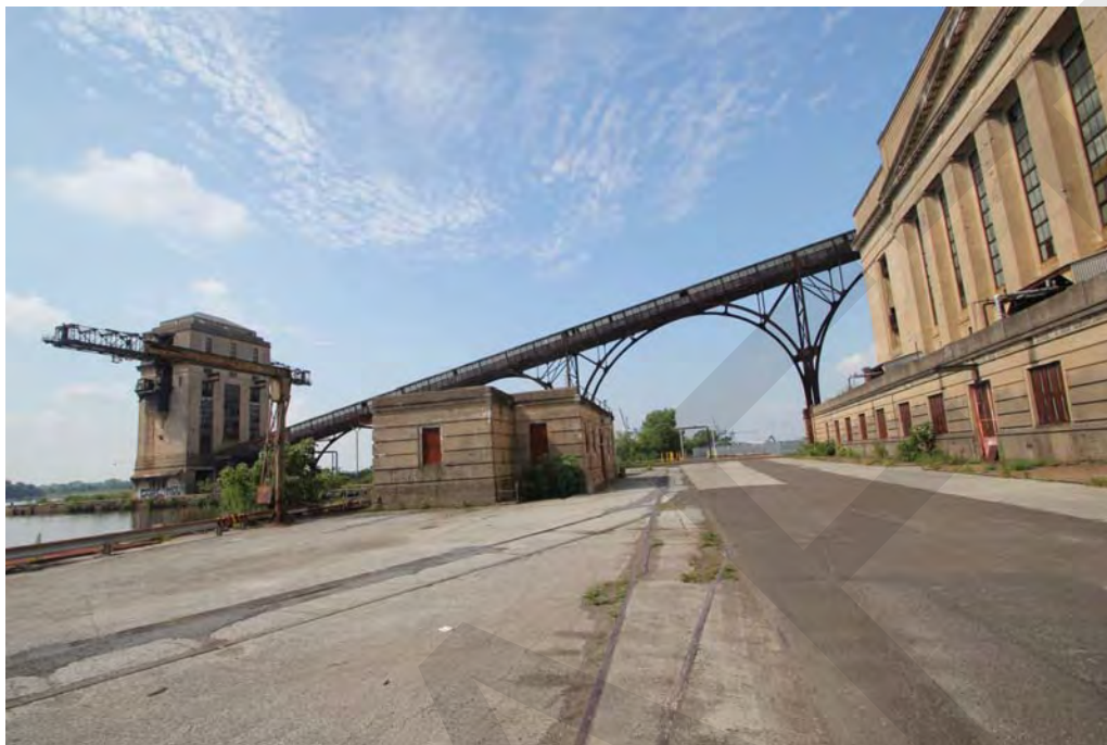
Photo 27 - Coal Conveyor, looking south.
