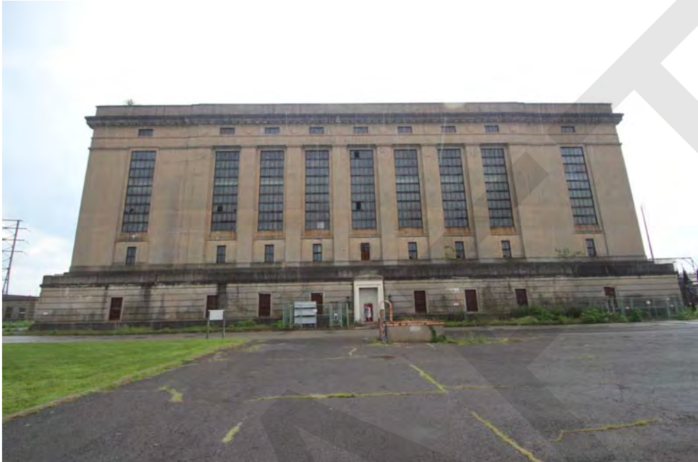
Photo 7 - Switch House, west elevation, looking east.
