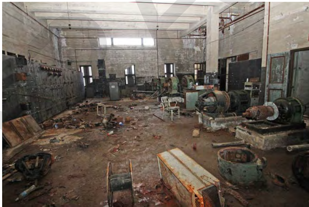
Photo 24 - Switch House, second floor, looking north.
