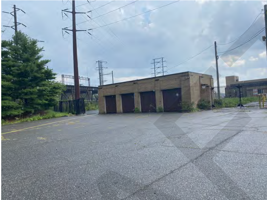
Photo 33 - Garage, west and south elevations, looking southeast.
