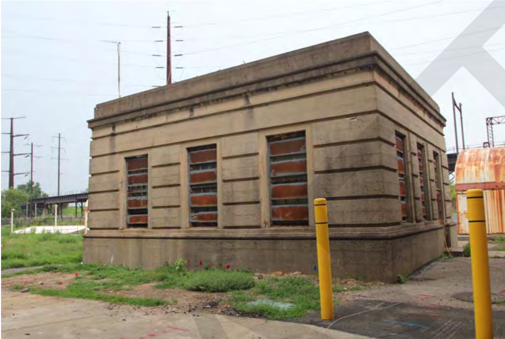
Photo 29 - Control House, south and east elevations, looking northwest.
