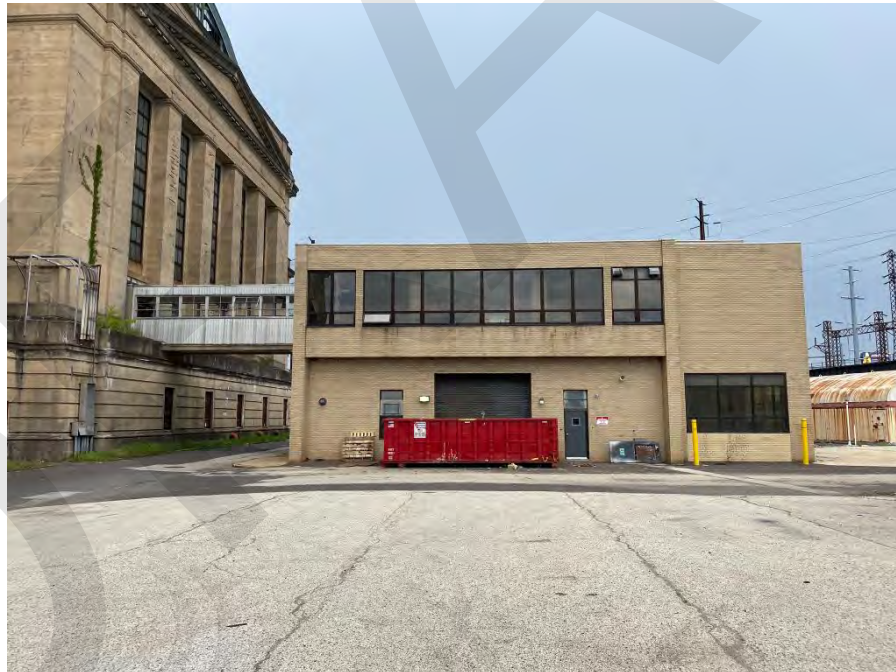
Photo 36 - Utility Building, east elevation, looking west.
