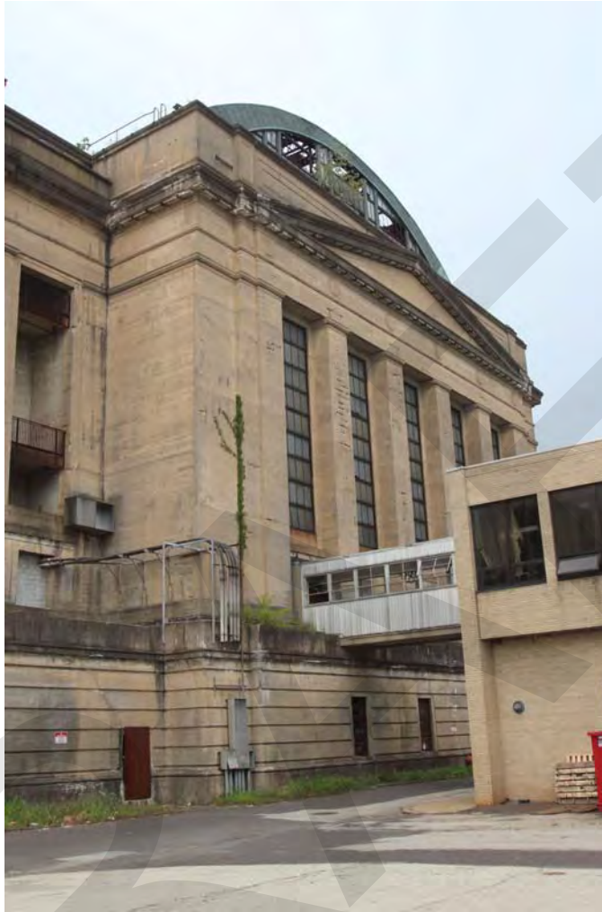
Photo 5 - Turbine Hall, north elevation, looking southwest.
