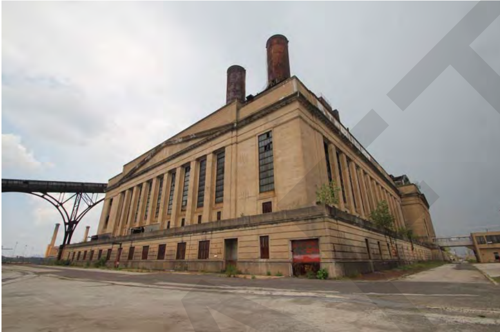
Photo 2 - Boiler House, east and north elevations, looking southwest.
