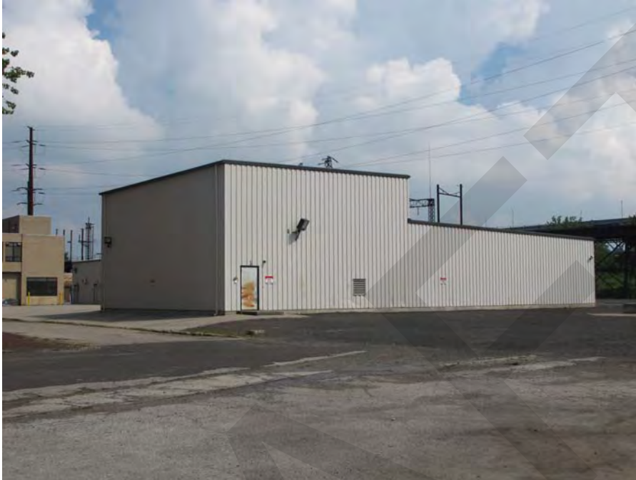
Photo 38 - Storage Building, south and east elevations, looking northwest.
