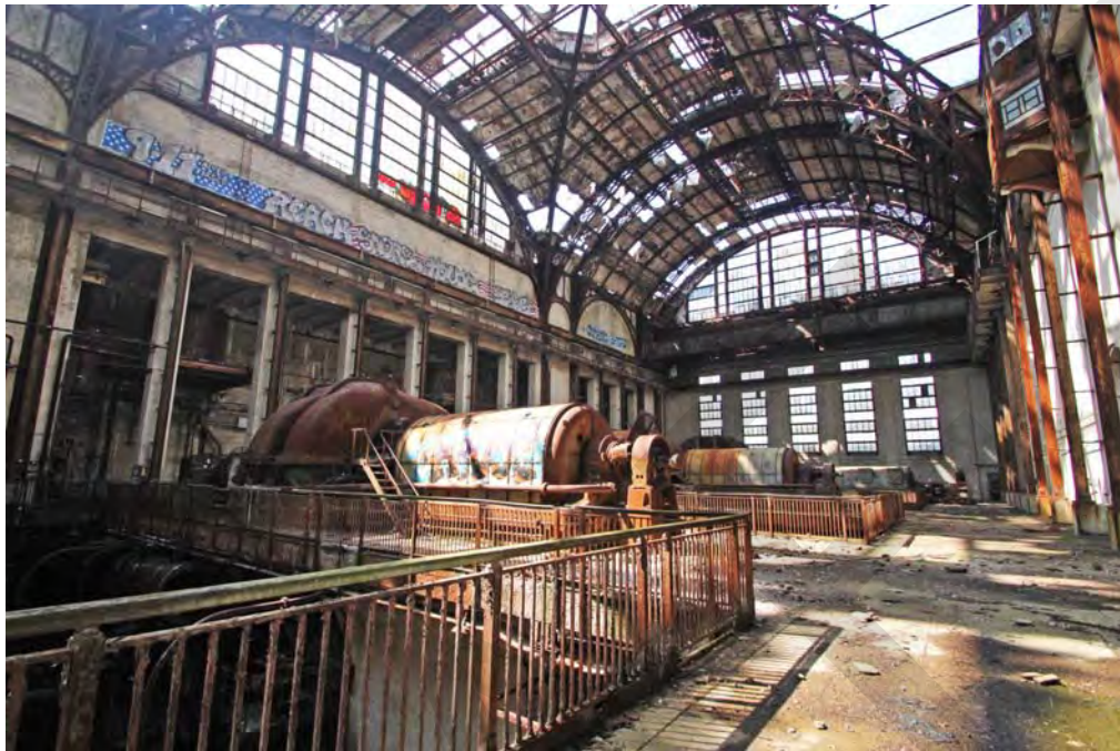
Photo 16 - Turbine Hall, main floor, looking southeast.
