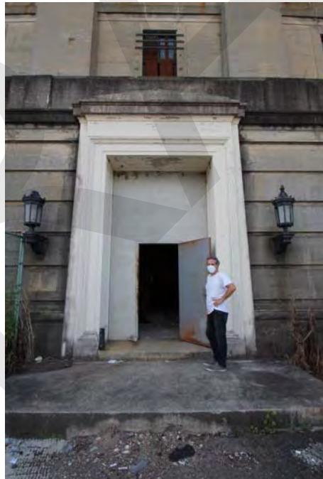
Photo 10 - Switch House, main entrance on west elevation, looking east.
