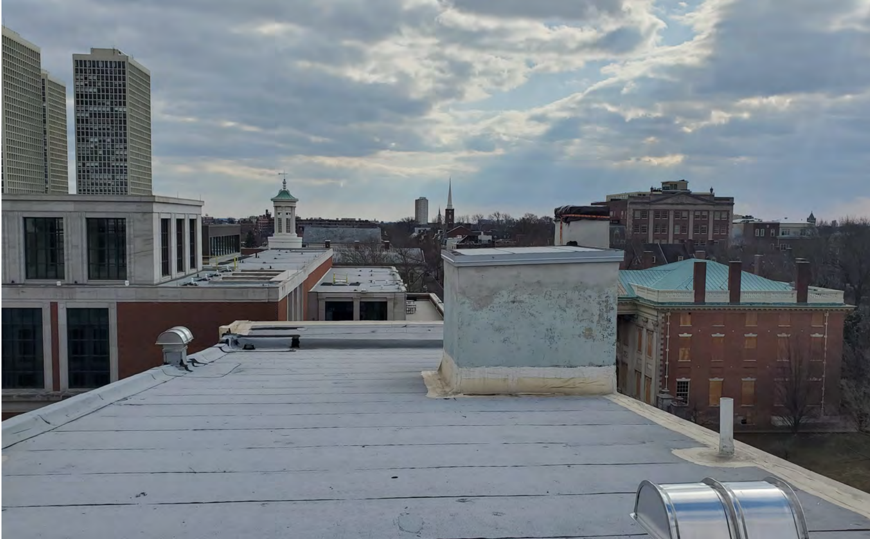
EXISTING VIEW SOUTH FROM UPPER ROOM OF 241 CHESTNUT STREET
