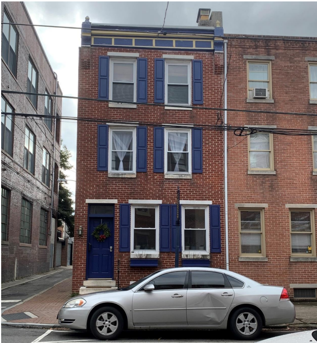
Figure 3. North (primary) façade of 1006 Bainbridge Street, January 2021.
