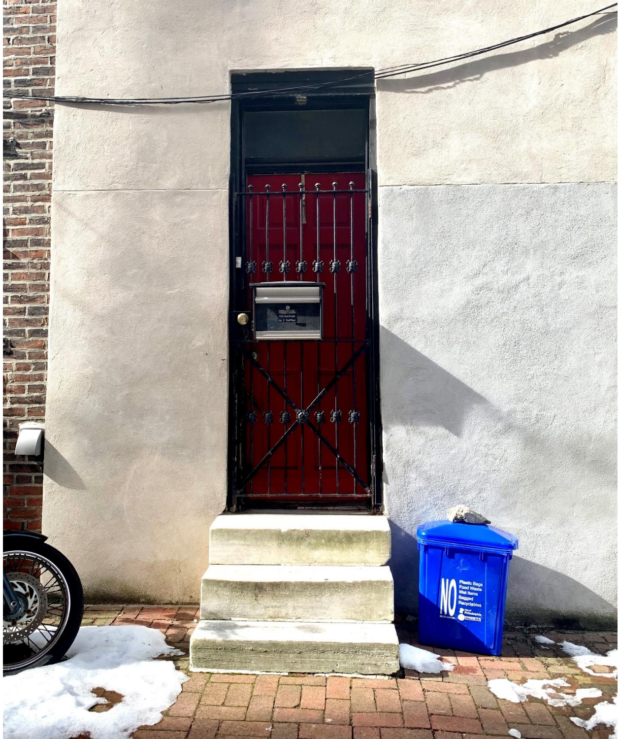
Figure 5. Side entrance with historic door frame and transom, February 2021.
