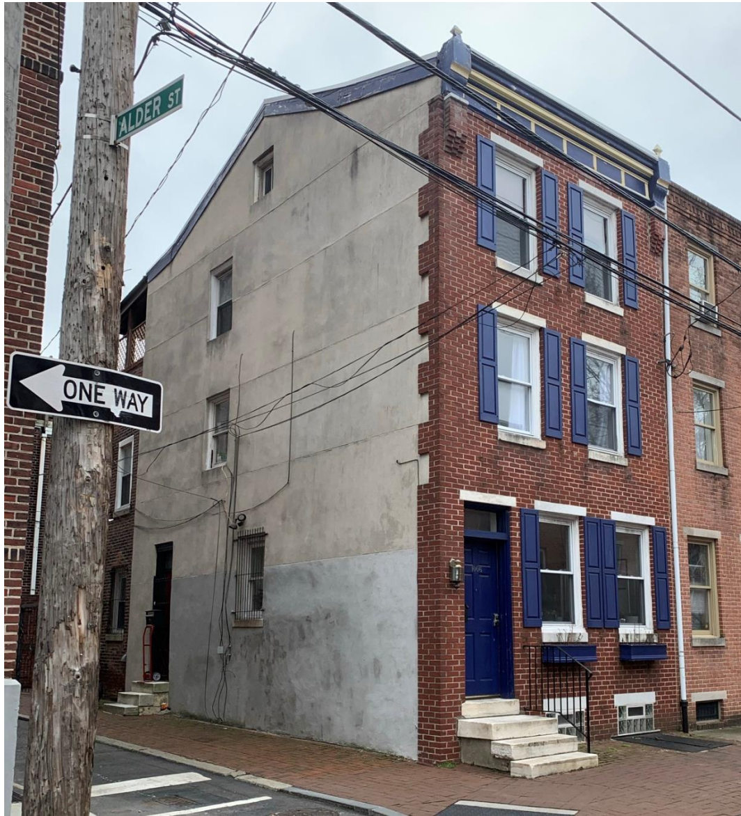
Figure 4. East (side) façade of 1006 Bainbridge Street, January 2021.
