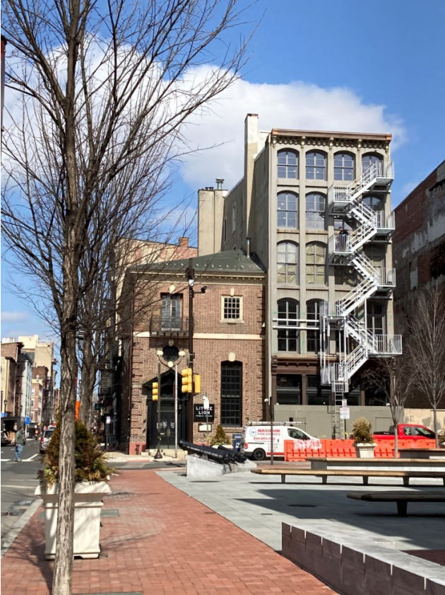
VIEW NORTH FROM 3RD ST
