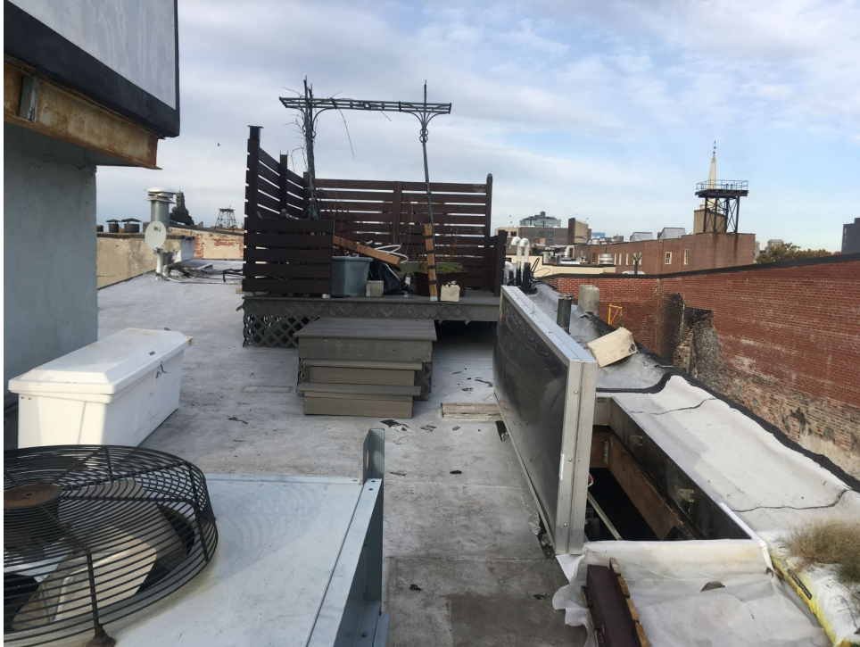
ORIGINAL ROOFTOP DECK & ACCESS HATCH, LOOKING NORTH (DATE: NOVEMBER 8, 2018)
