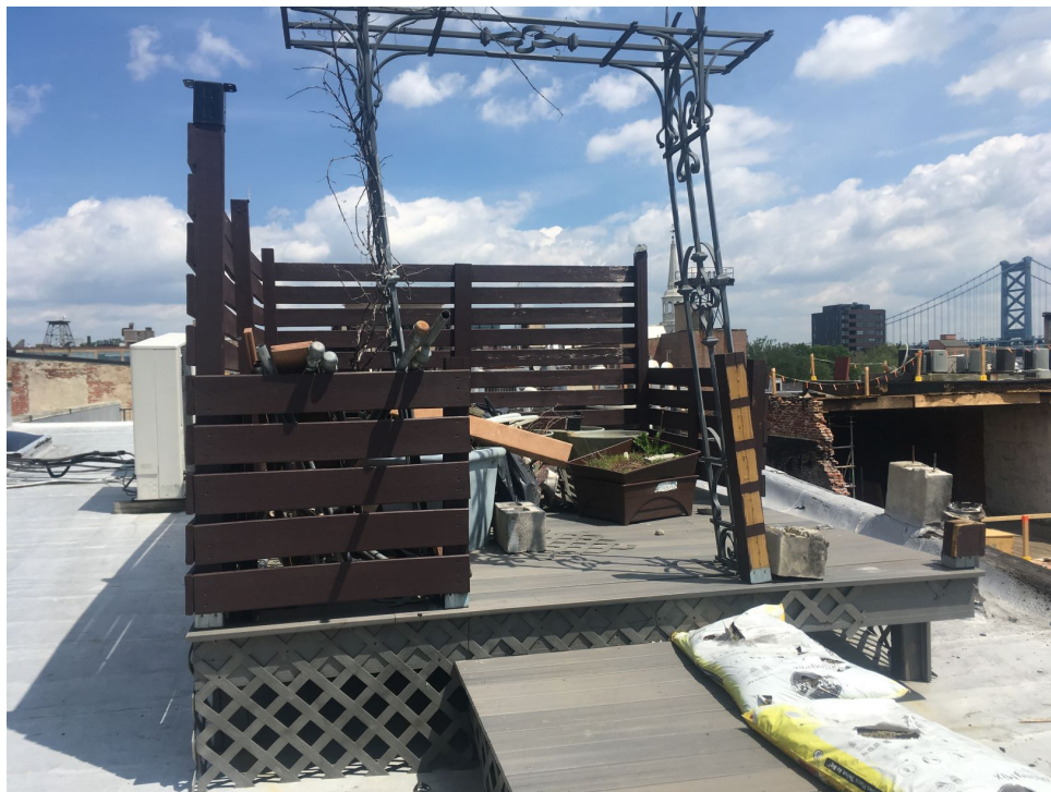
ORIGINAL ROOFTOP DECK, LOOKING NORTH (DATE: NOVEMBER 8, 2018)
