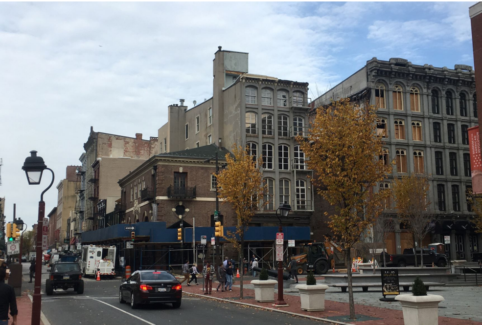
ORIGINAL ELEVATOR SHAFT WITH MACHINE ENCLOSURE SPACE, VIEW NORTH FROM 3 RD ST (DATE: NOVEMBER 8, 2018)
