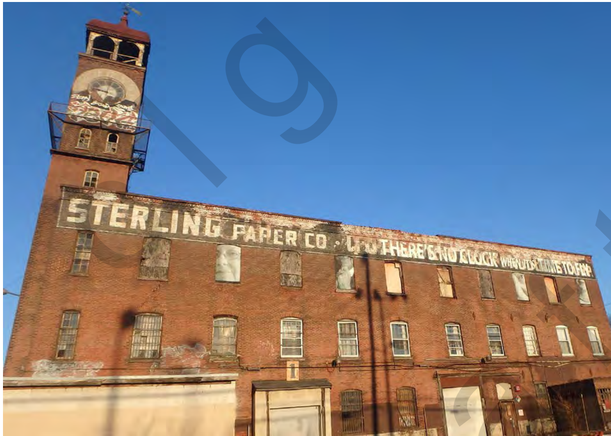
Photograph 1 – South elevations view northeast. 1881 and 1891 sections.
