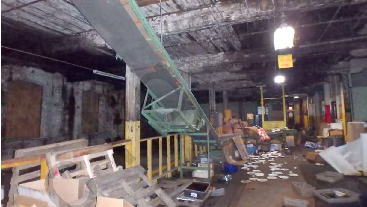
Photograph 6 – 1881 building, 1st floor, view north
