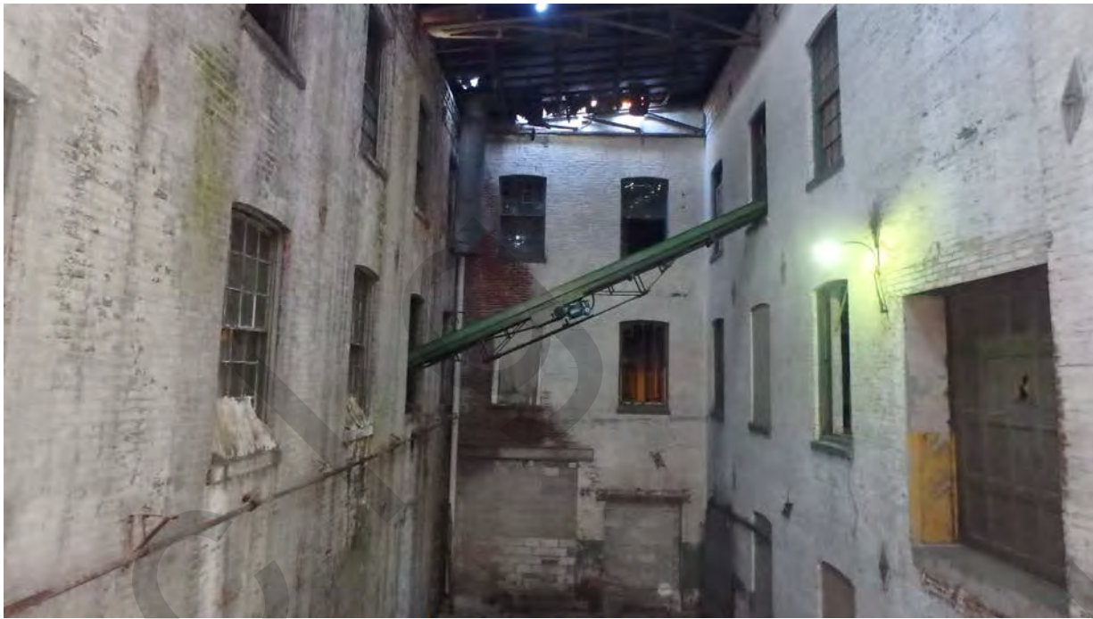
Photograph 14 – 1900 addition, 2nd floor, Courtyard, view north
