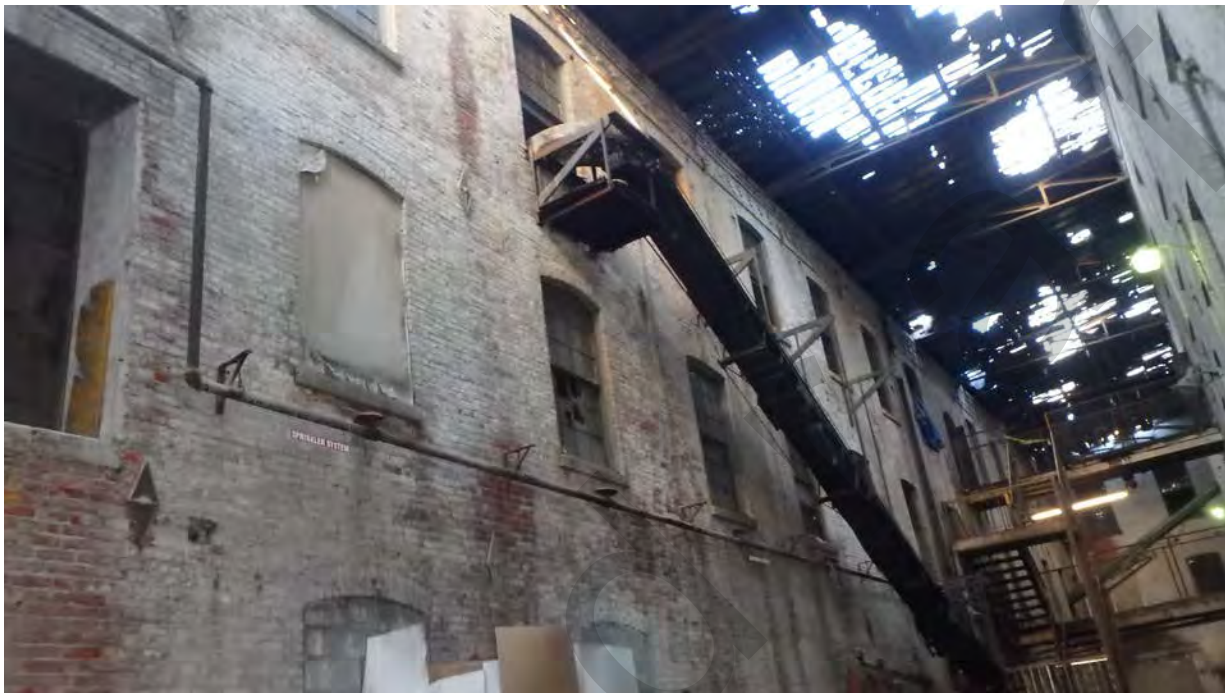
Photograph 9 – 1900 addition, Courtyard, 1st floor, view northeast
