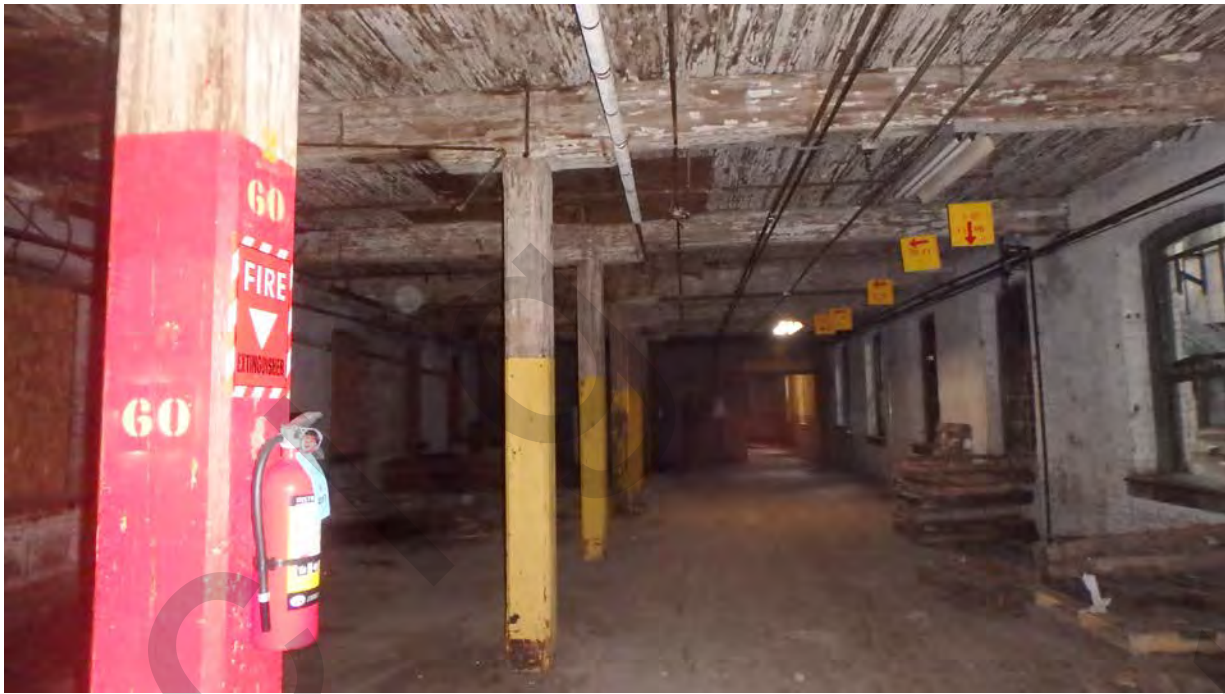
Photograph 8 – 1900 addition, 1st floor, view south
