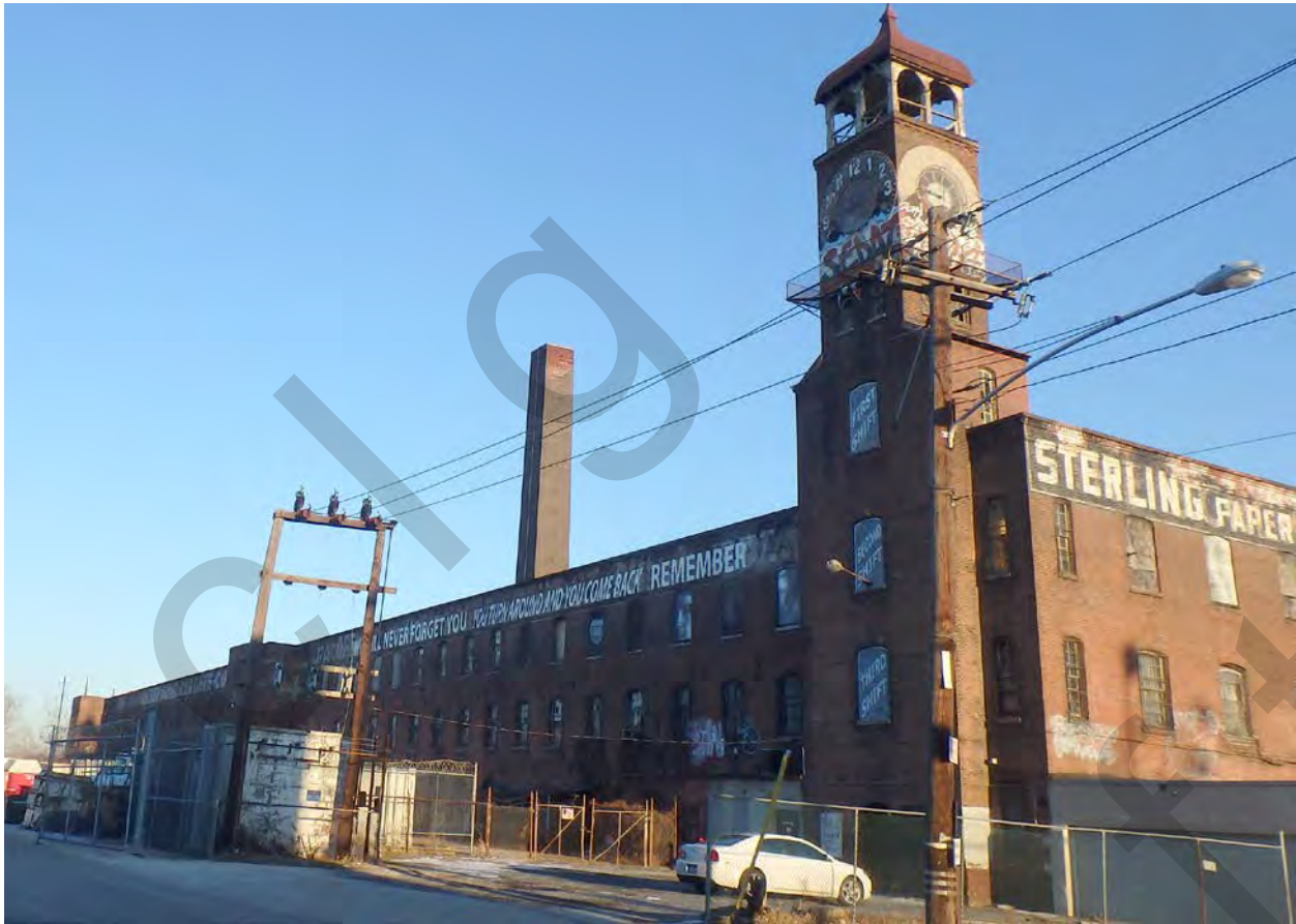
Photograph 2 – South and west elevations, view northeast. 1881 and 1900 sections.
