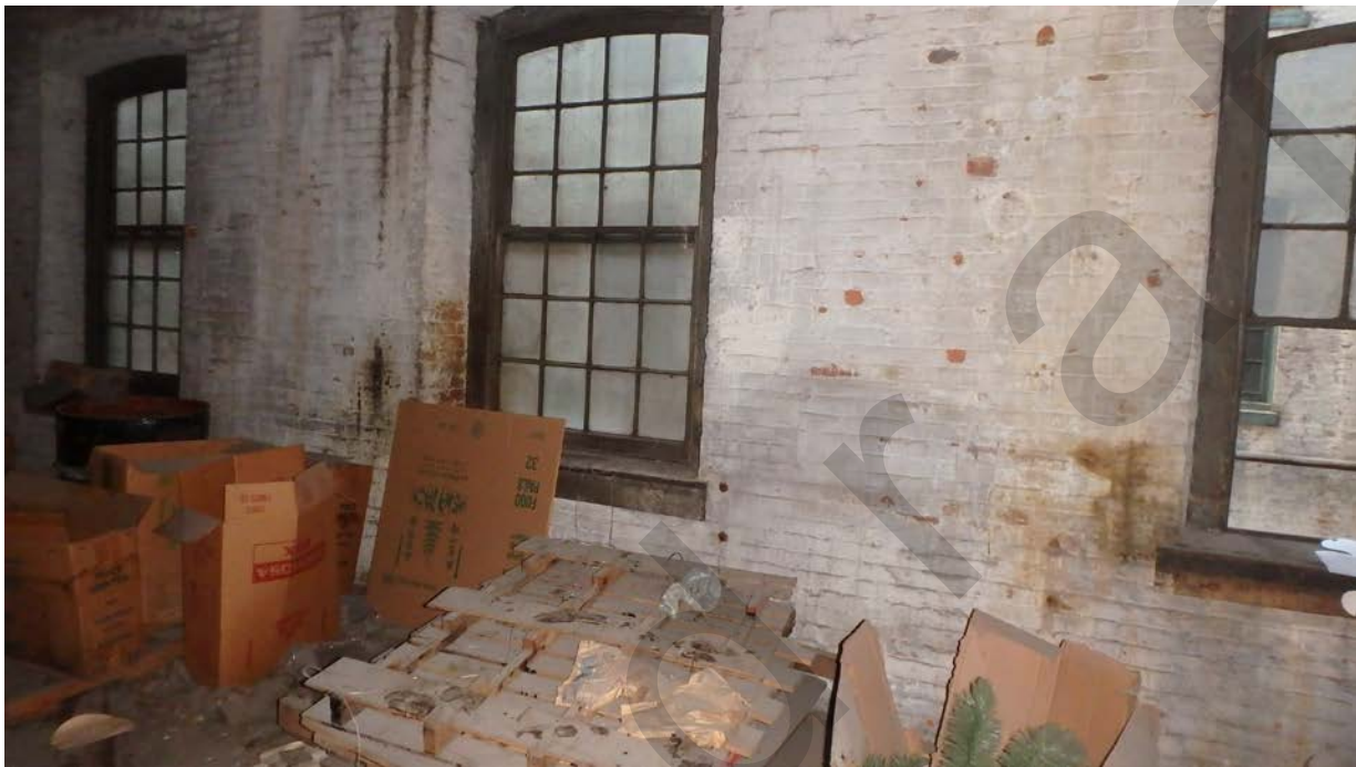
Photograph 11 – 1881 building, 2nd floor, view southwest
