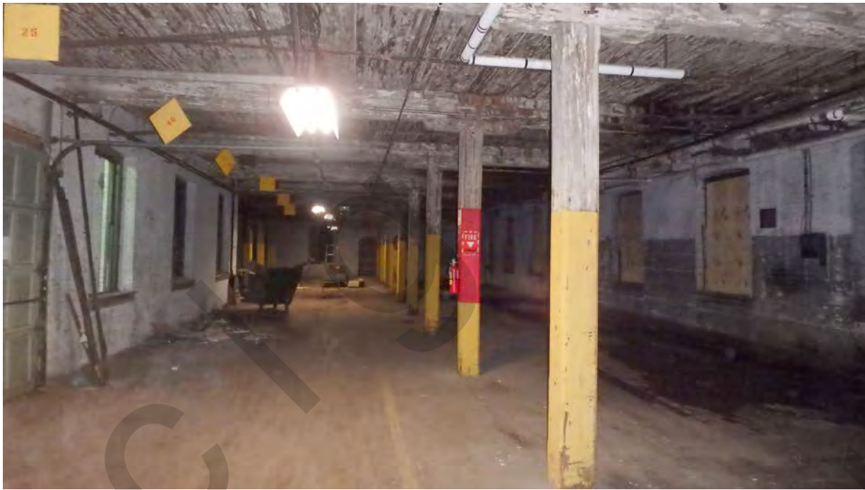
Photograph 10 – 1900 addition, 1st floor, view northeast
