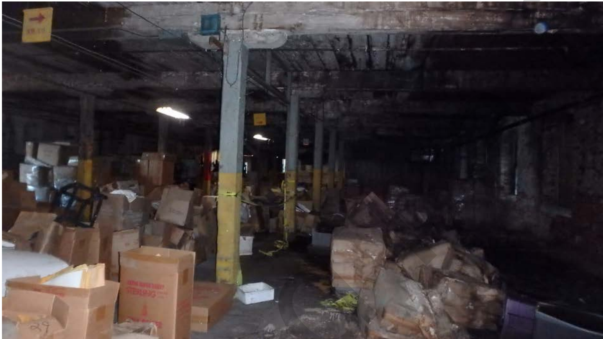
Photograph 13 – 1900 addition, 2nd floor, view north
