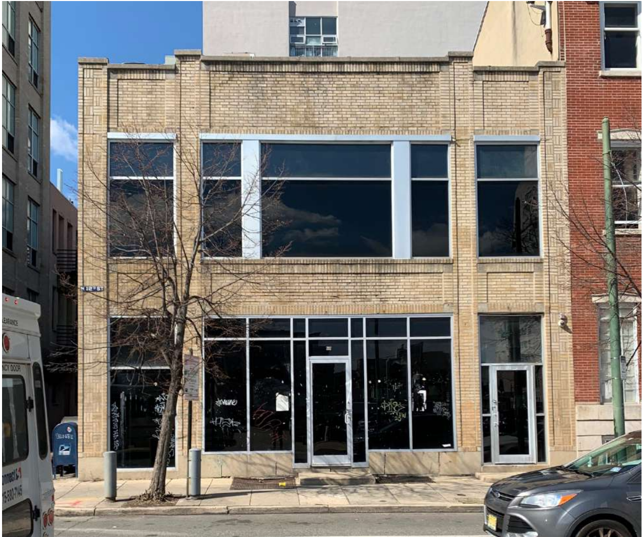
Figure 1: East (12 th Street) elevation of 210-212 N. 12 th Street.
